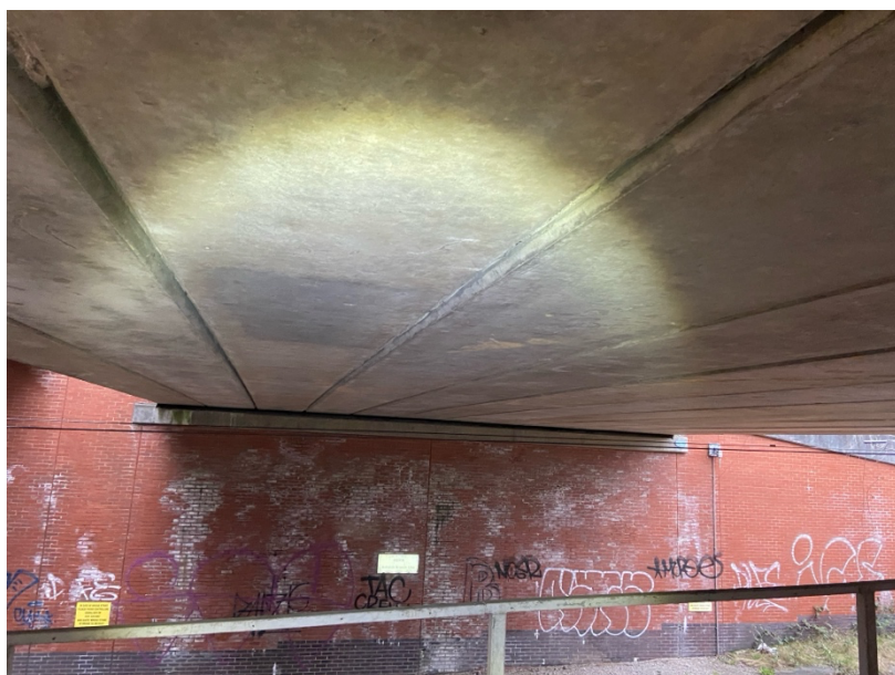
Figure 5 Rail Bridge North Side, Not Accessible
