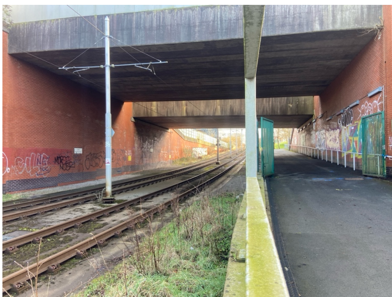
Figure 2 CWT_006 New Viaduct Street (Near) and Rail Bridge (Far)
