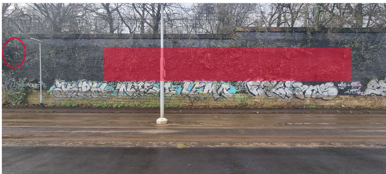
Figure 7 Location of CWT_002A Installation and bird nest
