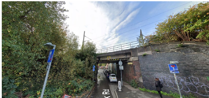
4. View through Cornbrook Metrolink Station Bridge (CDM 1/57)
