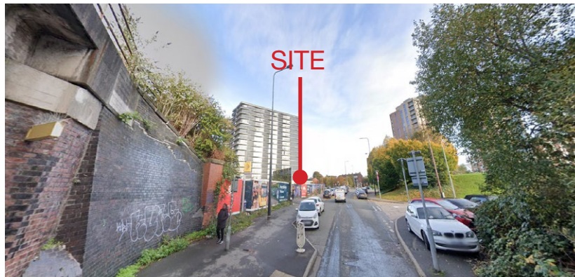
4. View of site from Cornbrook Metrolink Station Bridge (CDM 1/57)
