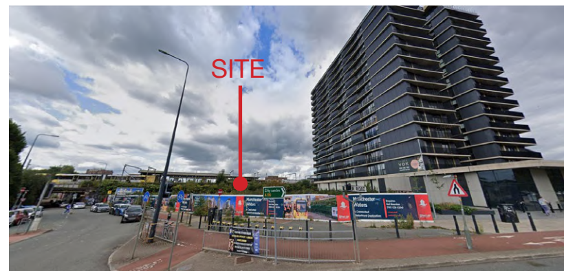
7. View of site from south corner outside site (A56)
