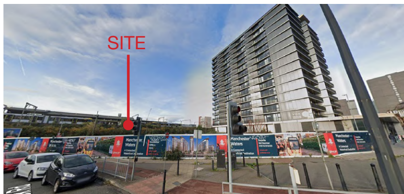
6. View of site from traffic lights/crossover on Cornbrook road
