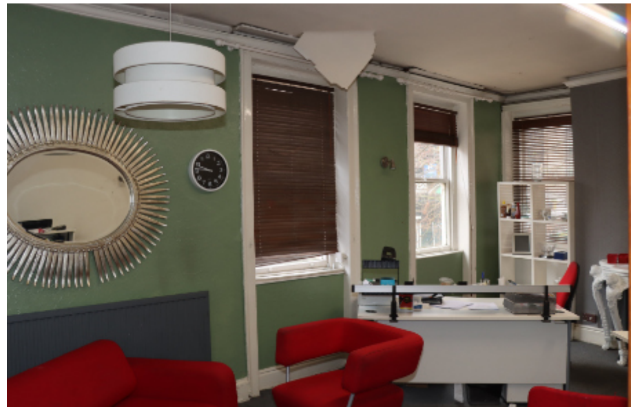
Photograph 24. The manager's office on the first floor above the pub.
