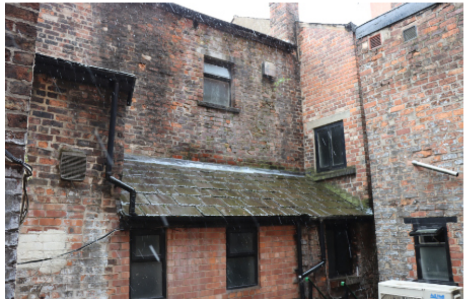
Photograph 16. A view from the flat roof at first floor level.
