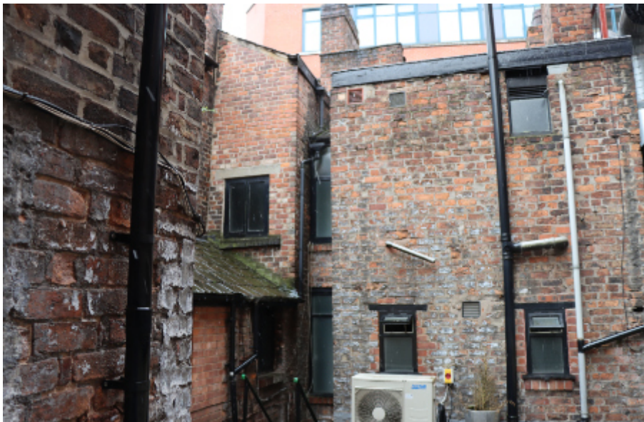
Photograph 15. A view from the flat roof at first floor level.
