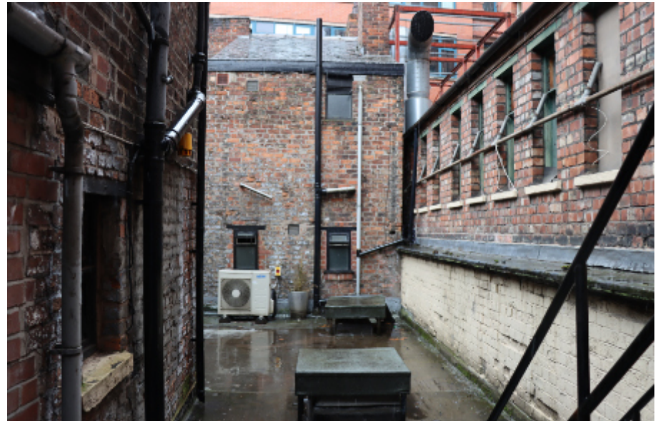
Photograph 14. Looking towards the rear from a first floor window.
