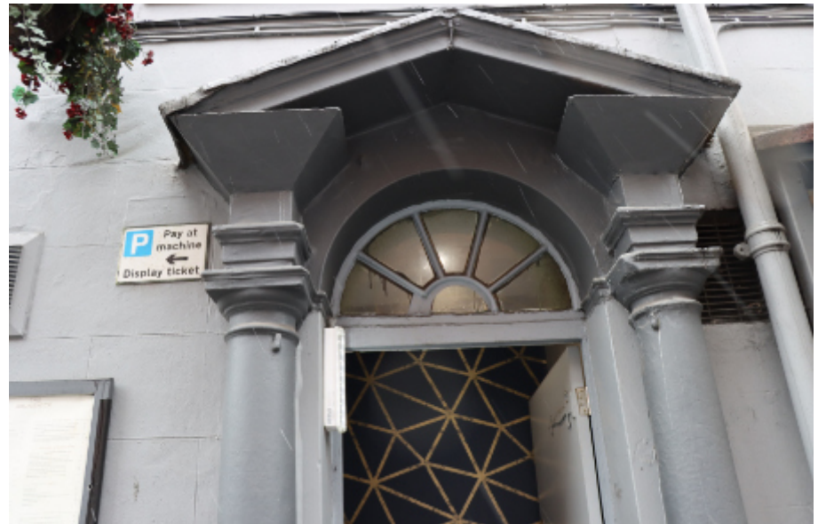
Photograph 12. The middle doorcase on the Paton Street elevation.
