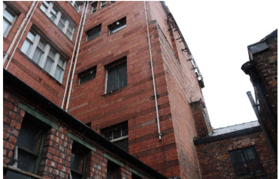
Photograph 18. A view from the flat roof at first floor level.
