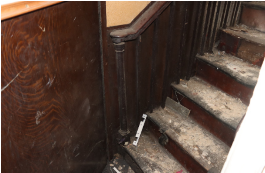
Photograph 25. The staircase from the first to the second floor in the front part of the building.
