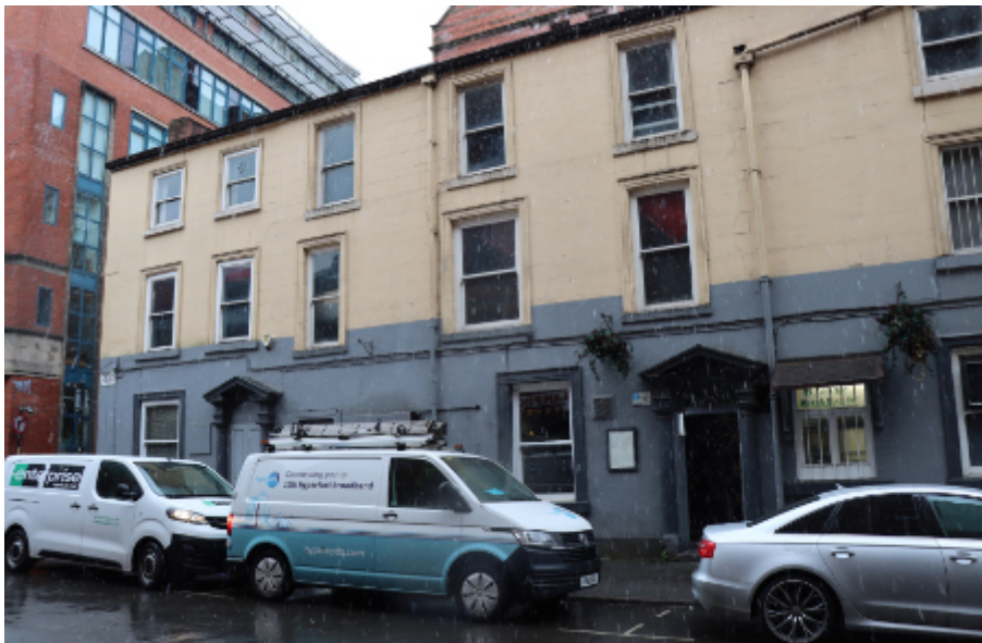
Photograph 7. The Paton Street elevation.
