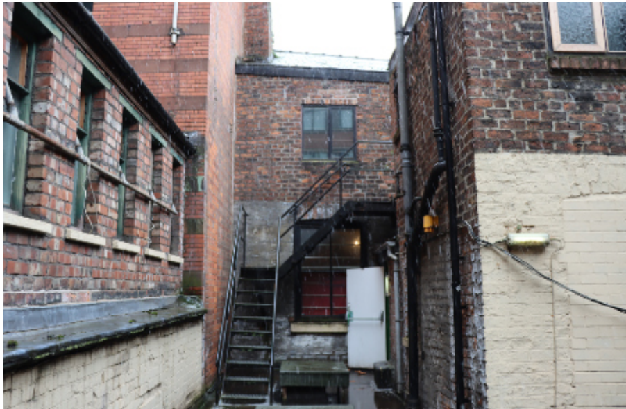
Photograph 17. A view from the flat roof at first floor level.
