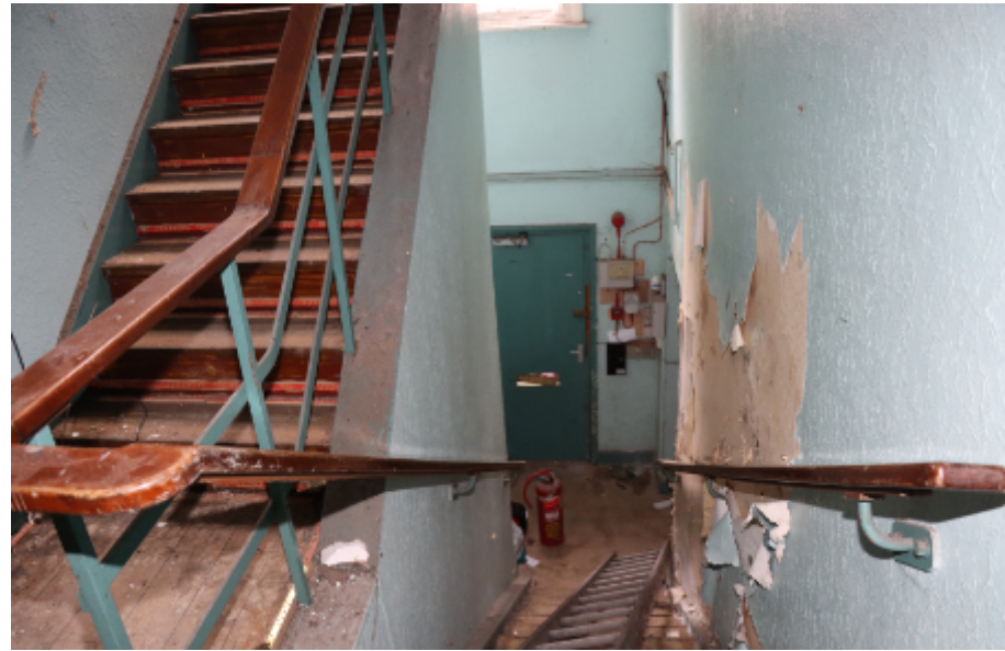
Photograph 34. The staircase from the ground to the first floor in the rear part of the building.
