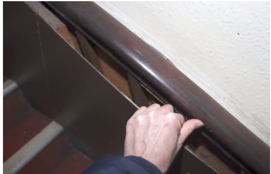
Photograph 22. The balustrade to the staircase that leads from behind the bar in the pub to the first floor.
