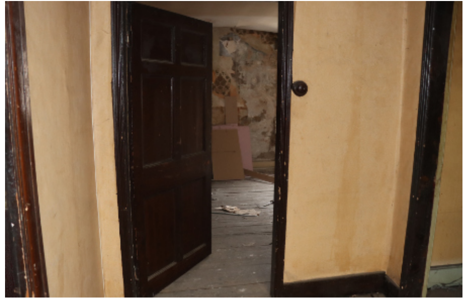
Photograph 30. A 6-panel door on the second floor.
