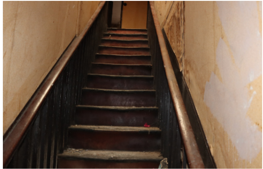
Photograph 26. The staircase from the first to the second floor in the front part of the building.
