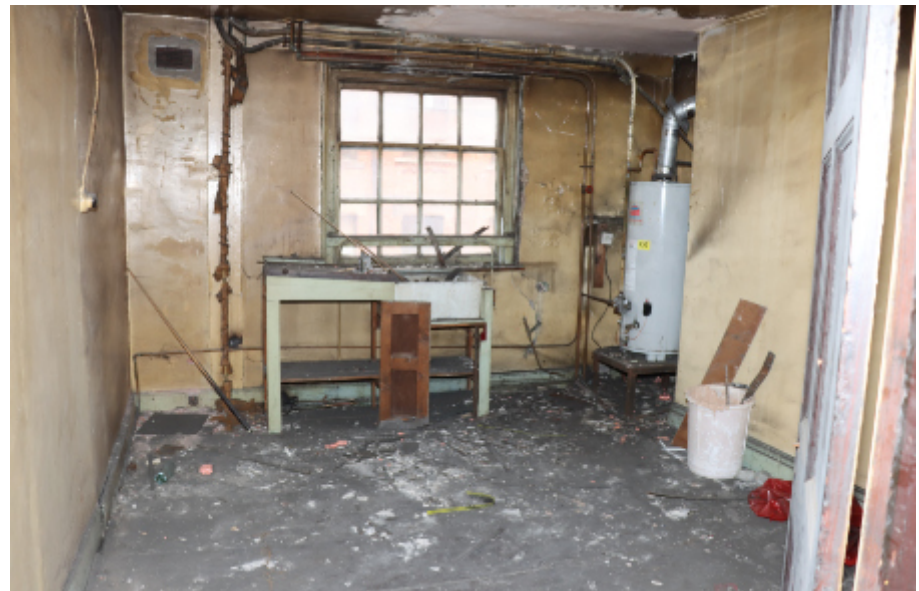
Photograph 28. A second floor room, with a 4 over 8 sash window on the Paton Street elevation.
