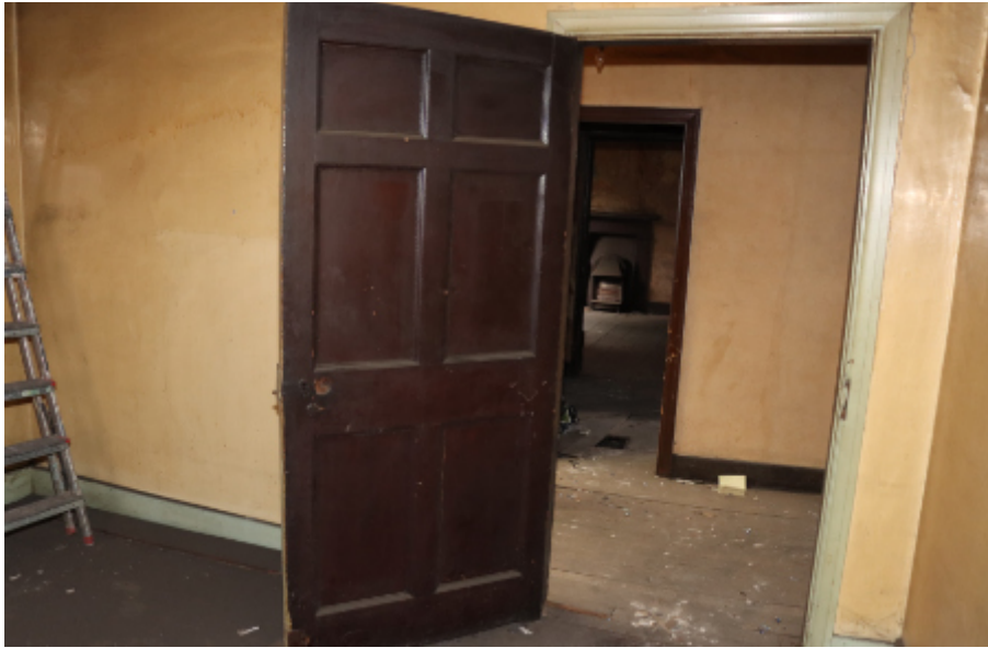
Photograph 29. A 6-panel door on the second floor.
