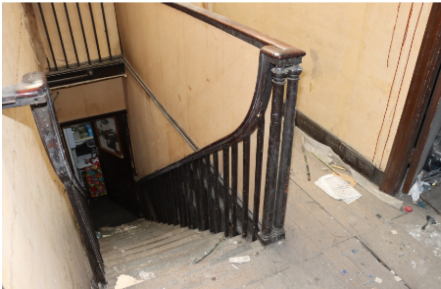
Photograph 27. The staircase from the first to the second floor in the front part of the building.
