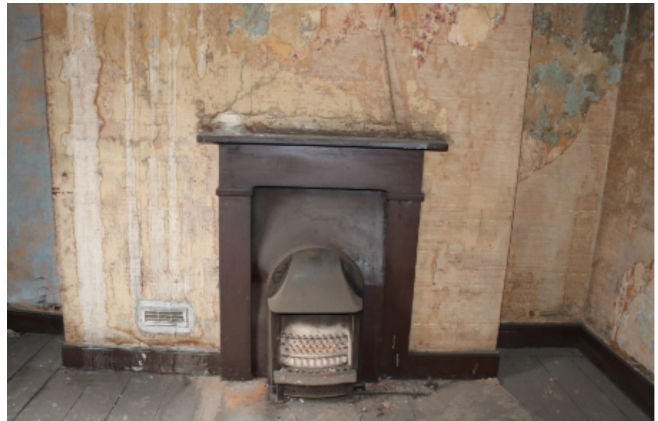
Photograph 32. A fireplace in the southern second-floor rear room.
