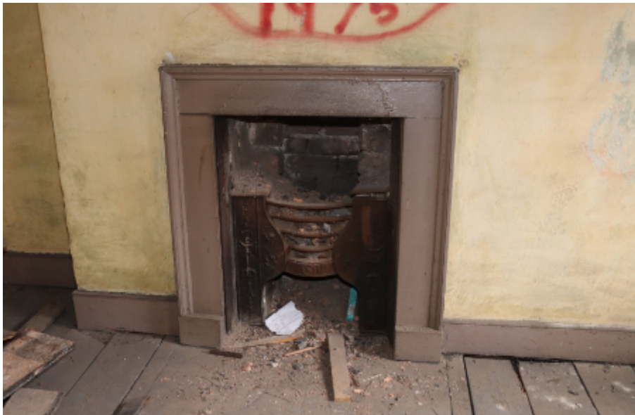
Photograph 31. A fireplace with a hob grate, in the southern second-floor room on the Piccadilly elevation.
