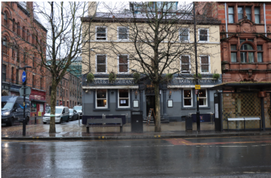
Photograph 3. The front of the building.
