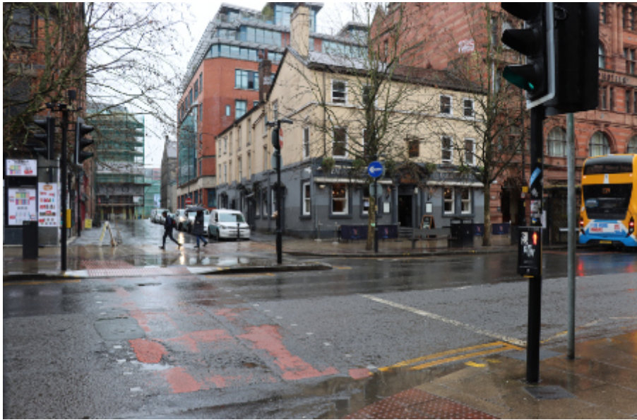
Photograph 5. Paton Street, viewed from Piccadilly.
