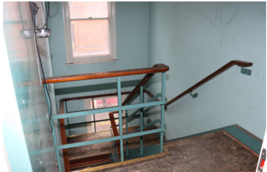
Photograph 40. Looking down from the second floor staircase landing in the rear part of the building.
