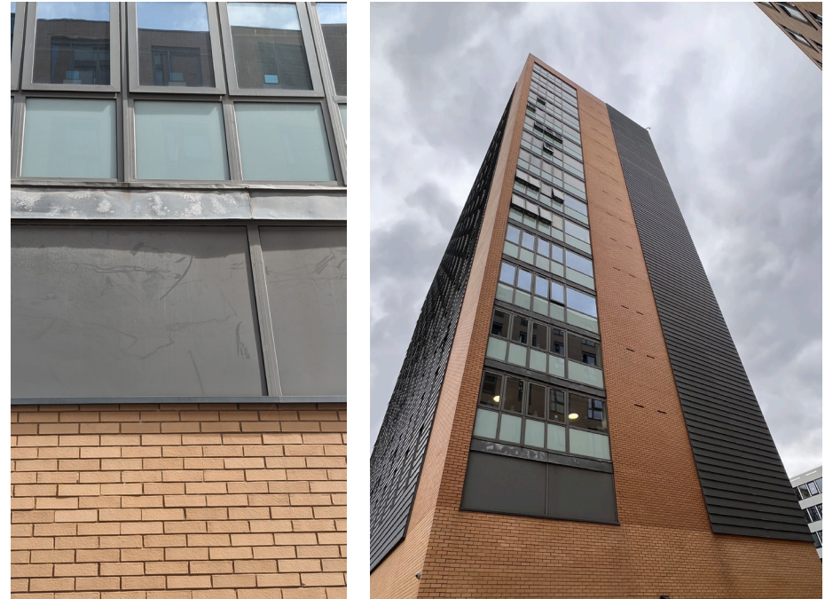
Figure 4 & 5 - Existing condition of the brick and zinc facade
