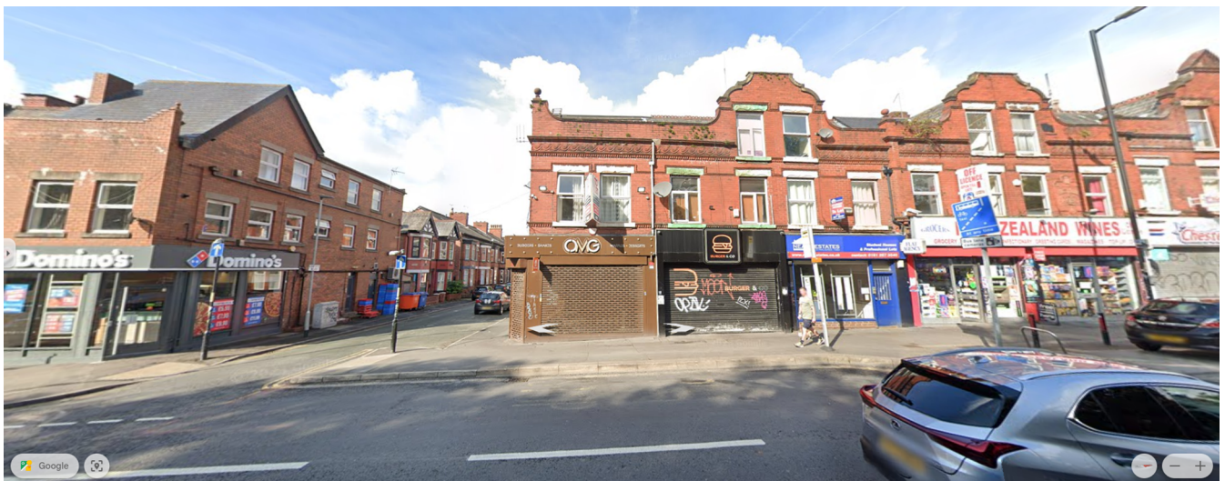
Figure 3. Wilmslow Road frontage.
