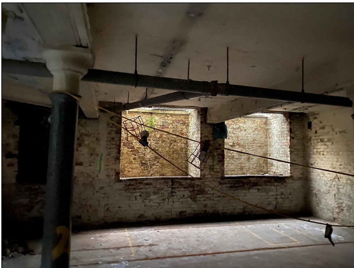
Plate 13 – Internal character of the cellar
