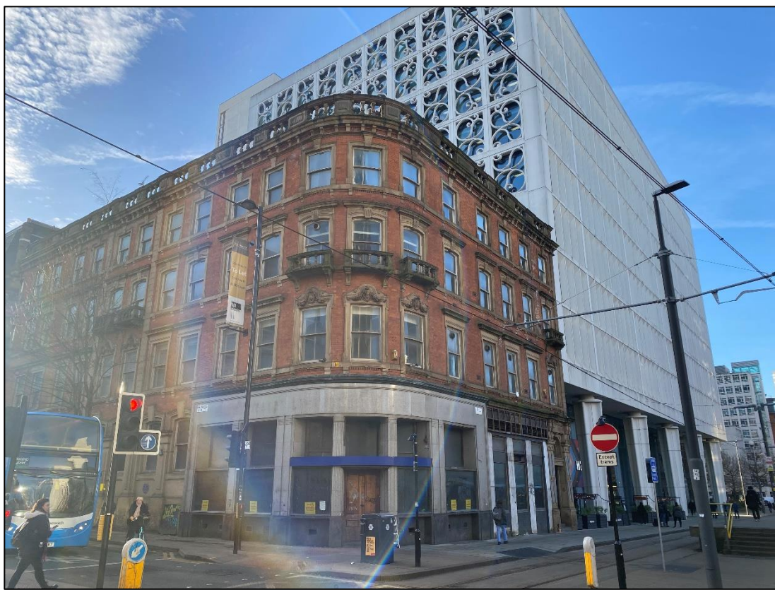
Plate 1 – 77-79 Mosley Street as seen from the north
