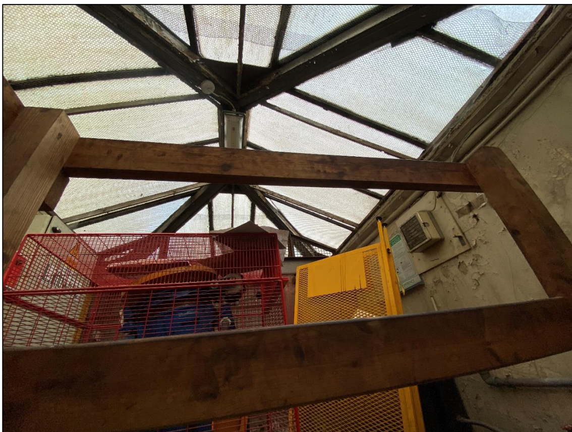
Plate 11 – Internal character of hipped section of the roof
