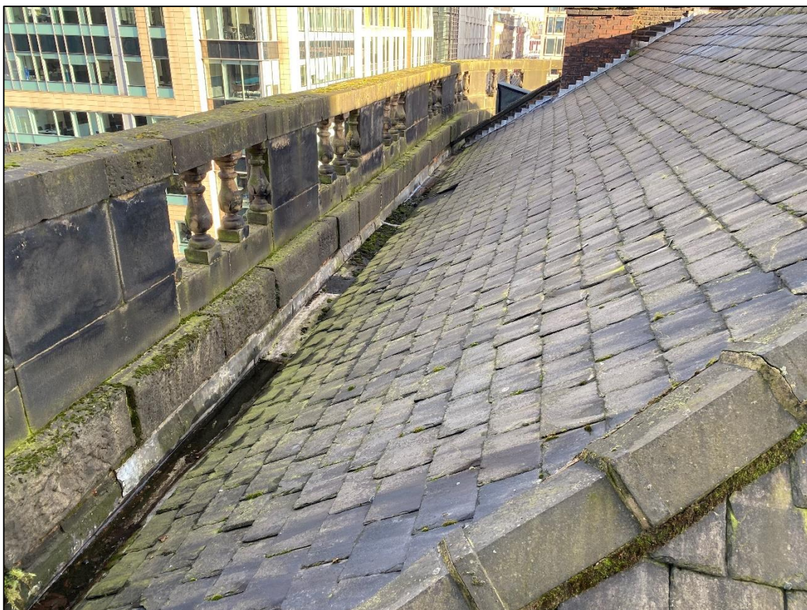
Plate 9 – Another portion of the roof accessed, with further lifted slates
