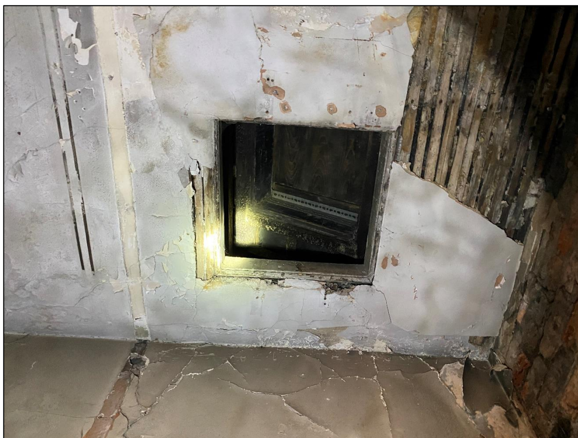
Plate 6 – Loft hatch providing access to the roof
