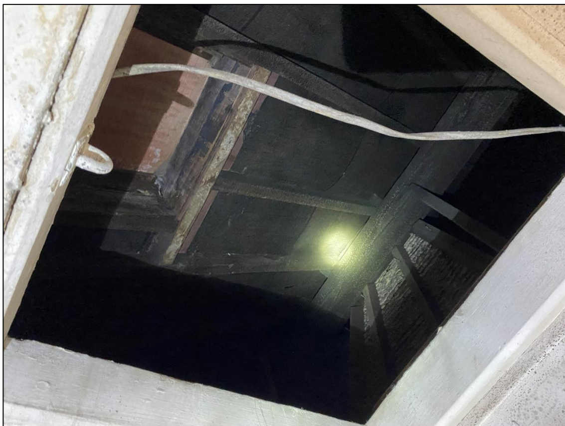
Plate 3 – Bitumen roof lining present in areas of loft
