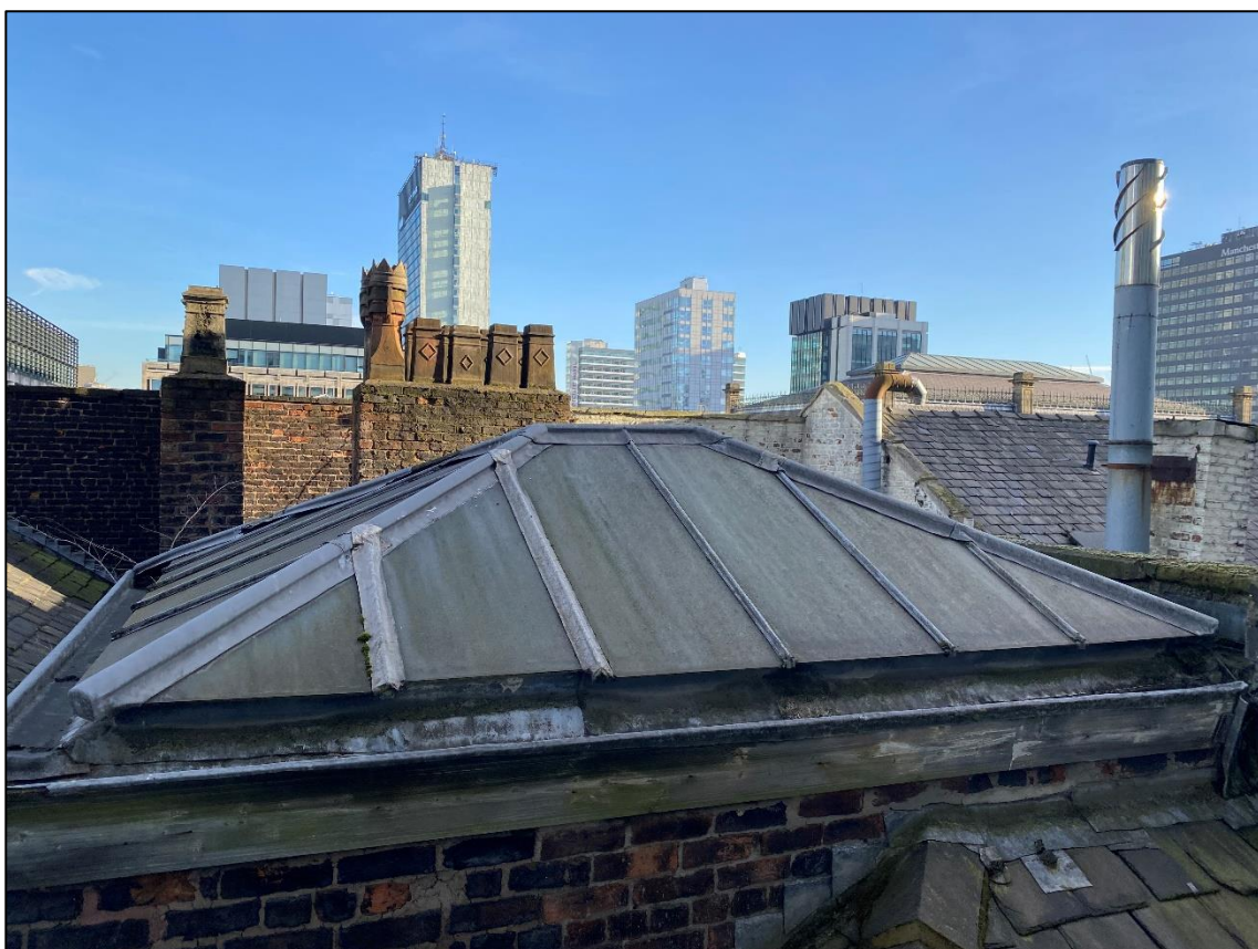
Plate 10 – Glazed, hipped section of roofing
