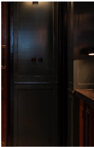
WF-01 / WF-06 MDF HAND PAINTED TIMBER RAILS ONTO EXISTING PLASTERBOARD. ALL TO BE PAINTED WITH GLOSS PAINT
