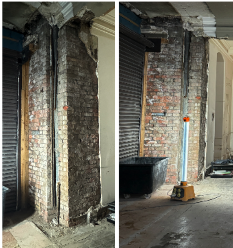
PHOTOGRAPHS SHOWING EXISTING WALL TREATMENT
