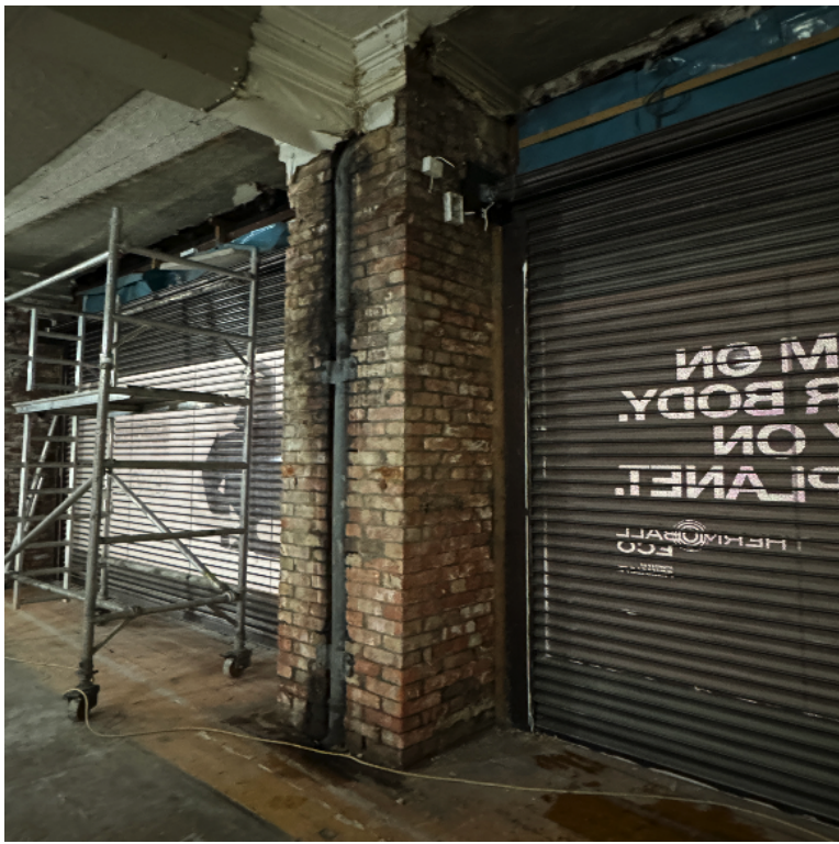
PHOTOGRAPH SHOWING EXISTING WALL TREATMENT
