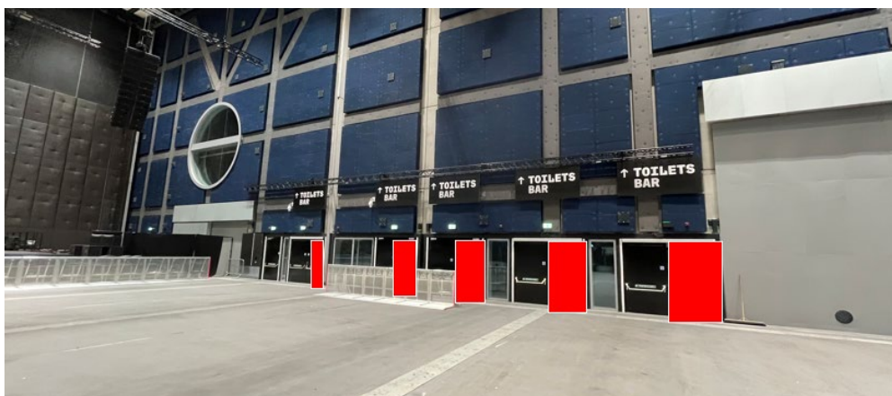
Figure 2: Doors in east wall Warehouse that were opened during one test (red)
