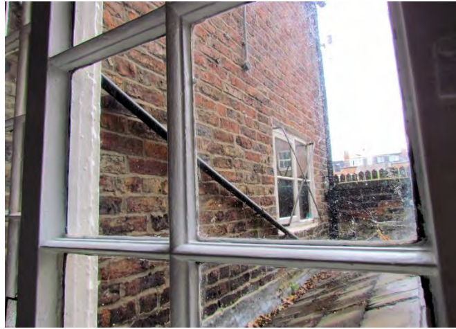
Window in North-West Range
