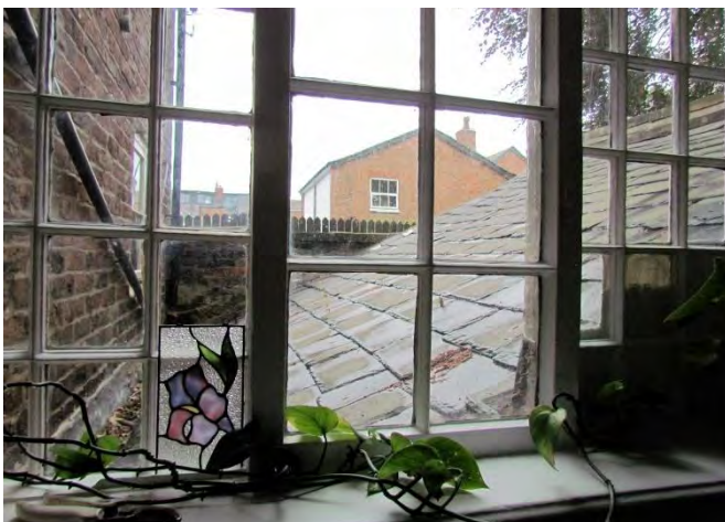
View of Roof Over Half Basement on North Side
