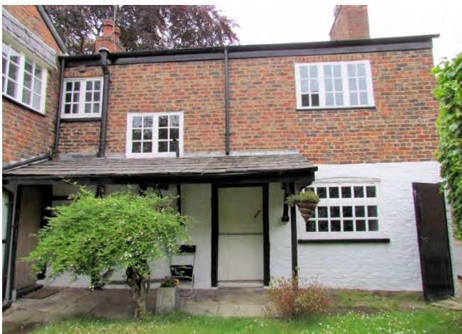
Rear Elevation, Main Range
