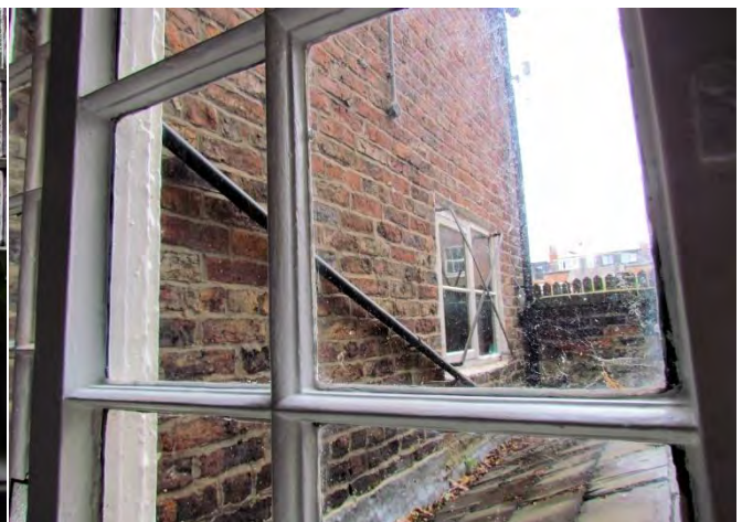
View Towards East Elevation of North-west Range
