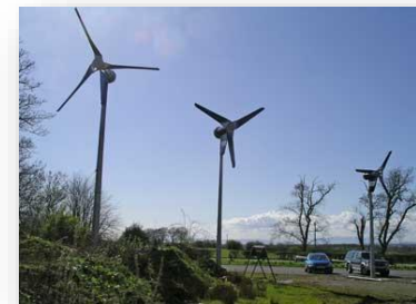
Wind Turbine Installation
