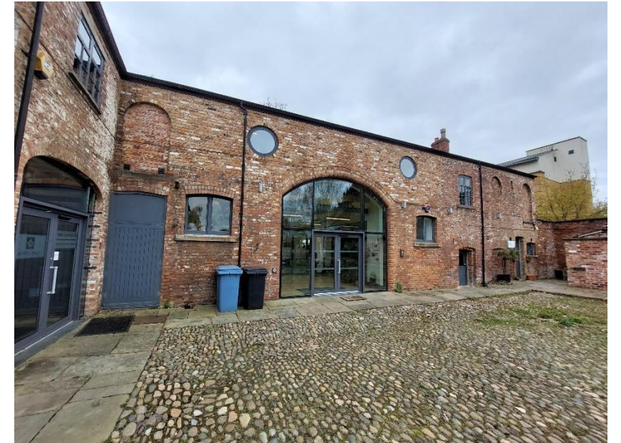
Courtyard External (East Elevation)
