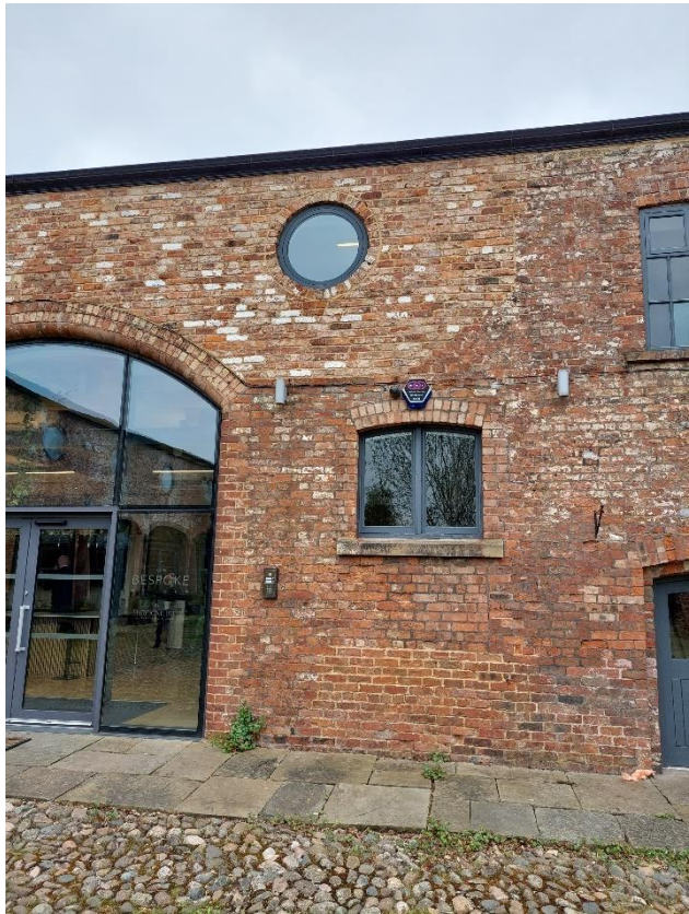
Courtyard External (East Elevation)
