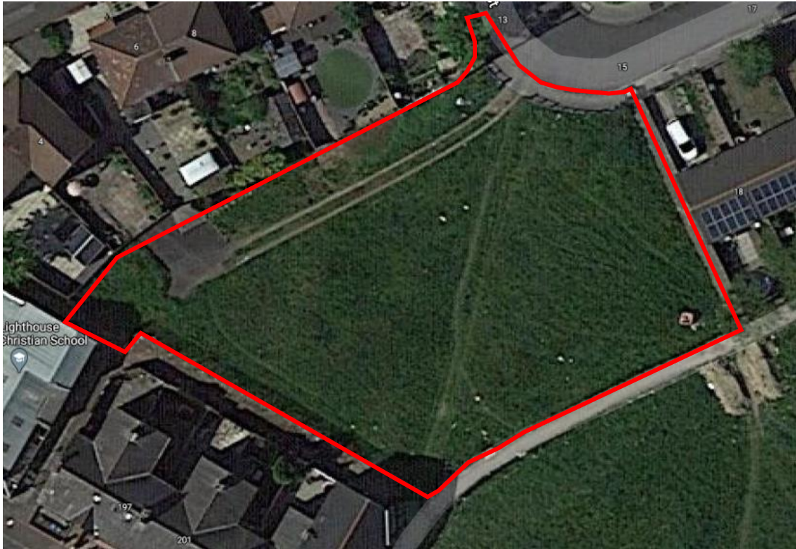
Figure 1.2 – Aerial view of existing Benton Street site
