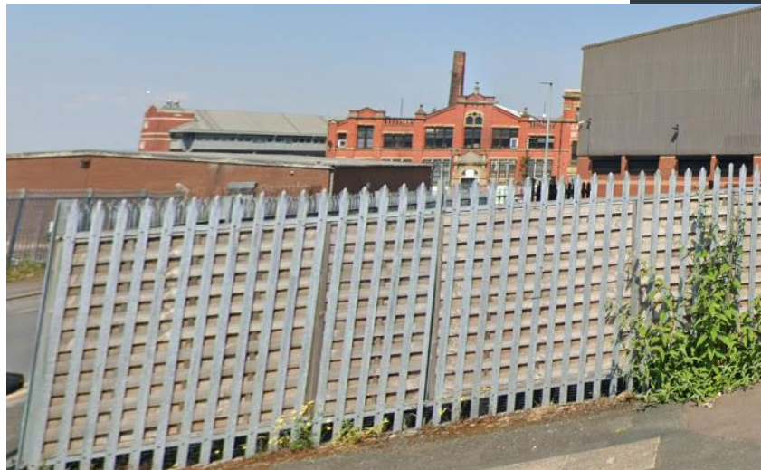
Insitu Palisade Fencing around the perimeter of the site.
