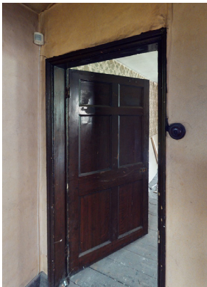
One of two 6-panel doors that have been identified as original.
