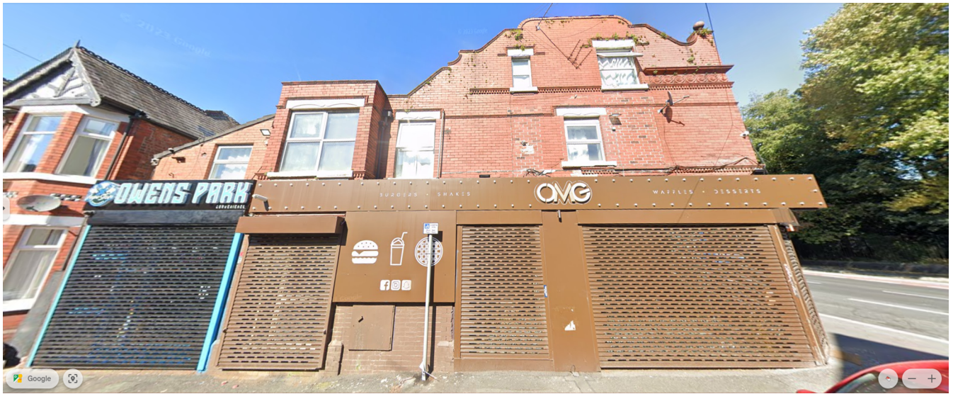
Figure 2. Cawdor Road frontage.
