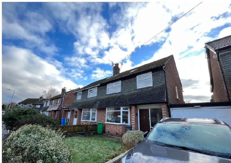
Figure 1. Main view of property.
