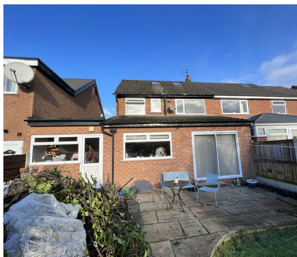
Figure 2. Rear view of property
