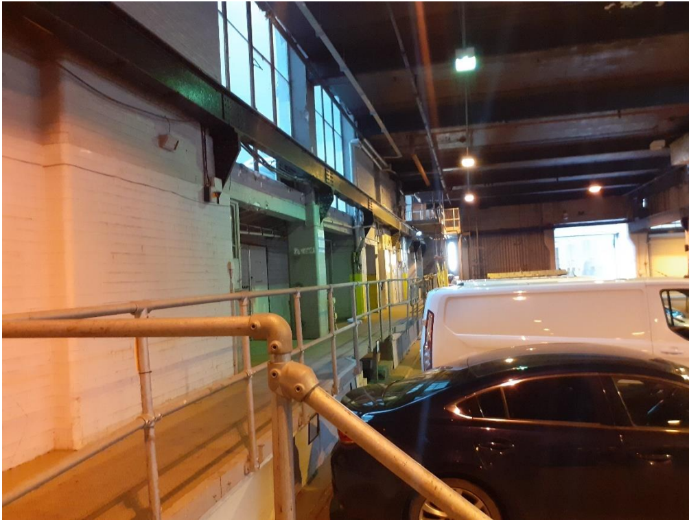
Plate 13: View along west elevation of undercroft wall looking north.
