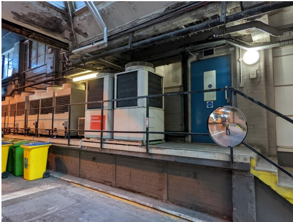
Plate 5: View of platform at the south end of the undercroft.
