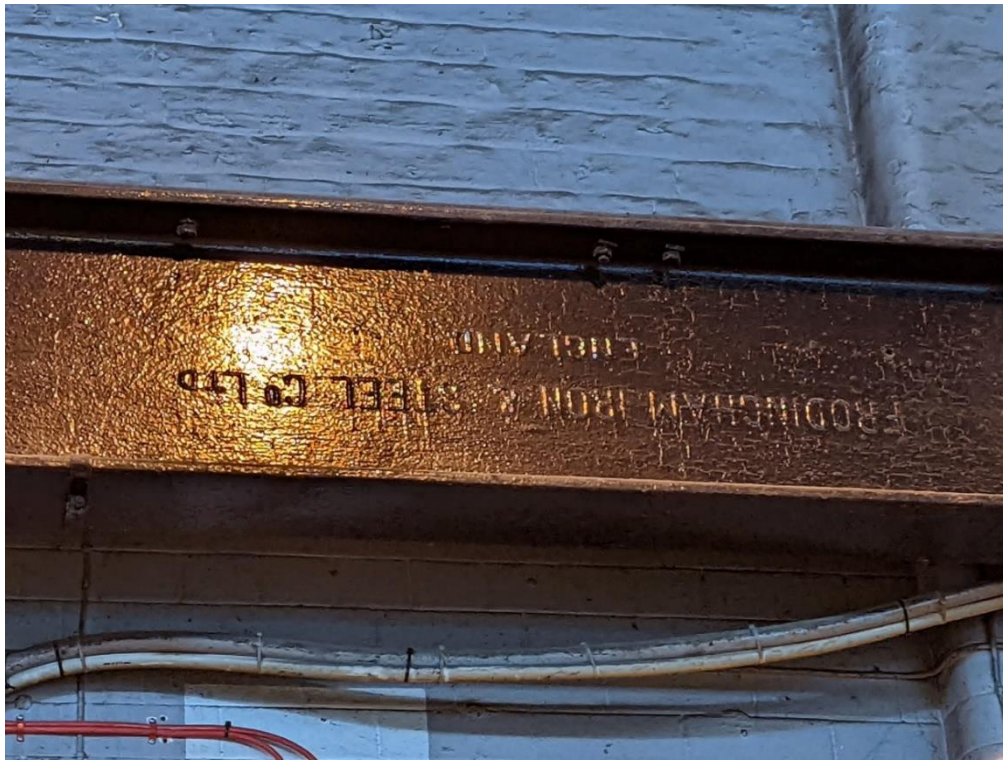
Plate 17: Detail of the RSJ on the west elevation of the undercroft.
