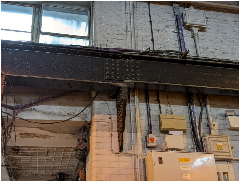
Plate 16: Detail of RSJ on the west elevation of the undercroft.
