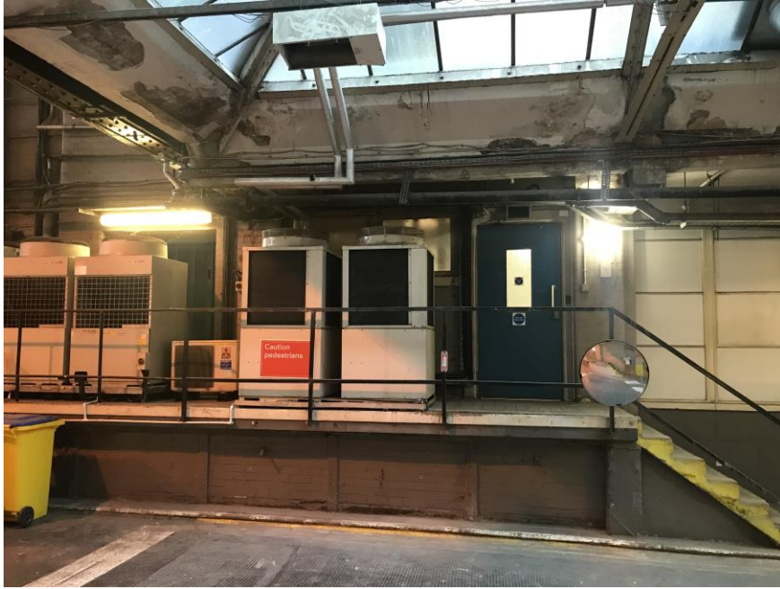
Figure 3: Location of existing windows behind A/C units
