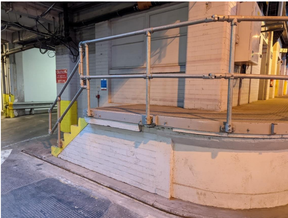
Plate 8: Detail of platform at the south end of the undercroft area.
