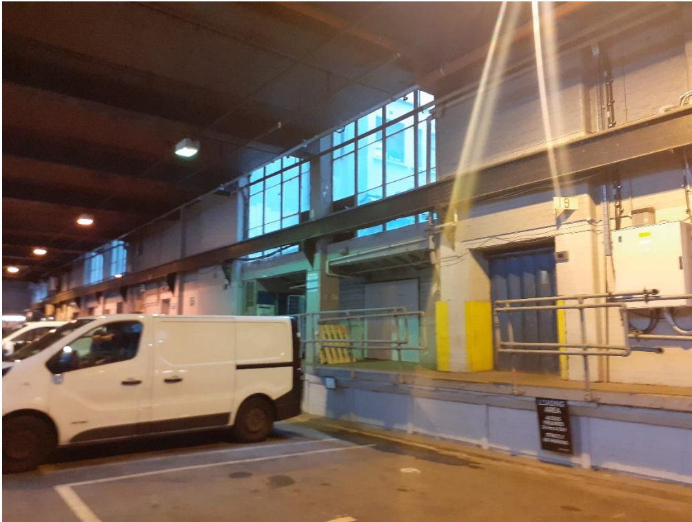
Plate 1: View of west elevation of undercoft wall.
