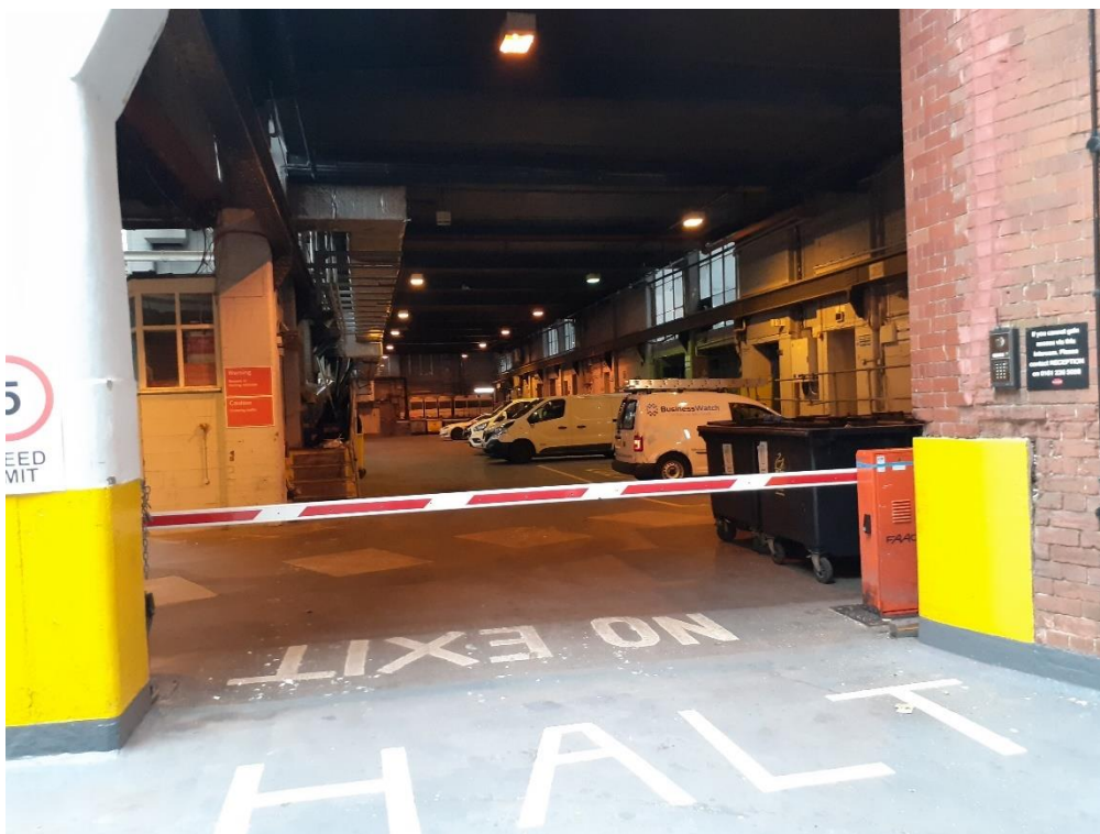
Plate 21: View into the undercroft area looking south.
