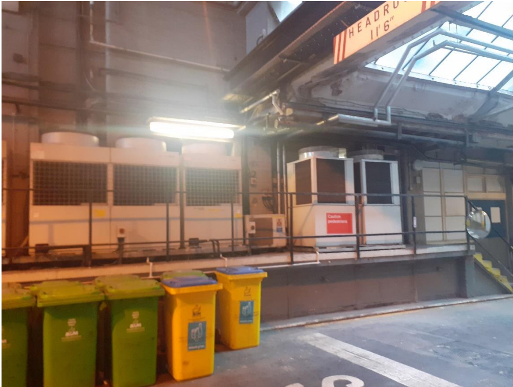
Plate 3: View of south end of undercroft area.
