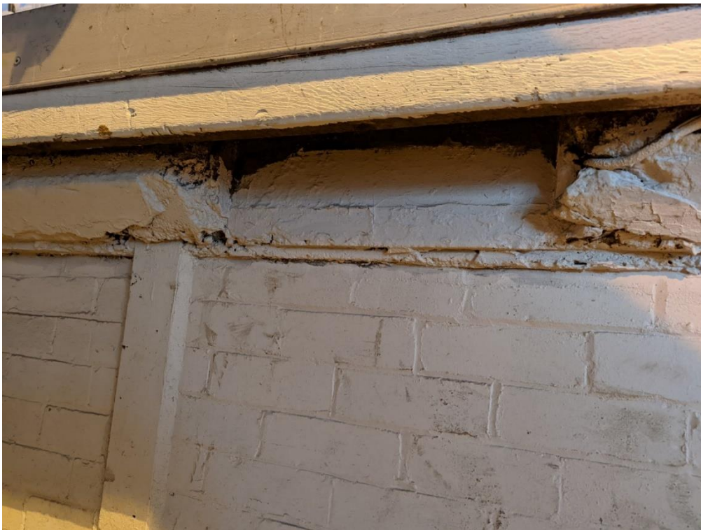
Plate 10: Detail of the area below the undercroft.
