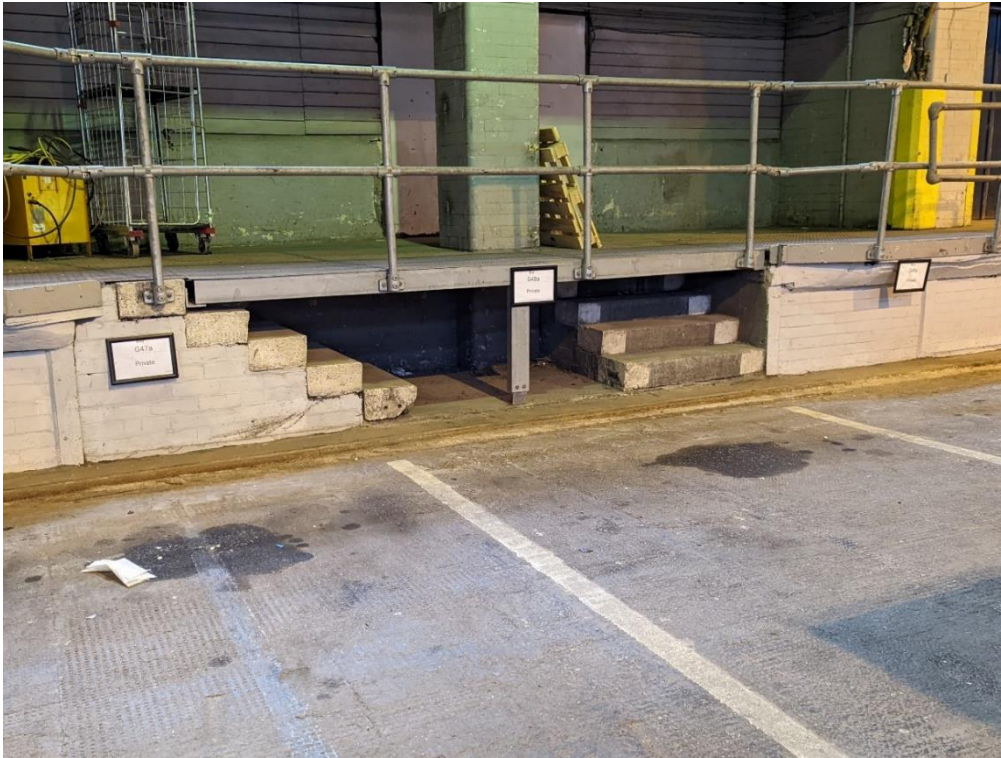
Plate 15: Details of stairs and platform on the south side of the undercroft.
