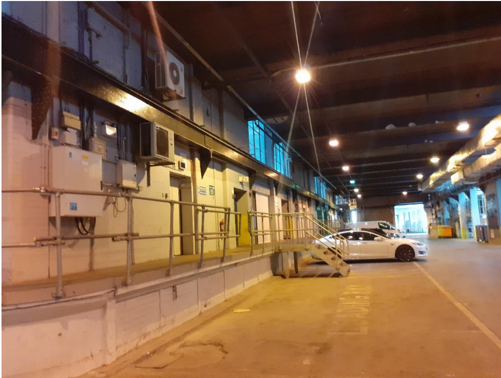
Plate 7: View looking north along the west elevation of the undercroft area.
