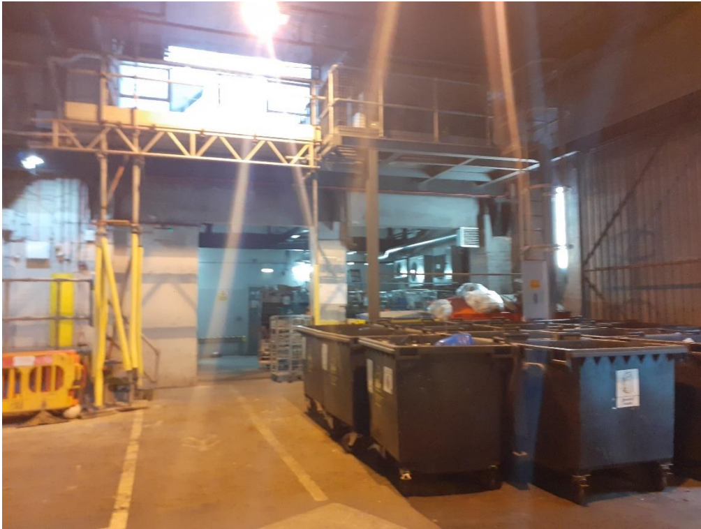
Plate 19: View of bin storage and gantry at the north end of the undercroft area.
