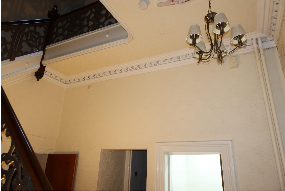
Fig 2: Plaster and joinery details in the stairwell
