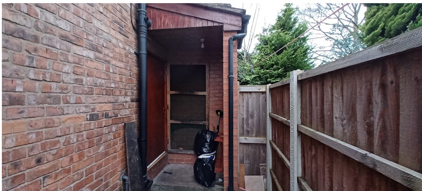
Figure 3. View of existing single storey rear extension (and lack of outdoor amenity space).
