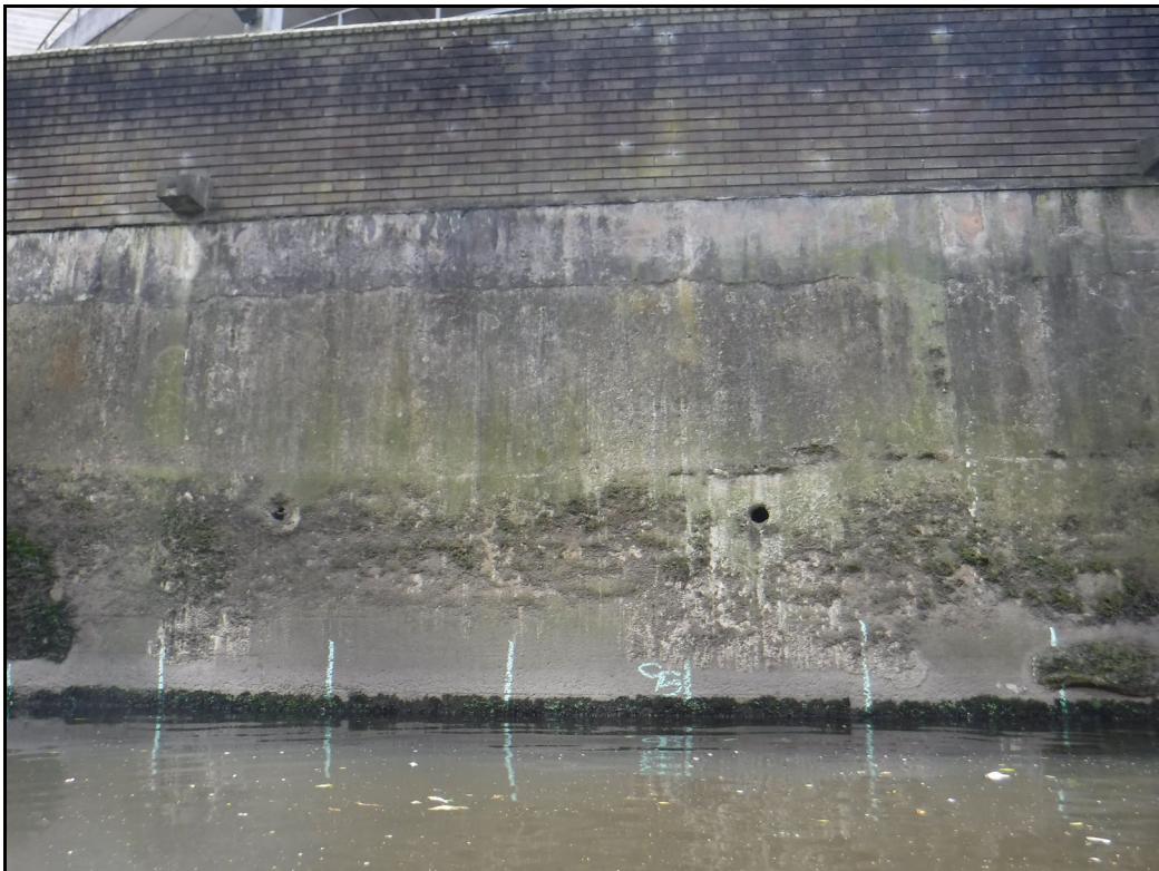
Above:- General view of wall at Ch 70m. Open joints and vegetation growth
