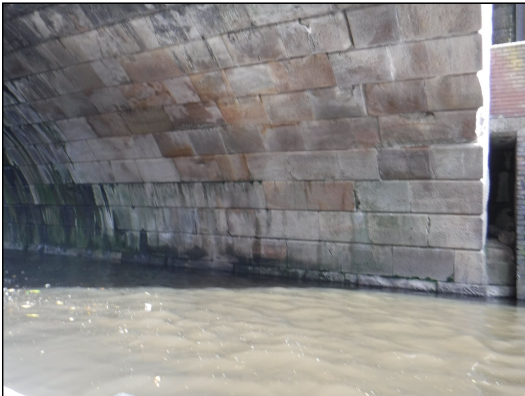
Above:- Ch 0m – 15m Blockwork to Victoria Bridge
