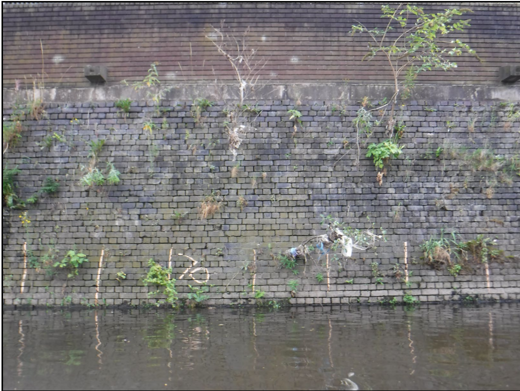
Above:- General view of wall at Ch 70m. Open joints and vegetation growth
