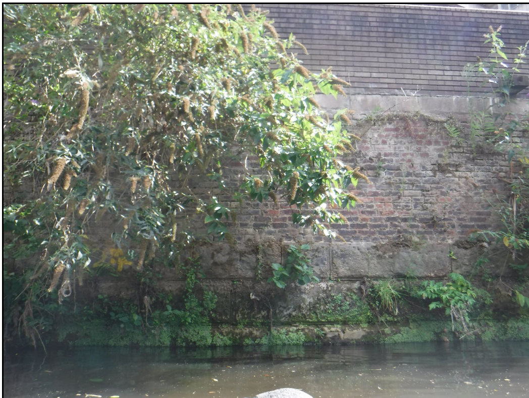
Above:- General view showing condition of wall and construction detail
