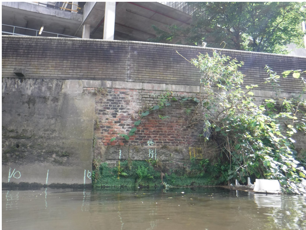
Above:- General of Ch115m showing change in construction detail
