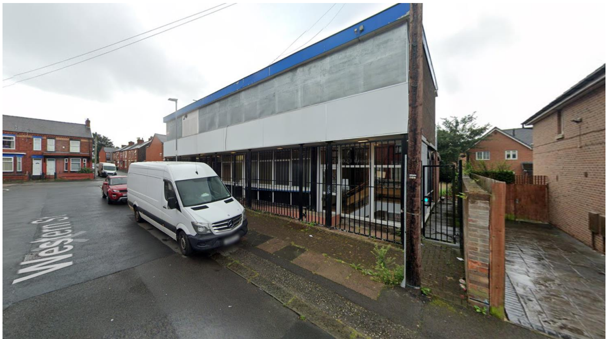
Photo above shows the pedestrian access into the rear yard area from Western Street and the buildings rear elevation.
