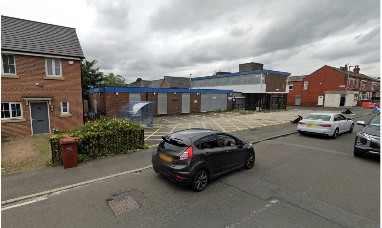
Photo above shows the front of the site from Constable Street, the available parking and turning areas, as well as the secure cycle storage.
