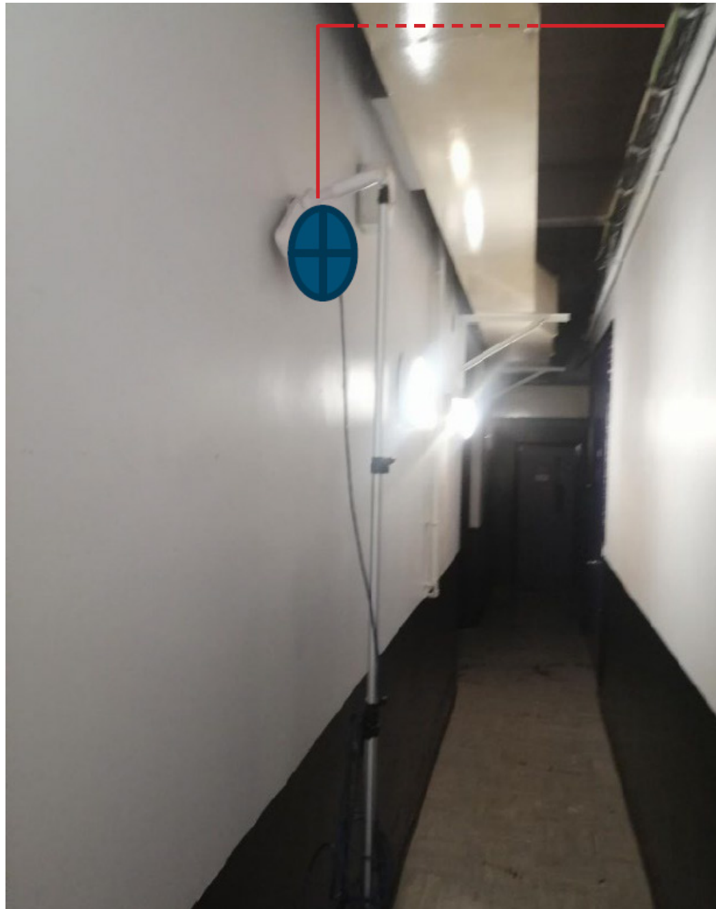
AP 5 - Basement Corridor
