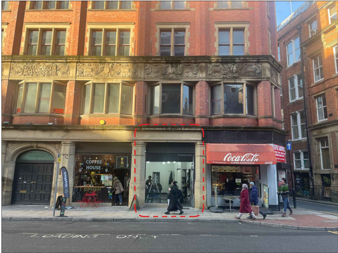
SHOP IN CONTEXT - STREET VIEW - NEWTON STREET
