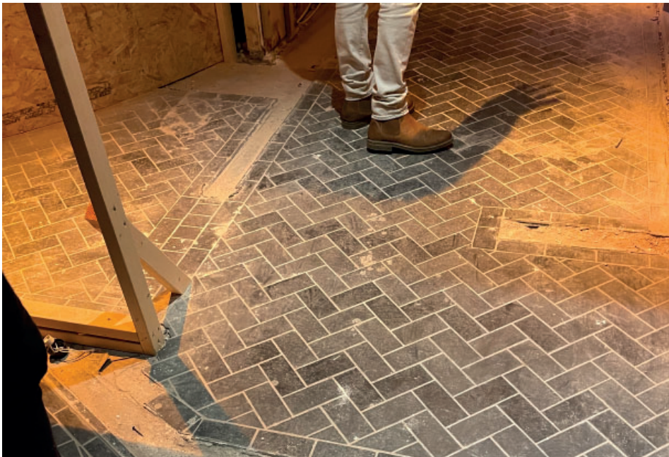
2 View of the tiled finish to be retained
