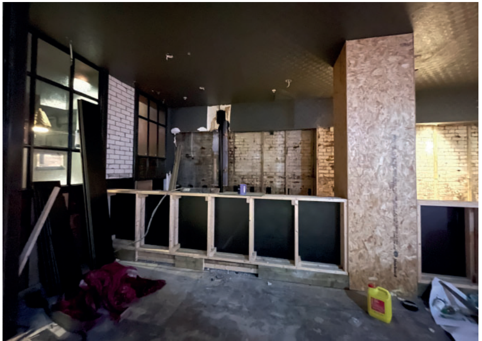
6 View of the reception area
