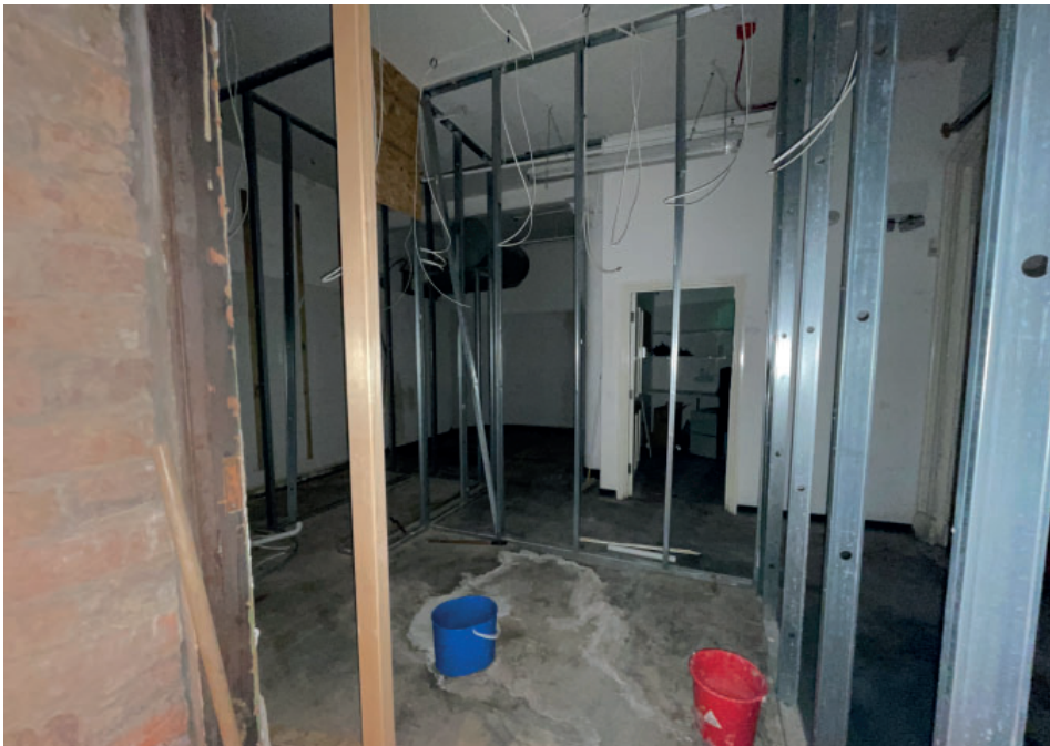
5 View of the existing female changing rooms
