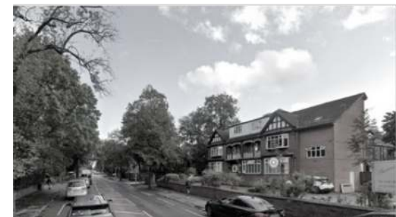
Street View of the Alexandra Care Home
