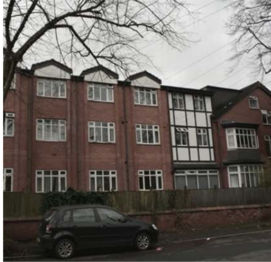
View from Blair Road of the previous extension to the Care Home
