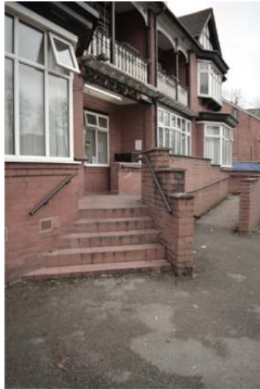
Stairs and Ramp at the front- main access
