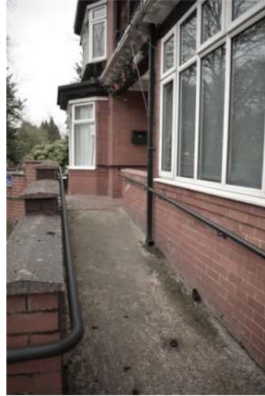
Ramp up to Existing Front Entrance
