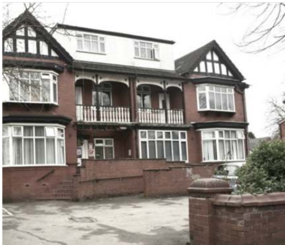
Front View of Alexandra Care Home
