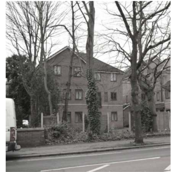
3 Storey Apartment Block opposite the site
