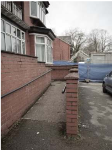
Ramp to Front Entrance
