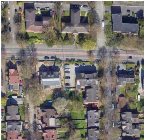
Aerial View of Alexandra Care Home and Immediate Surroundings
