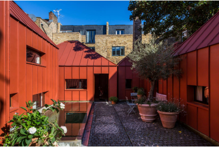
Material Reference : Red standing seam metal by Henning Stummel Architects.
