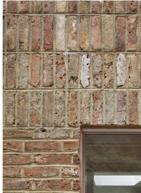
Stack bonded soldier coursing proposed to parapet
