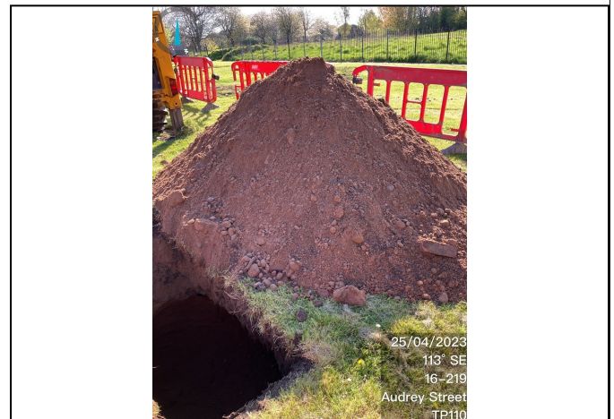
Trial Pit 110 Spoil
