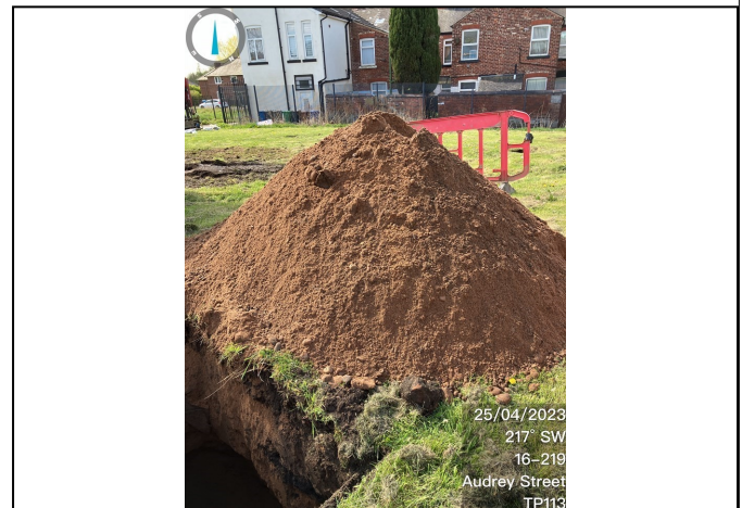
Trial Pit 113 Spoil
