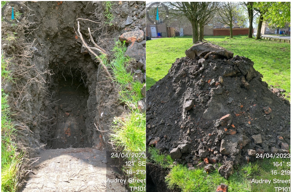
PLATE 3 TP101 EXCAVATION AND ARISING
