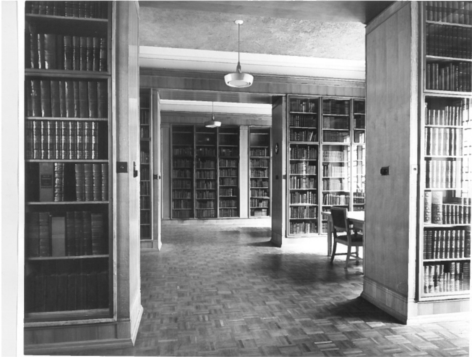
Image from 1962 shows original ceiling arrangement (which does not include the current suspended ceiling). Current suspended ceiling believed to be installed in 1990s when fluorescent lighting was included into the room. Amendments required to this ceiling (including addition of AC units, new lighting, structural alterations and additional MEP) necessitate the installation of a new ceiling. Existing, non-original, ceiling would need to undergo notable repairs and areas of replacement of retained.
