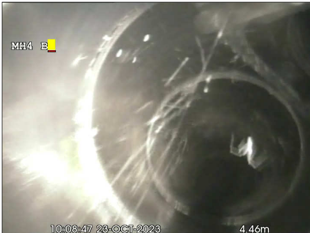
Photo: 58_4a, 00:00:00 4.6m, Junction at 02 o'clock, dia 100 mm
