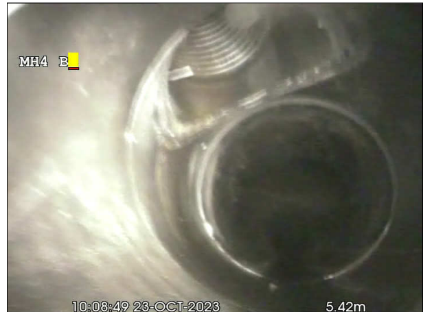
Photo: 59_5a, 00:00:00 5.5m, Junction at 11 o'clock, dia 100 mm
