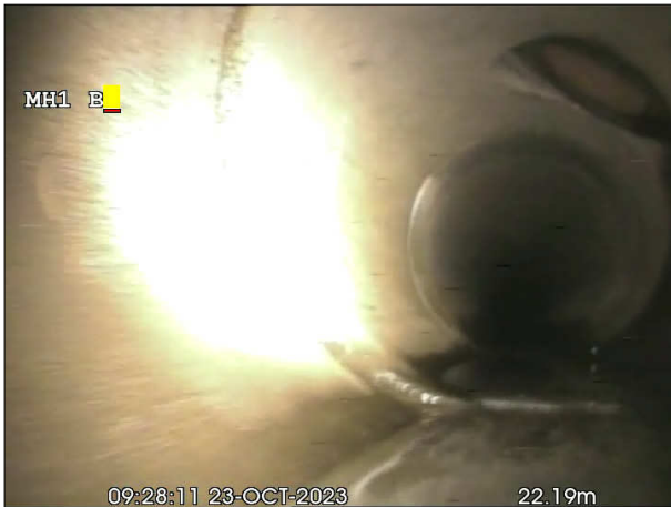
Photo: 20_8a, 00:00:00 23m, Junction at 01 o'clock, dia 150 mm
