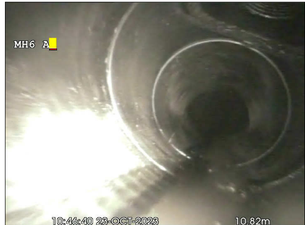
Photo: 80_5a, 00:00:00 11m, Junction at 12 o'clock, dia 150 mm
