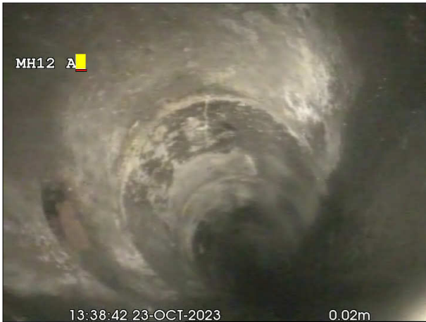
Photo: 189_4a, 00:00:00 0.5m, Junction at 09 o'clock, dia 150 mm
