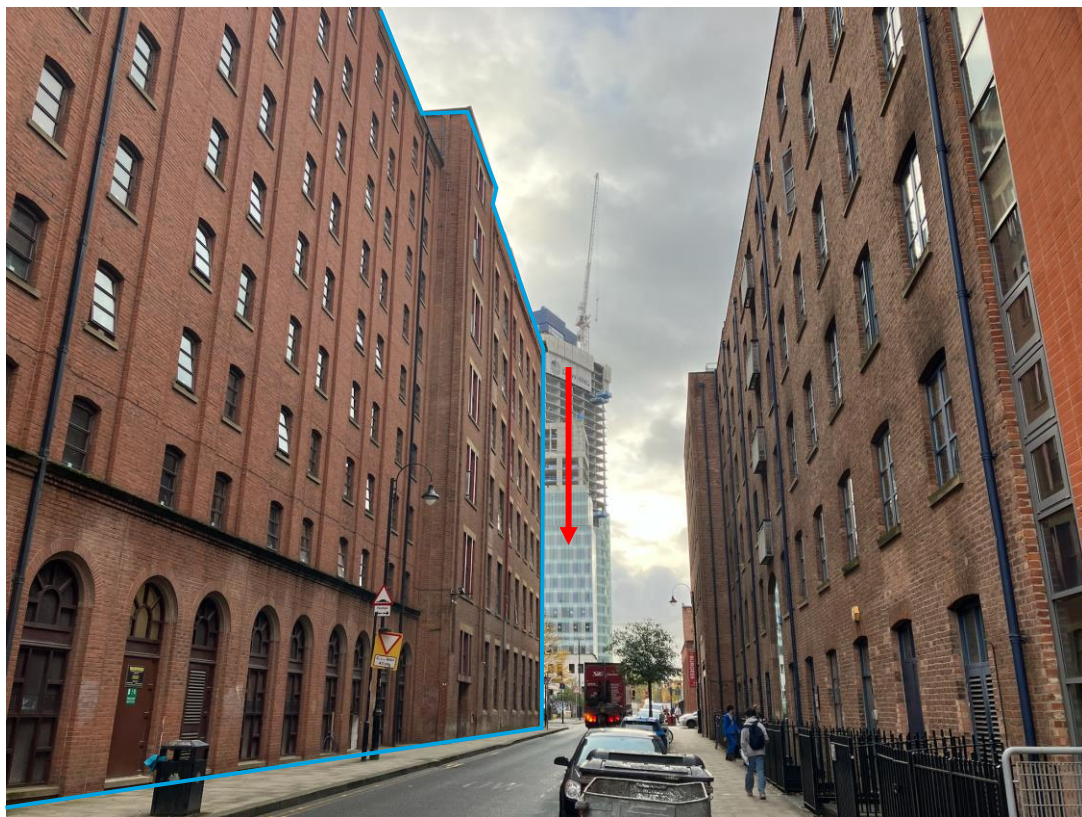
Figure 4.7– View of Chorlton Old Mill from Hulme Street looking west in conjunction with the Site denoted by red arrow and heritage asset edged in blue. (View 17 - Author's own, 2023)
