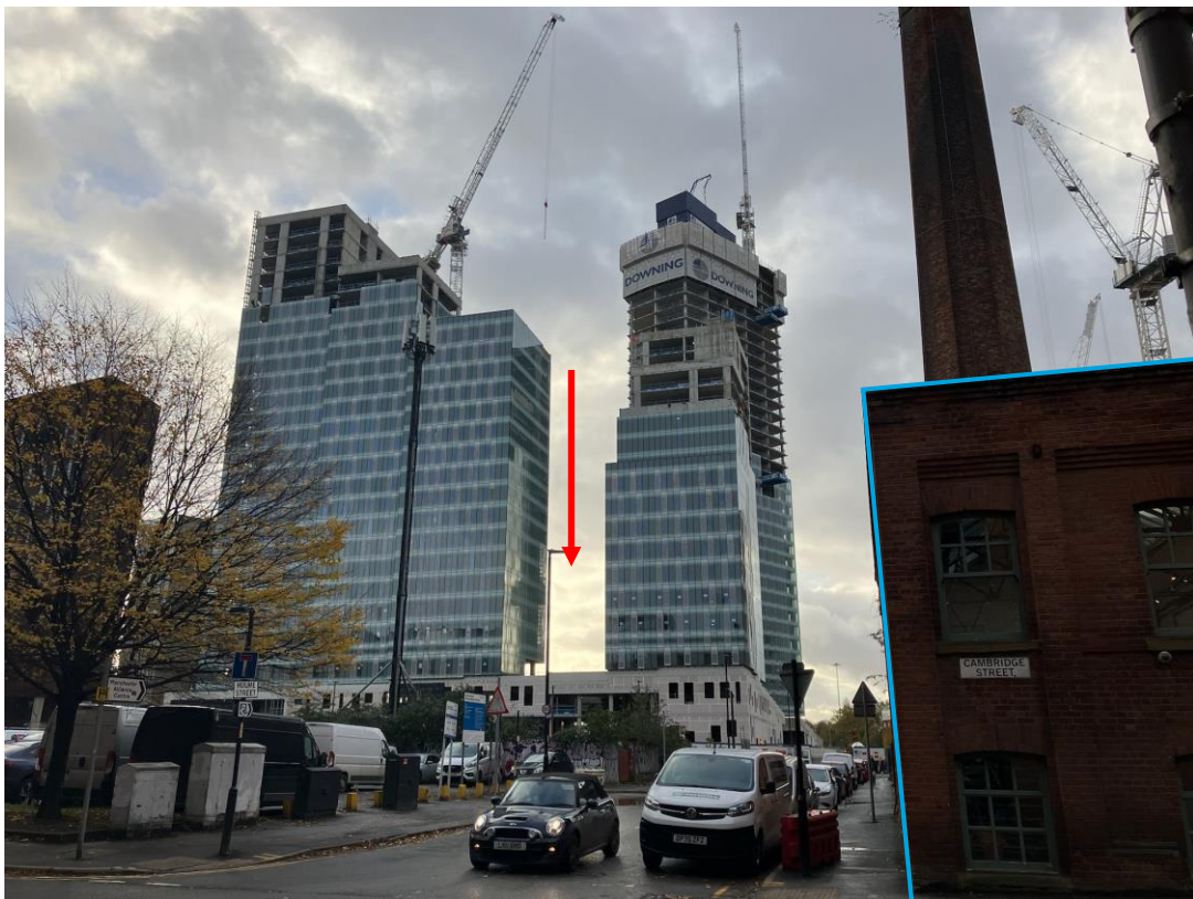
Figure 4.4 – View of Macintosh Mill from Hulme Street looking west in conjunction with the Site denoted by red arrow and heritage asset edged in blue. (View 18 - Author's own, 2023)
