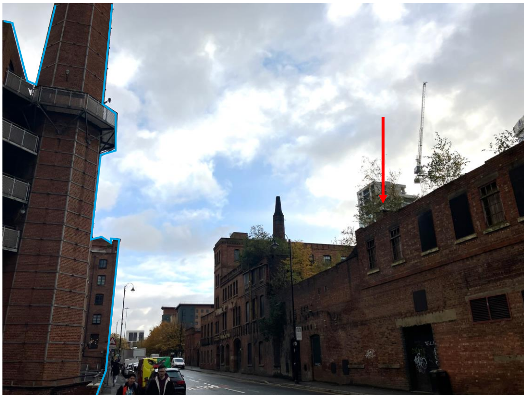
Figure 4.7 – View of Chorlton New Mill from Cambridge Street looking south west in conjunction with the Site denoted by red arrow and heritage asset edged in blue. (View 16 - Author's own, 2023)
