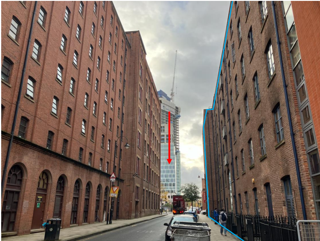
Figure 4.6 – View of Chorlton New Mill from Hulme Street looking west in conjunction with the Site denoted by red arrow and heritage asset edged in blue. (View 17 - Author's own, 2023)
