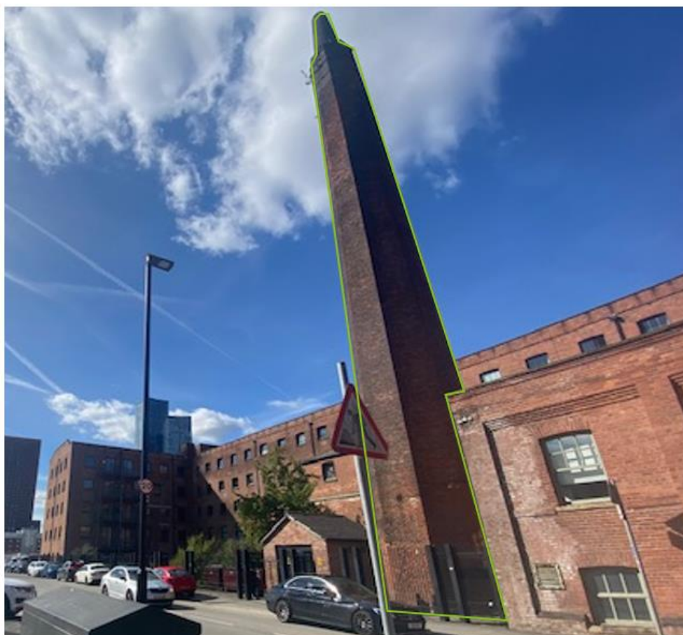
Figure 5.3 –Macintosh Mill Chimney, asset edged in green. (Author’s own, 2022)
