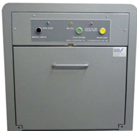
Figure 4.2: Three Way Waste Chute Panel
