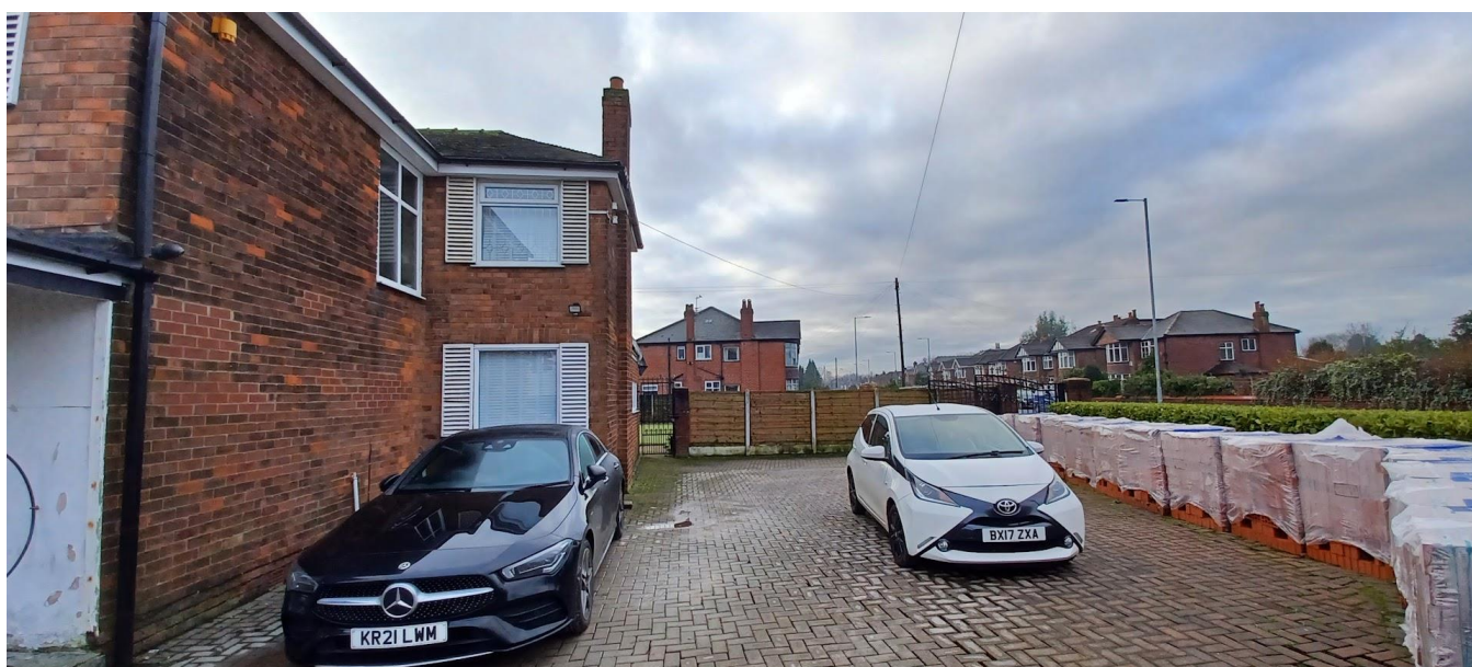
Figure 3. Western side of property.
