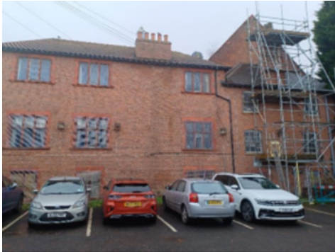
Chimney in Proposal located behind Scaffold.
