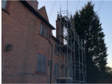
Chimney in Proposal located behind Scaffold.
