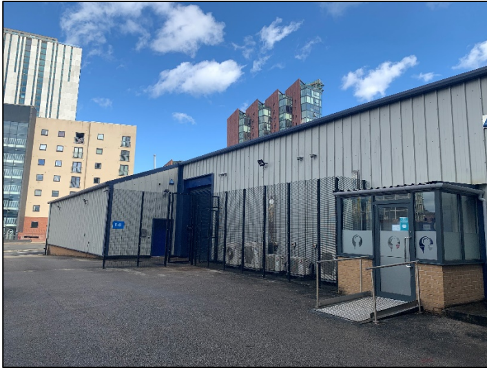
Photo 1 The western metal-clad aspect of the buildings
