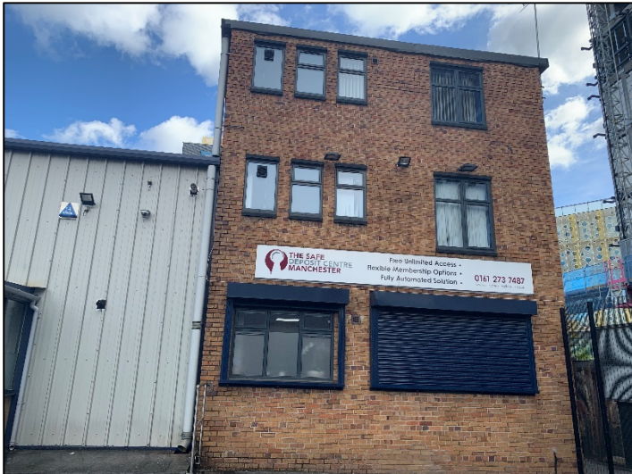
Photo 2 The eastern brick-built aspect of the building
