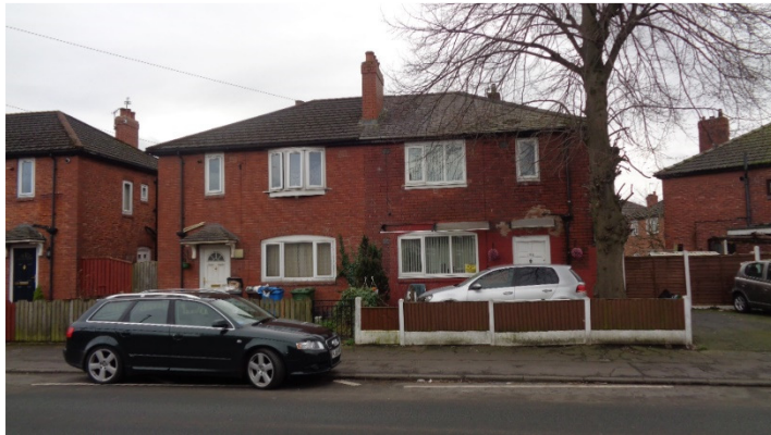
Front Elevation to Application Property.
