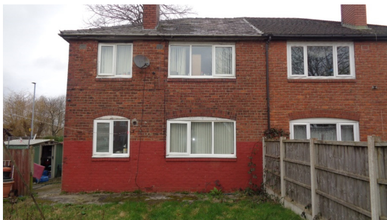
Rear Elevation of Application Property.
