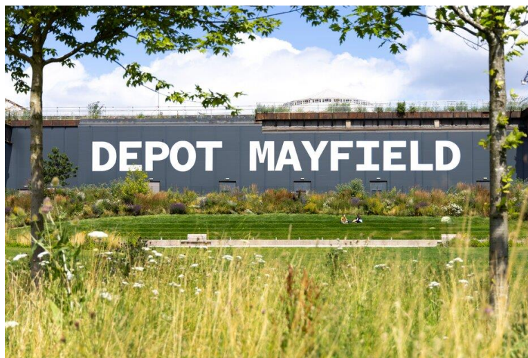
Figure 3.6 – Cladding at Depot Mayfield
