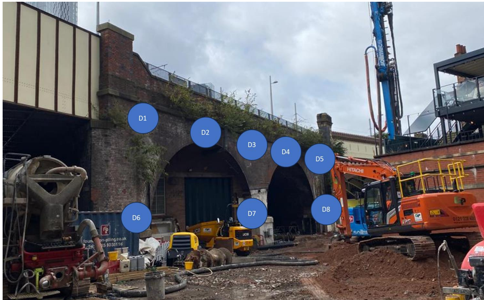
Figure 18 - Viaduct Face, D1-8
