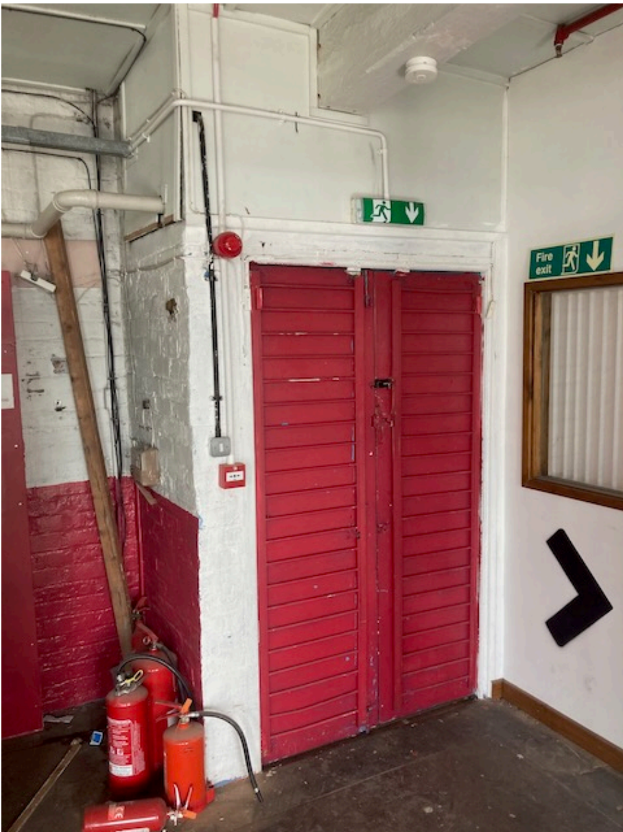
ITEM 21 Brickwork lobby and timber doors to north east stair (office side)
