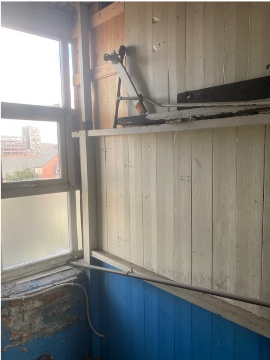
ITEM 33 Timber board partition forming WC area
