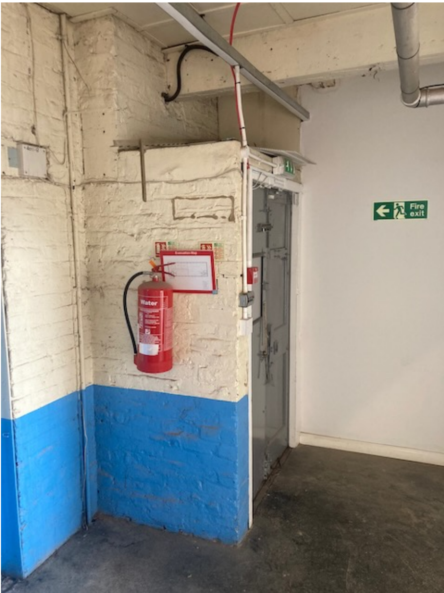
ITEM 31 Brickwork lobby and timber doors to north east stair (office side)
