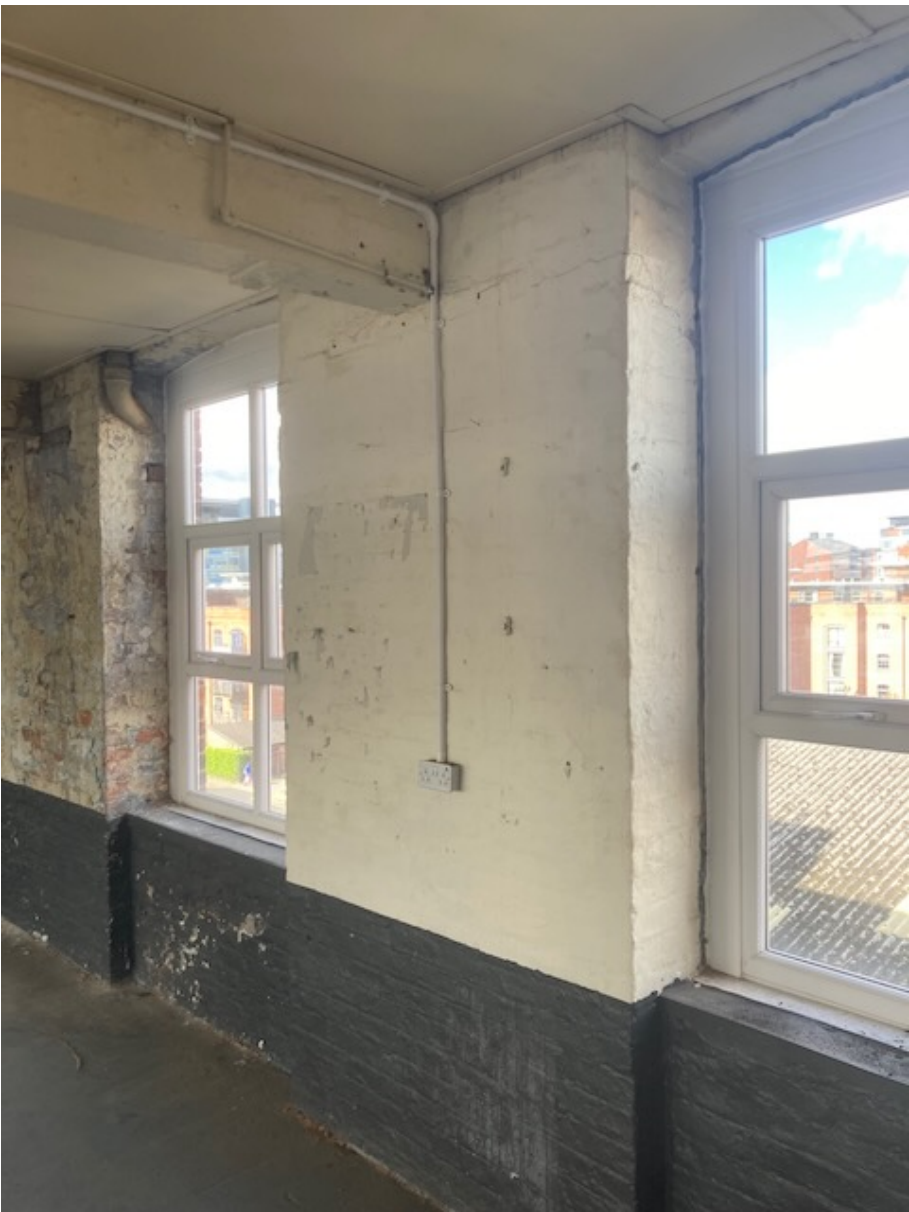
ITEM G6 Typical painted brickwork walls (3rd floor)
