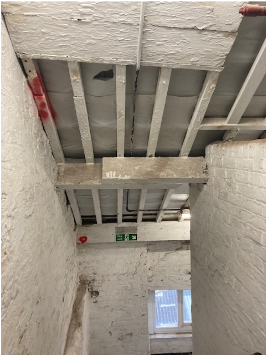
ITEM G12 Timber joists to top floor of north west stair
