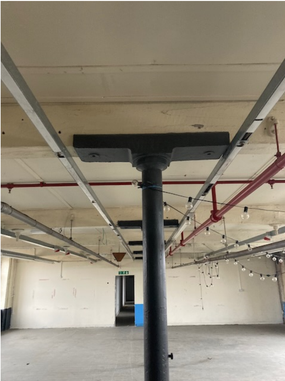
ITEM G1 Typical column and beam shoe at 3rd floor
