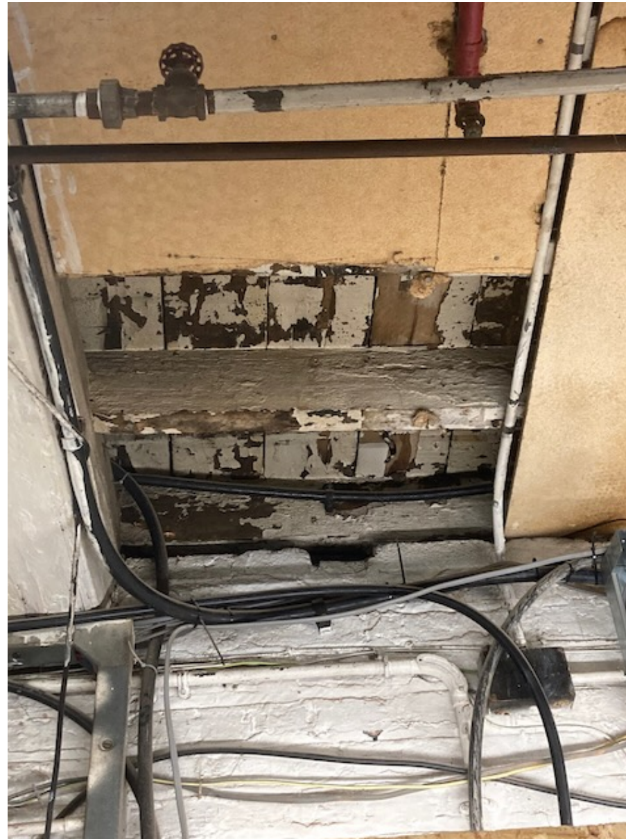
ITEM G3 / G4 Hardboard ceiling to joists at ground floor
