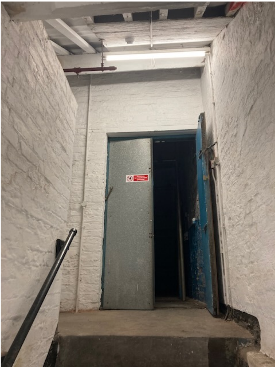
ITEM 46 Timber doors to north west stair
