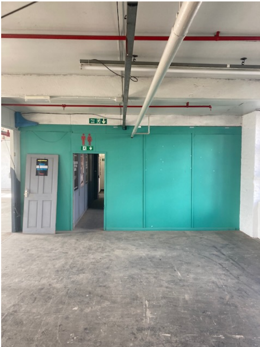
ITEM 23 Boarded partitions forming WC enclosure
