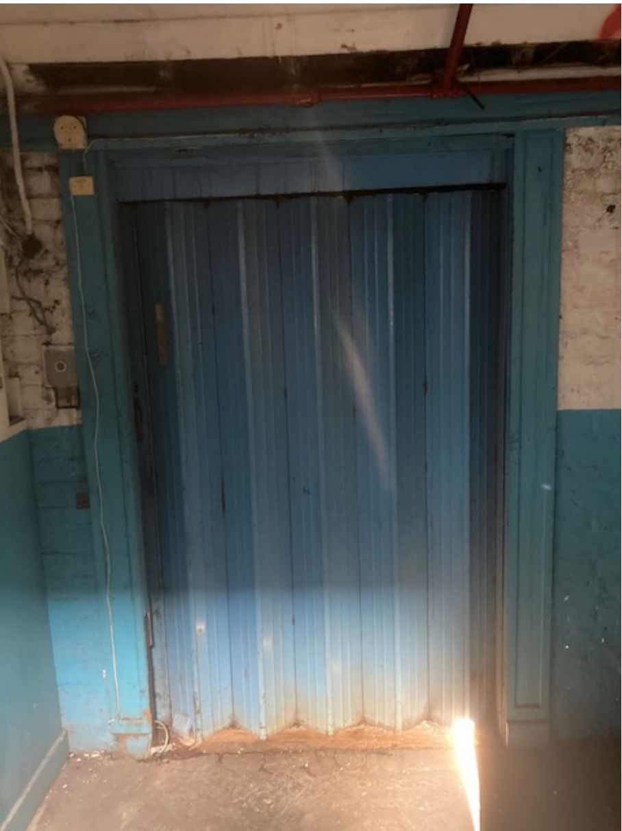
ITEM G7 Internal lift doors at 3rd floor
