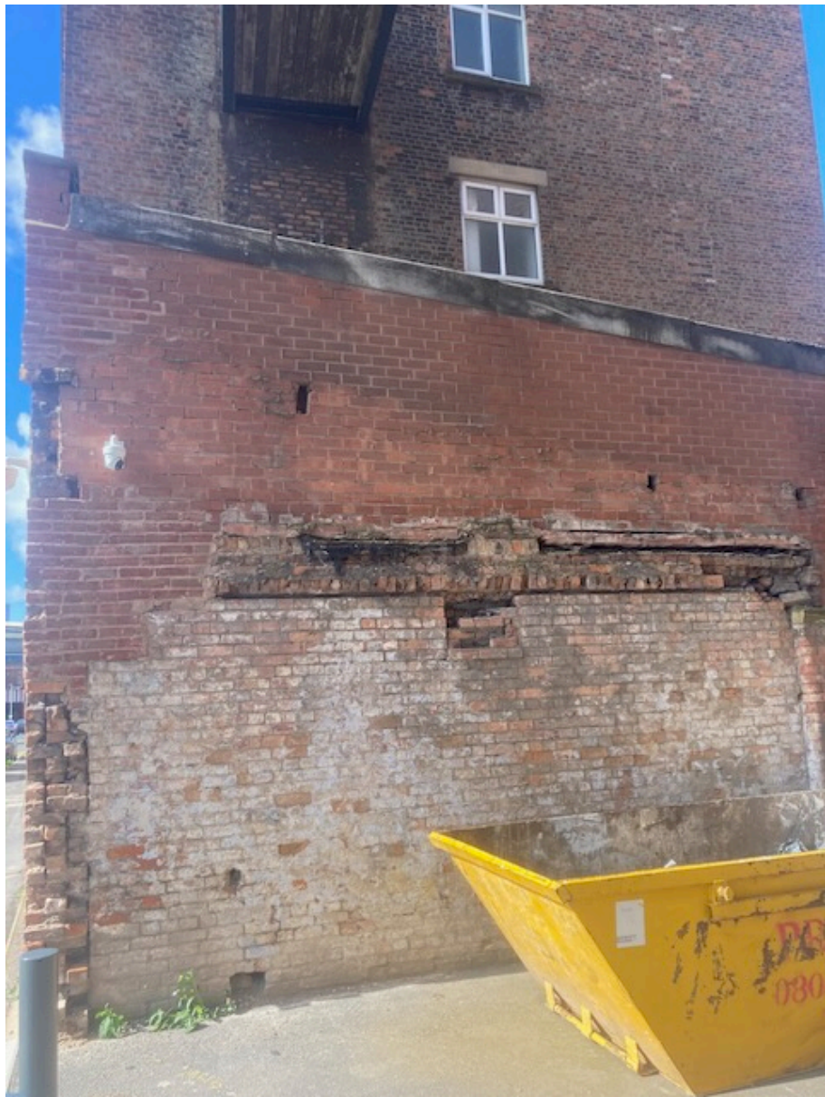
ITEM 01 Single storey offshoot east elevation
