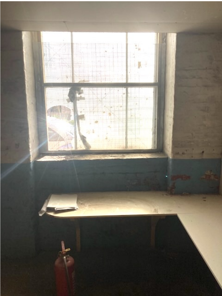
ITEM 06 Internal view brickwork below window to Baird Street ground floor
