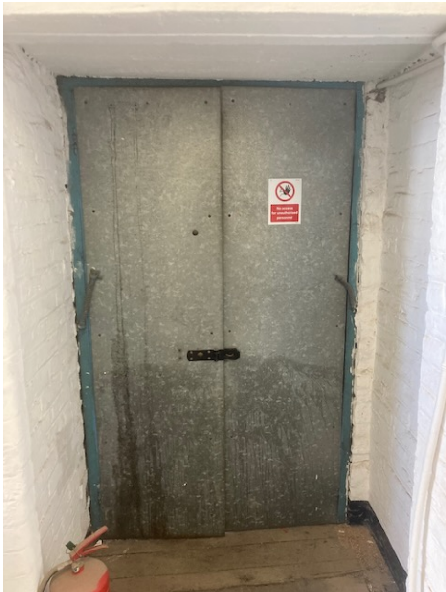
ITEM 32 Brickwork lobby and timber doors to north west stair (stair side)
