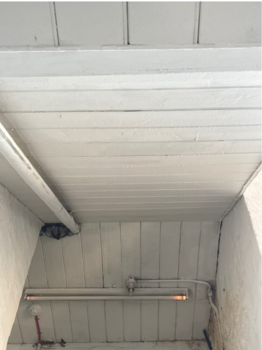
ITEM G11 Typical timber soffit to north east stair
