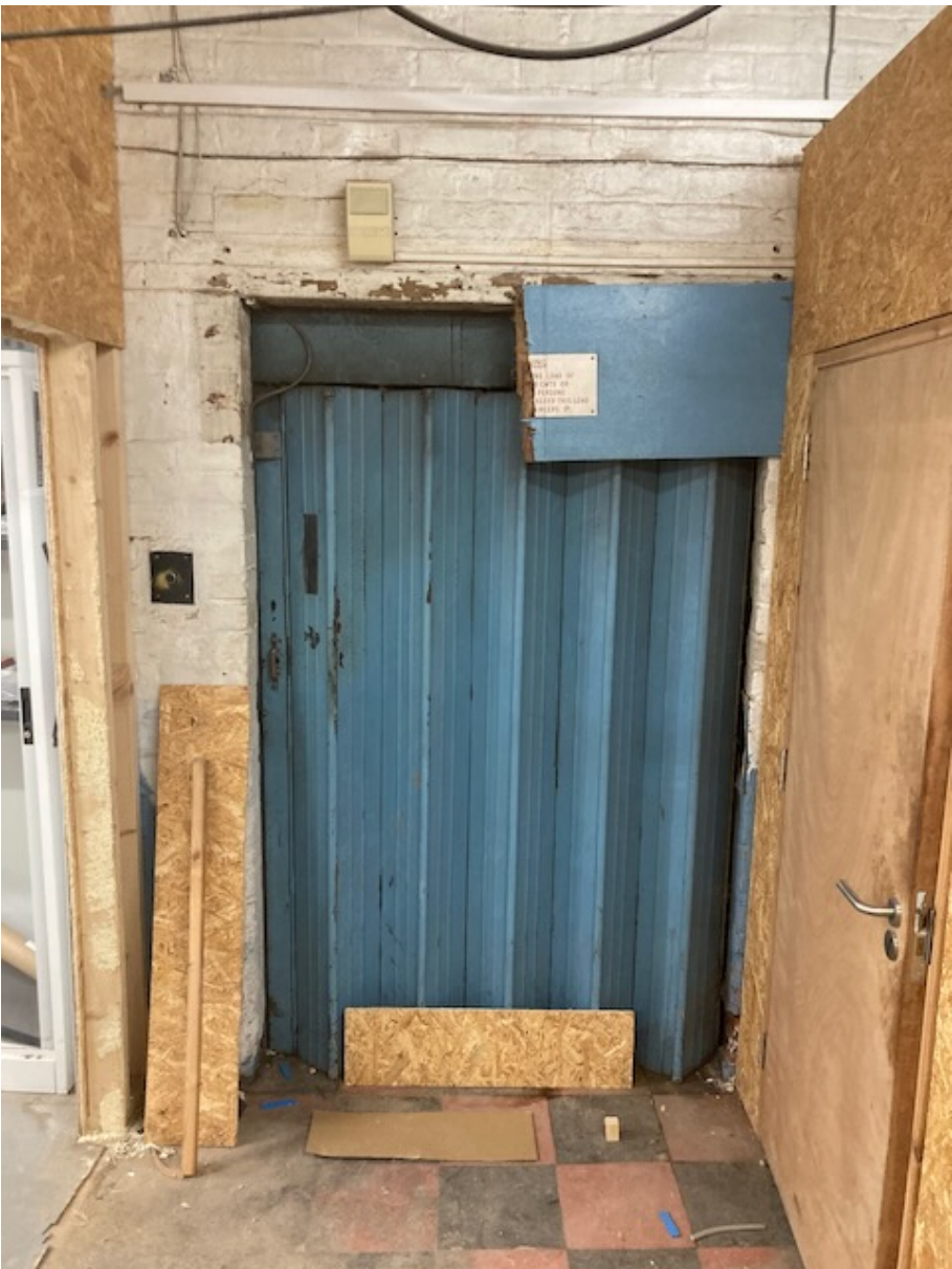
ITEM G7 Internal lift doors at ground floor
