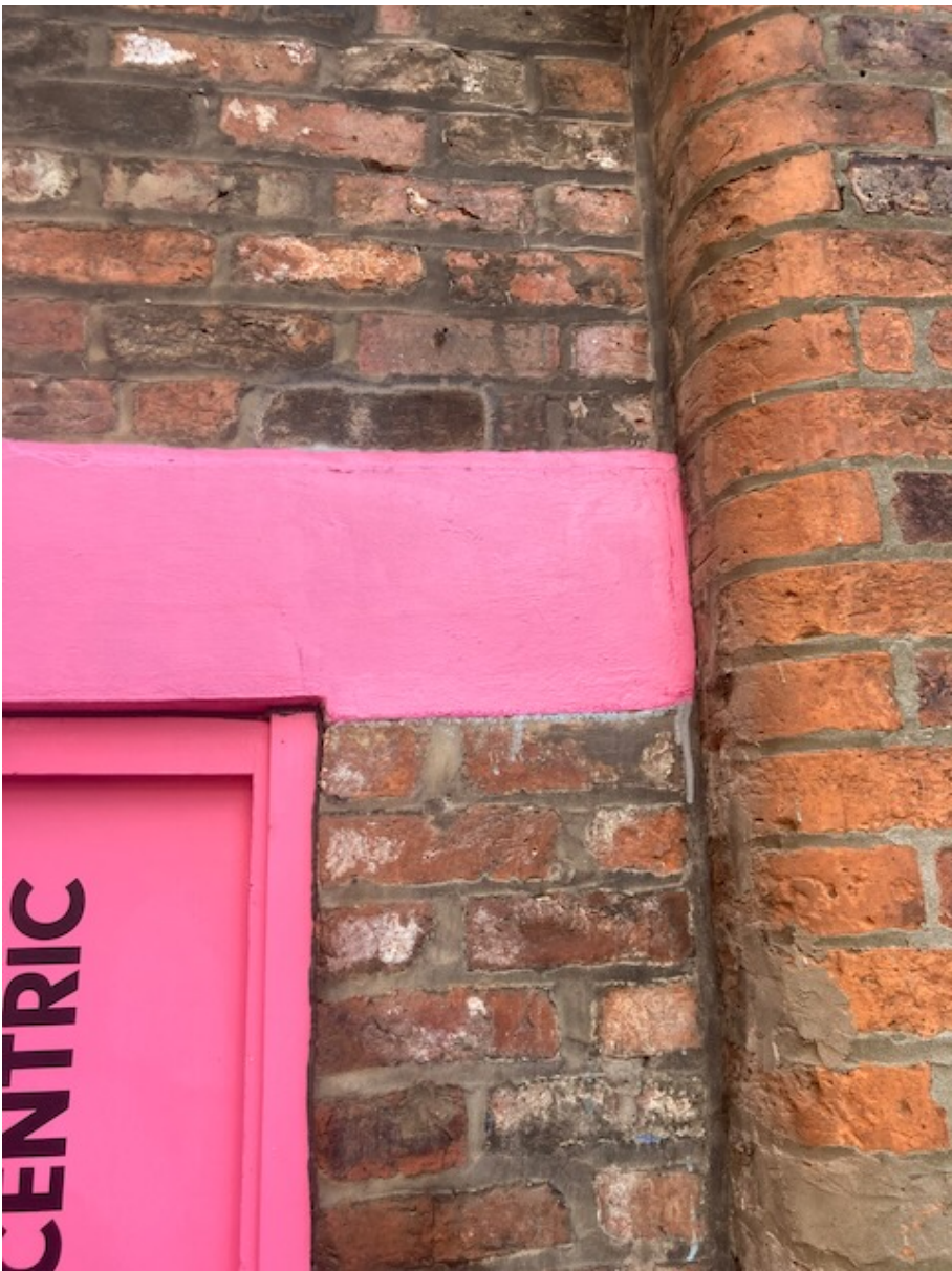
ITEM 03 Painted stone lintel to head of entrance opening
