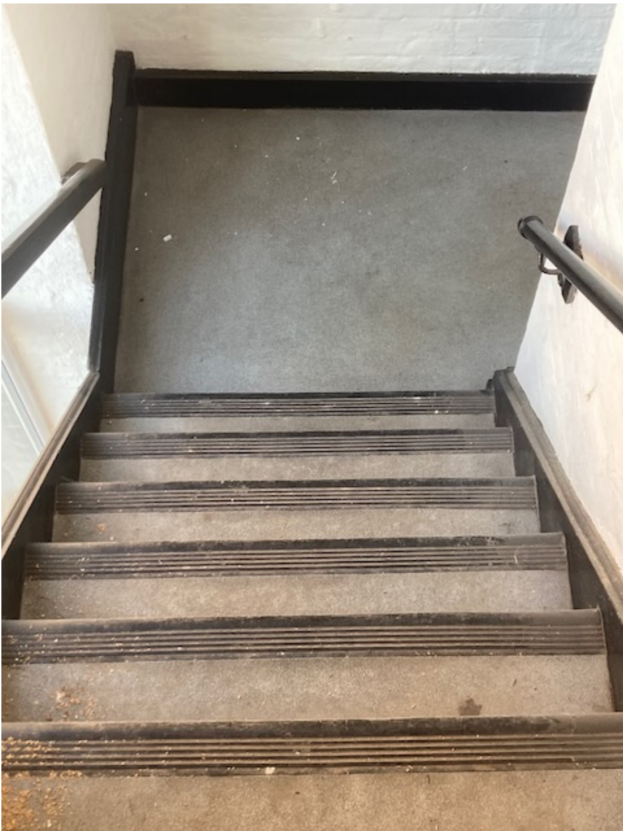
ITEM G11 Typical vinyl floor covering to north east stair
