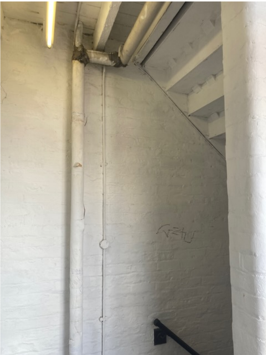
ITEM G11 Typical painted walls to north east stair
