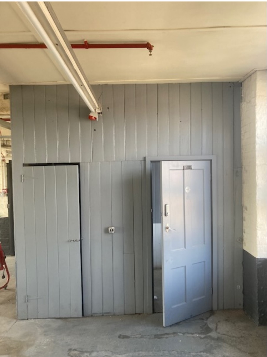
ITEM 33 Timber board partition forming WC area
