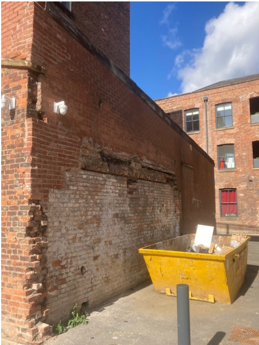
ITEM 01 Single storey offshoot east elevation
