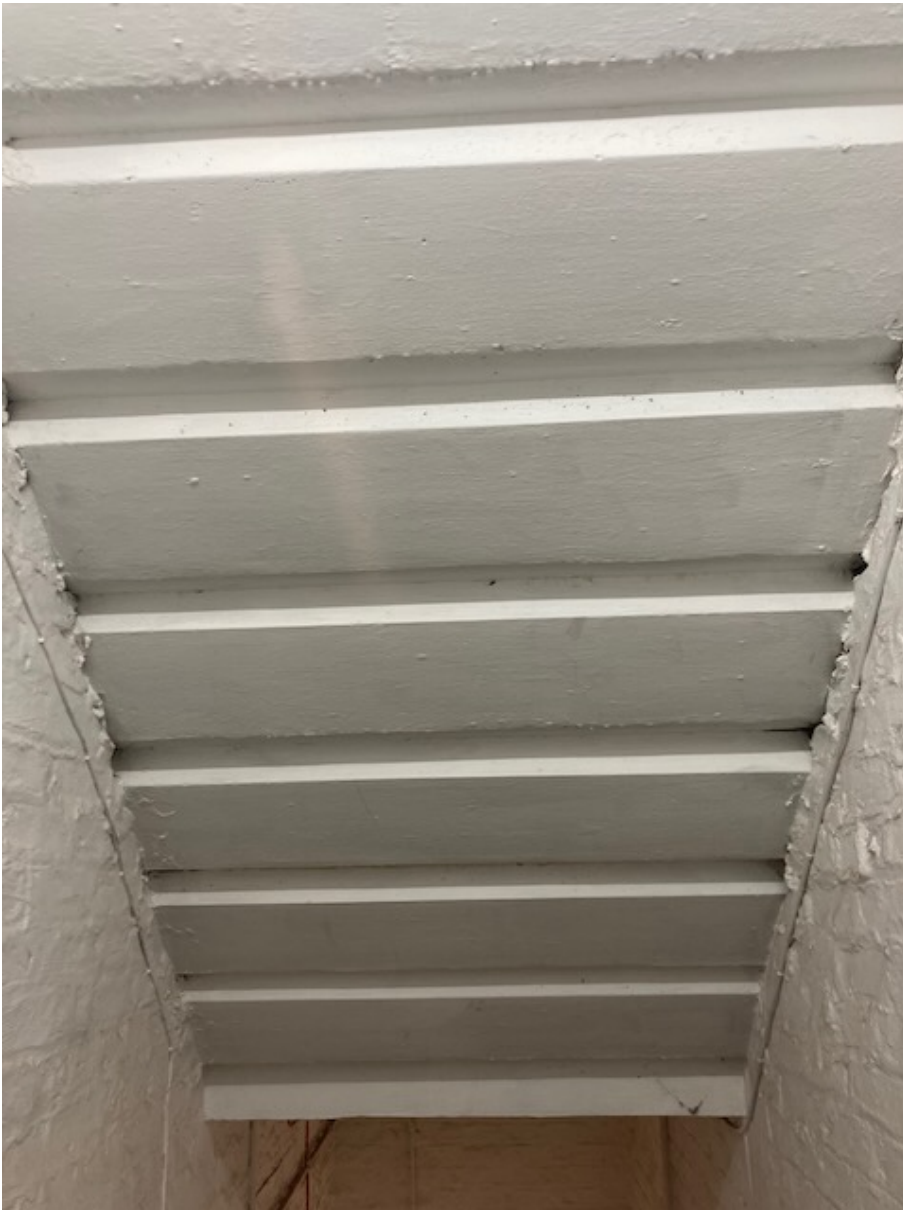
ITEM G12 Painted concrete soffit to flights in north west stair
