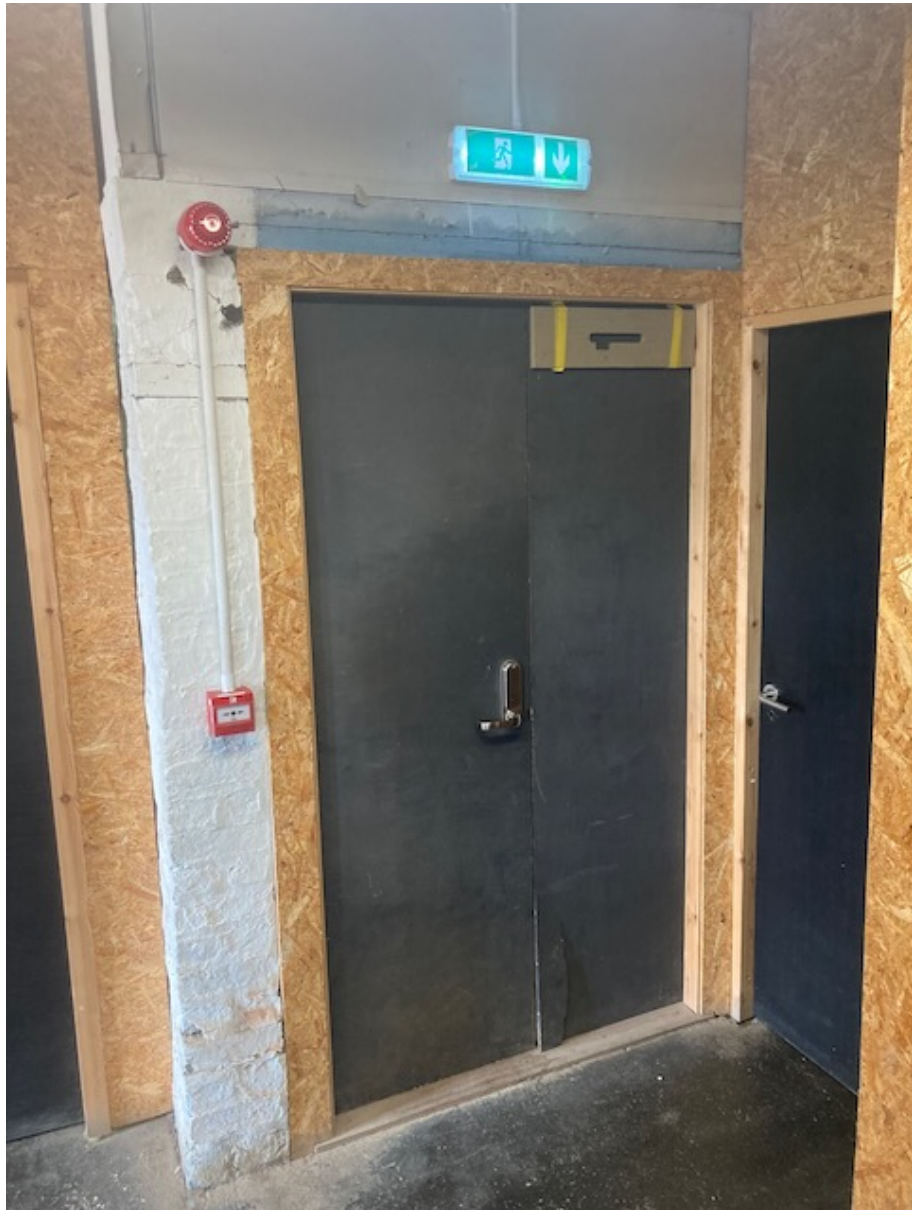
ITEM 12 Brickwork lobby and timber doors to north west stair (office side)
