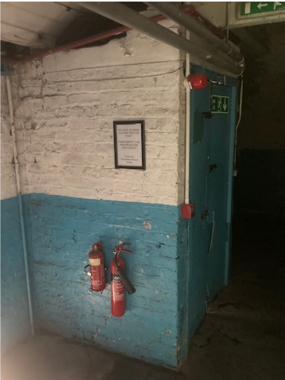
ITEM 45 Brick lobby and timber doors to north east stair (office side)
