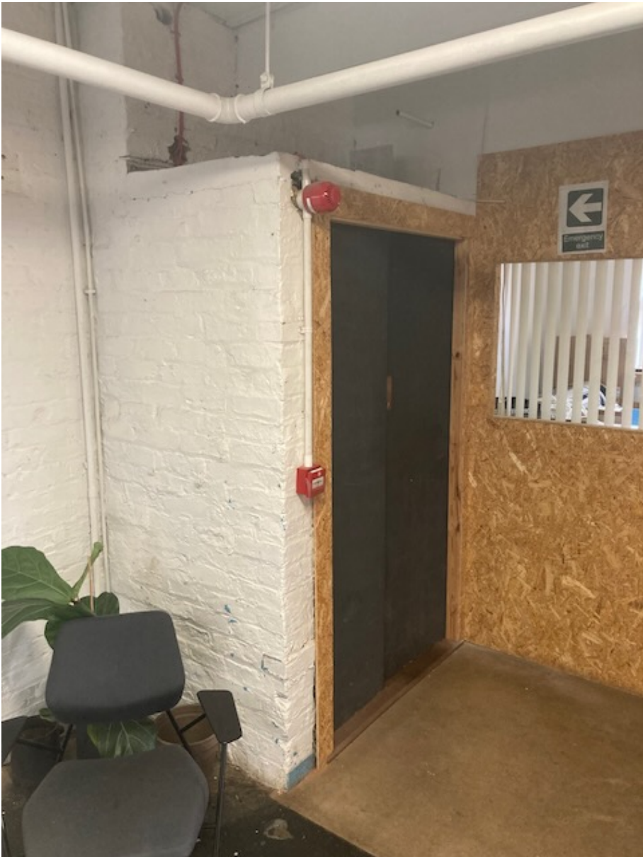
ITEM 11 Brickwork lobby and timber doors to north east stair (office side)
