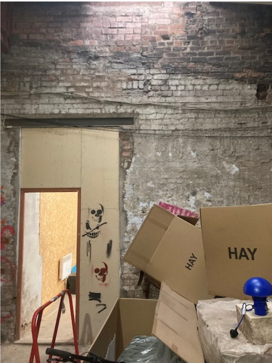
ITEM 02 Brickwork and features to external face of east gable
