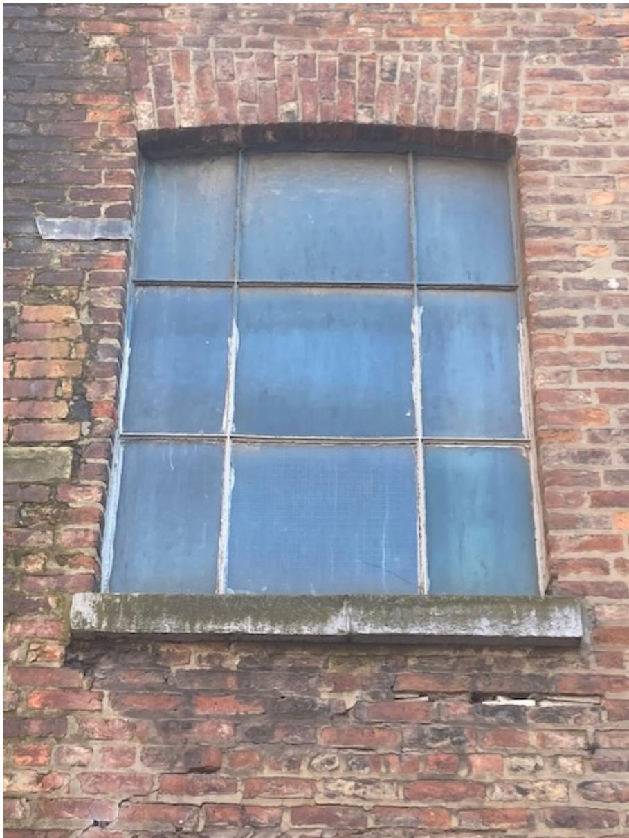
ITEM G13 Typical metal window to lift shaft on north elevation
