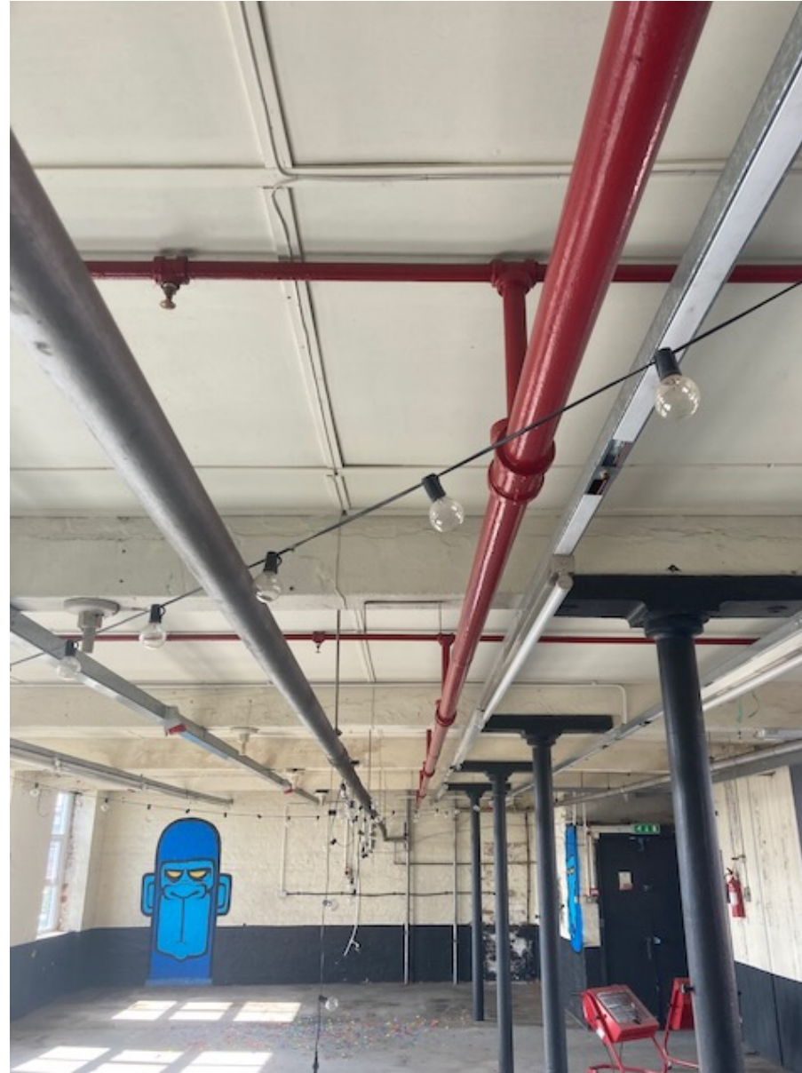
ITEM G8 Typical sprinkler pipework layout
