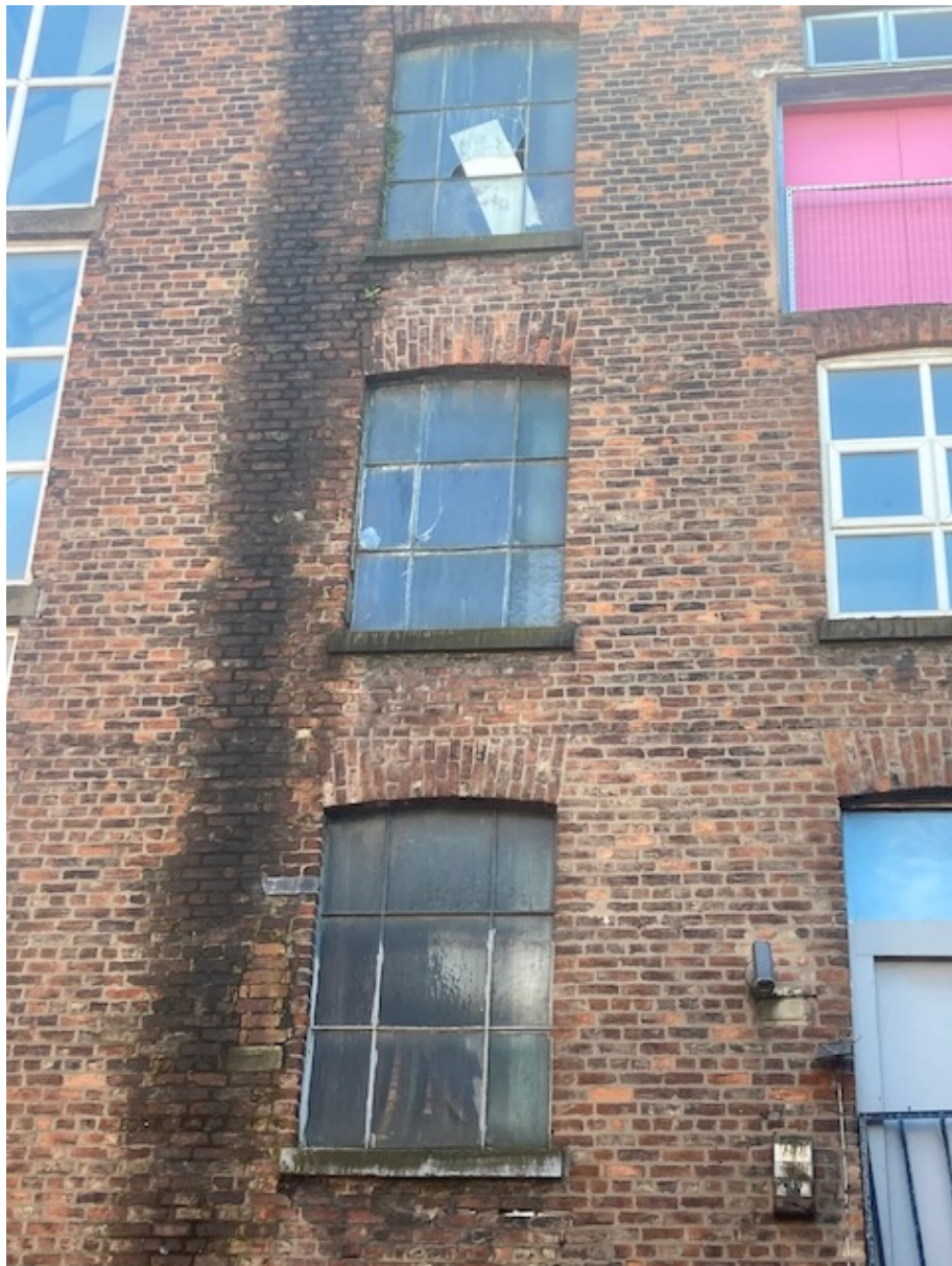
ITEM G13 Group of three metal windows to lift shaft on north elevation
