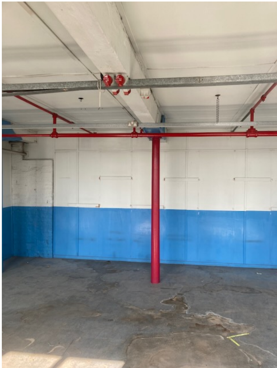
ITEM 23 Boarded partitions forming WC enclosure
