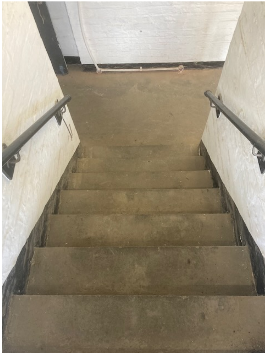
ITEM G12 Typical concrete stairs to north west stair
