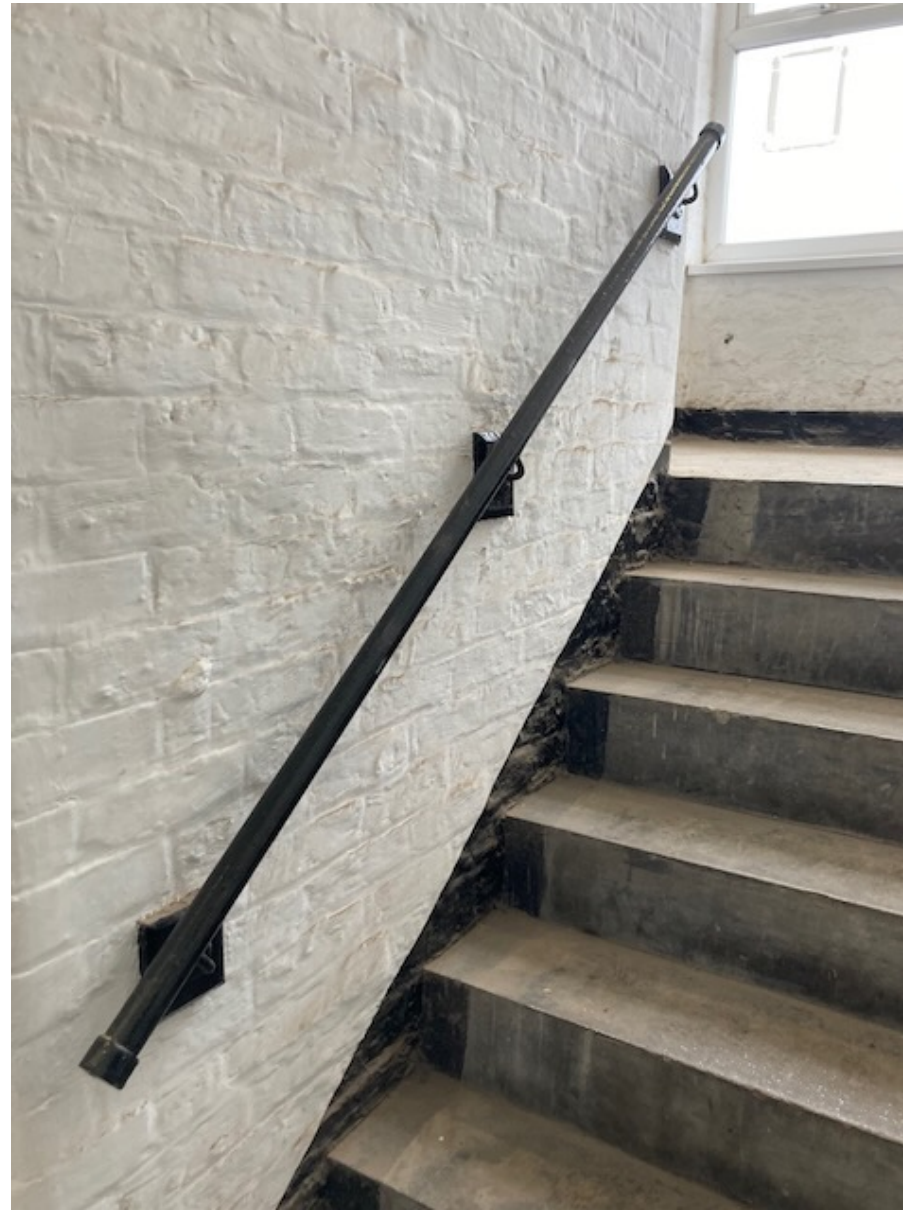
ITEM G12 Painted walls, concrete steps and steel handrails to north west stair
