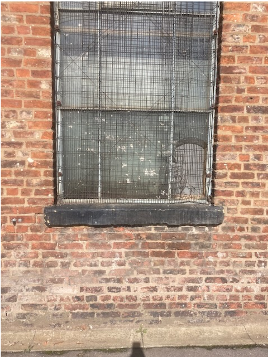
ITEM 06 Cill and brickwork below to Baird Street ground floor
