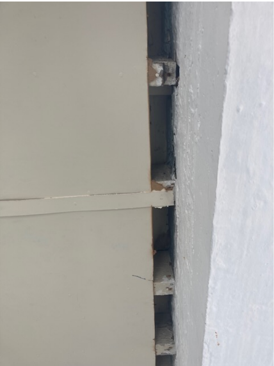
ITEM G5 Typical board ceiling to upper floors with edge trim removed to show joists
