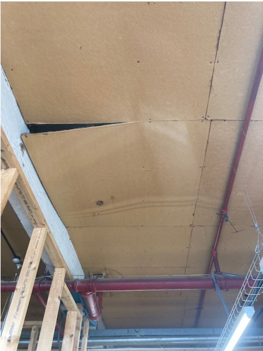
ITEM G5 Hardboard ceiling to ground floor
