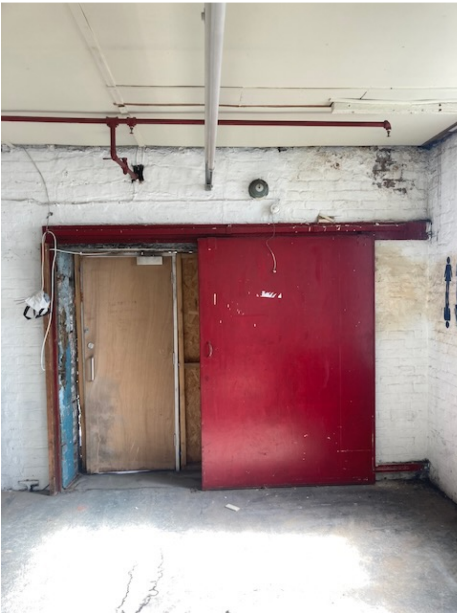
ITEM 34 Sliding door and track to bridge link access
