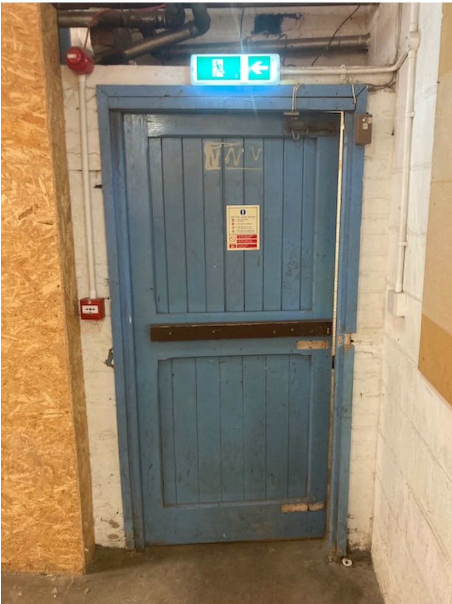
ITEM 04 Access door to north west stair (office side)
