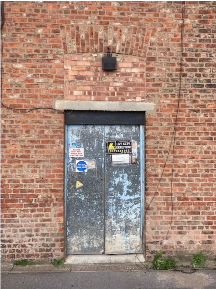
ITEM 08 Infill brickwork, concrete lintel and timber doors to Baird Street opening
