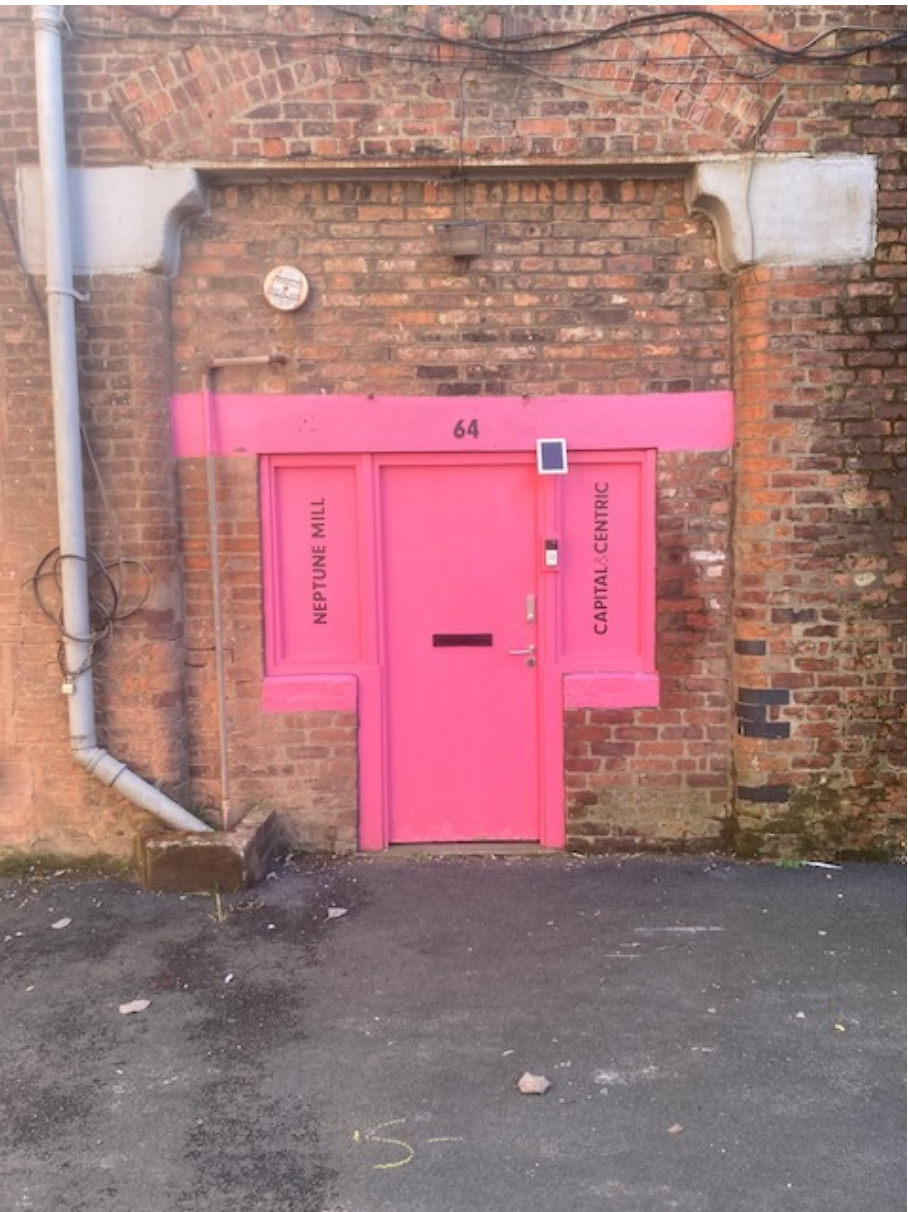
ITEM 03 Brickwork opening with stone lintel to north elevation
