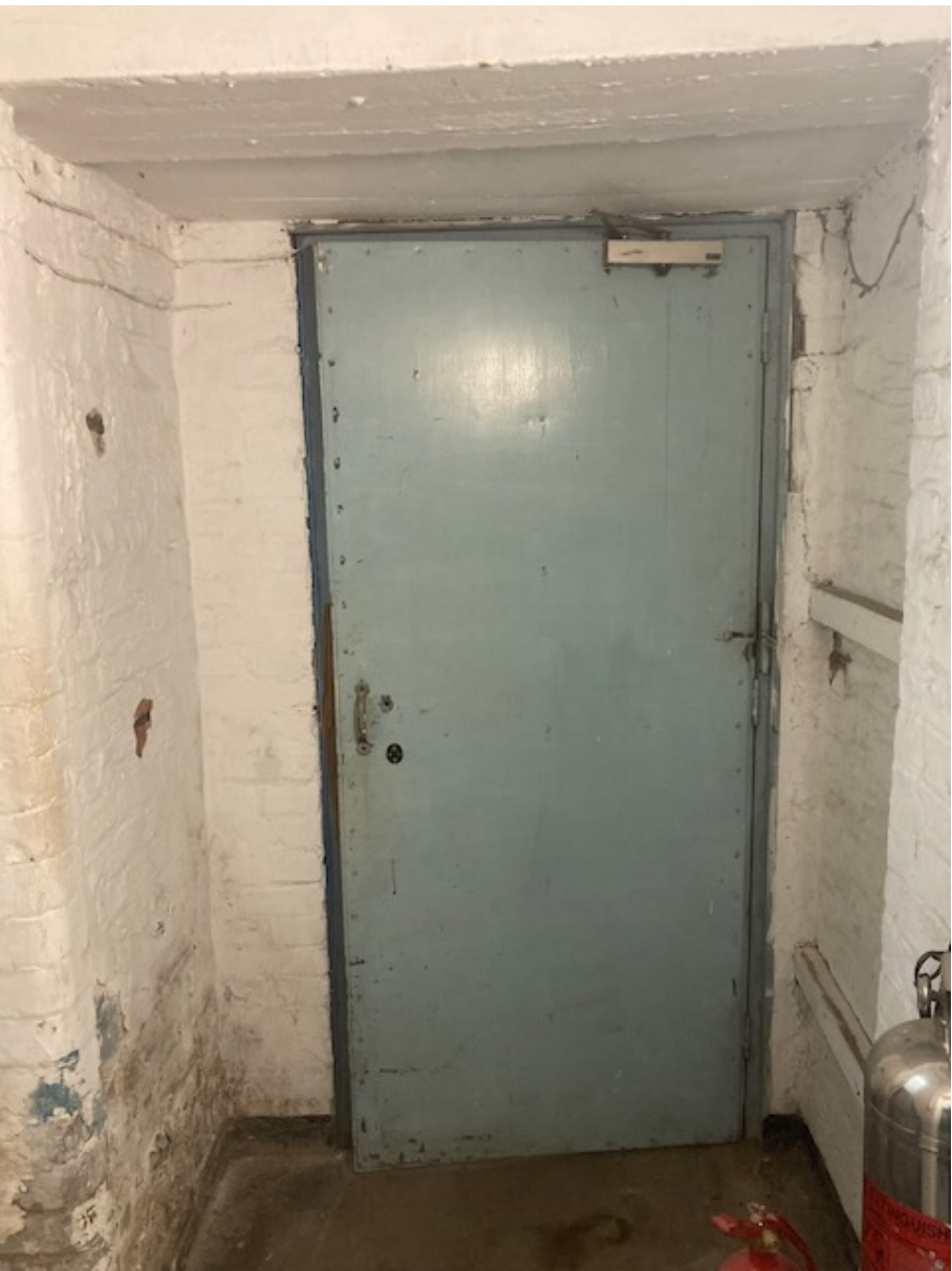
ITEM 04 Access door to north west stair (staircase side)
