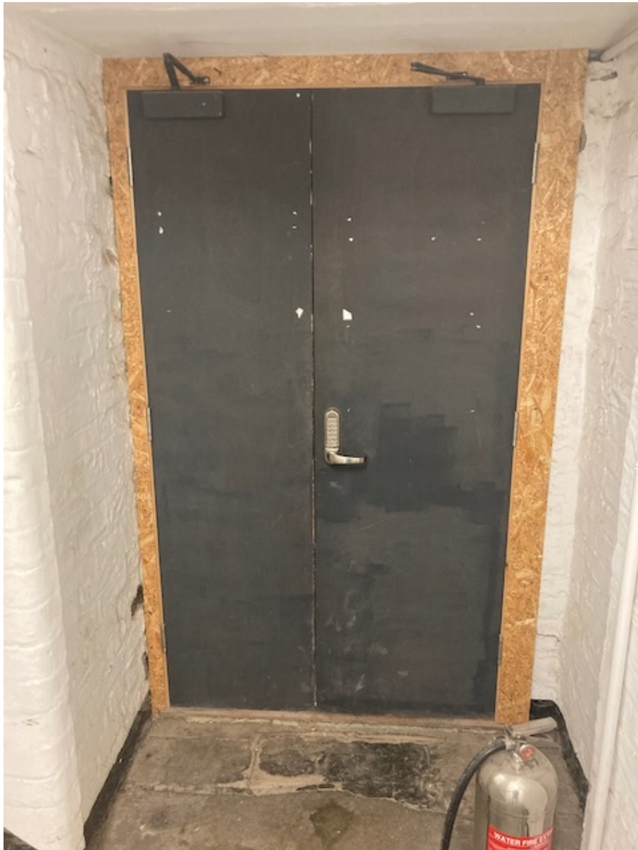
ITEM 12 Brickwork lobby and timber doors to north west stair (stair side)
