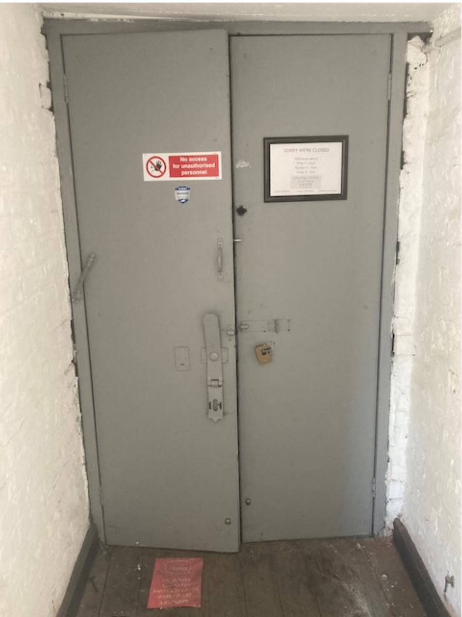
ITEM 45 Brick lobby and timber doors to north east stair (stair side)
