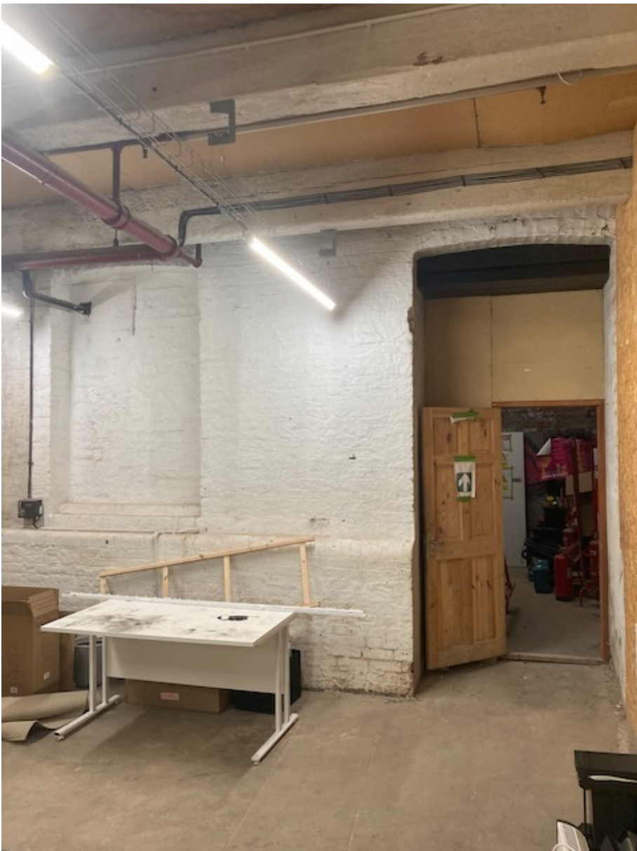
ITEM 02 Brickwork and features to internal face of east gable
