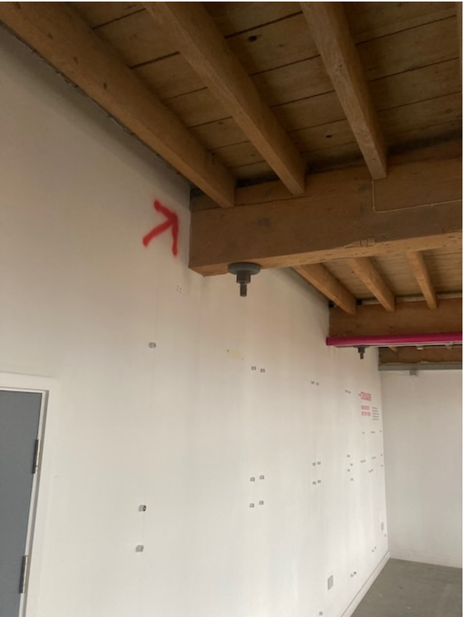
ITEM G2 Exposed primary beam at 3rd floor
