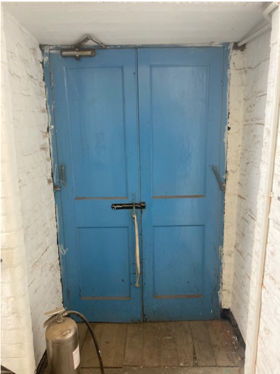
ITEM 22 Brickwork lobby and timber doors to north west stair (stair side)
