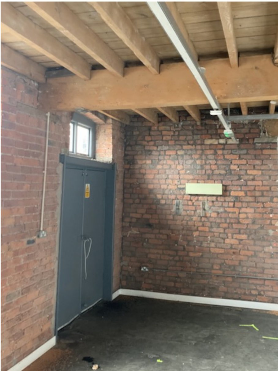
ITEM G6 Sample of cleaned brickwork at 3rd floor
