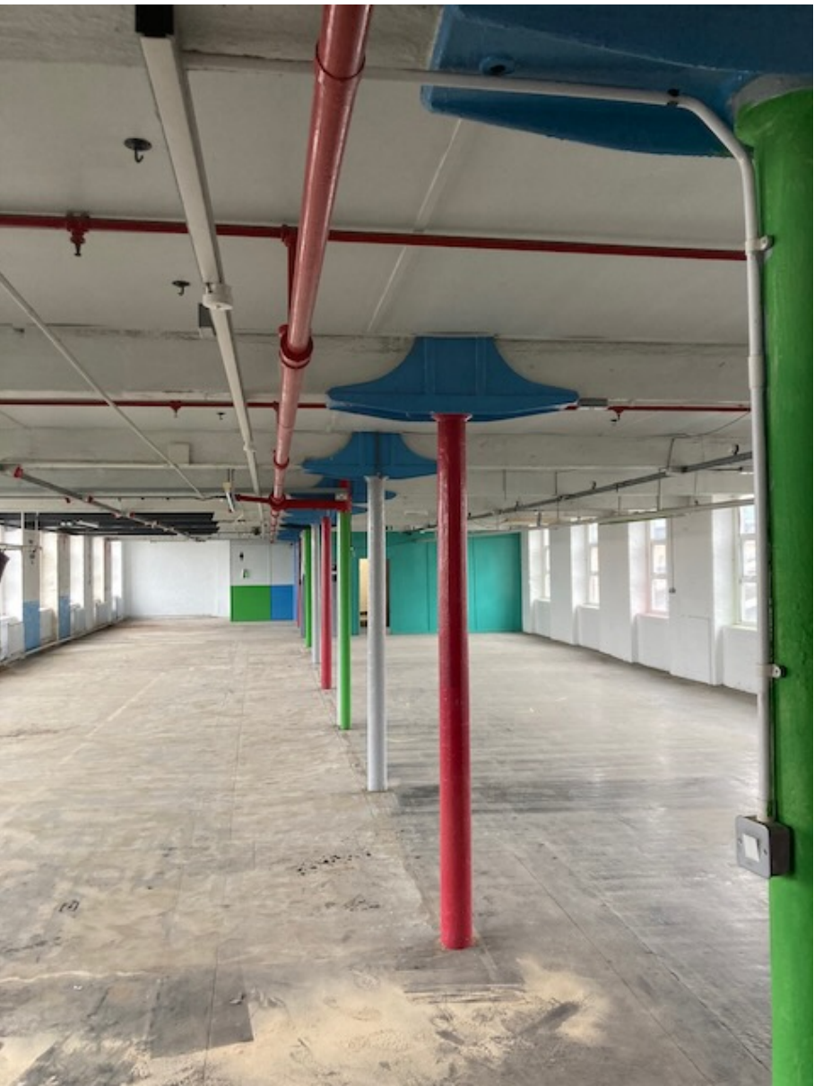
ITEM G1 Typical column and beam shoe at 2nd floor
