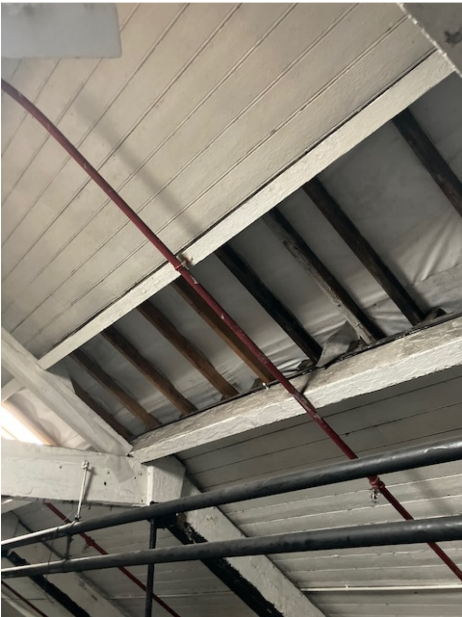
ITEM 42 Purlins to south roof slope with infill to former rooflight opening
