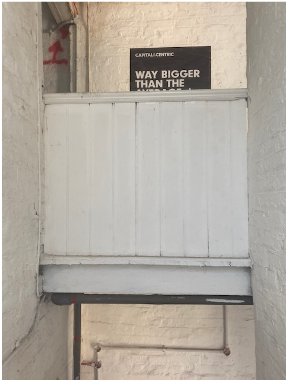
ITEM 47 Timber balustrade panel at head of north east stair
