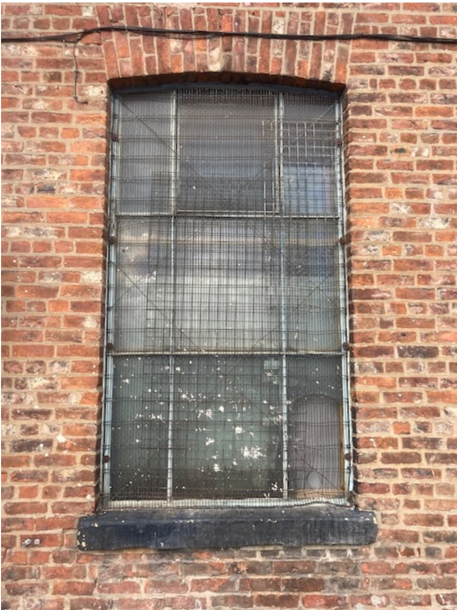
ITEM G13 Typical metal window to Baird Street ground floor
