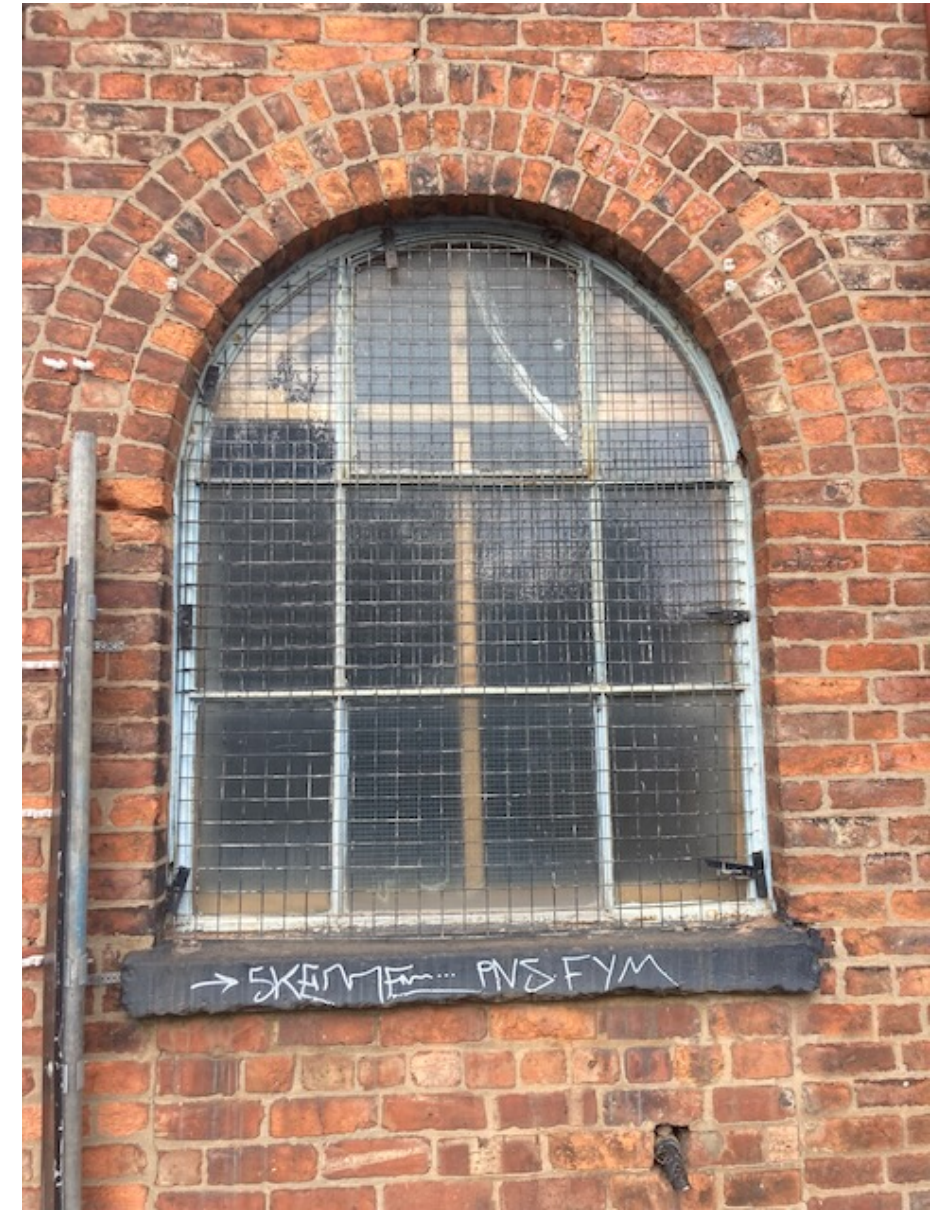
ITEM G13 Metal arched window to Baird Street ground floor
