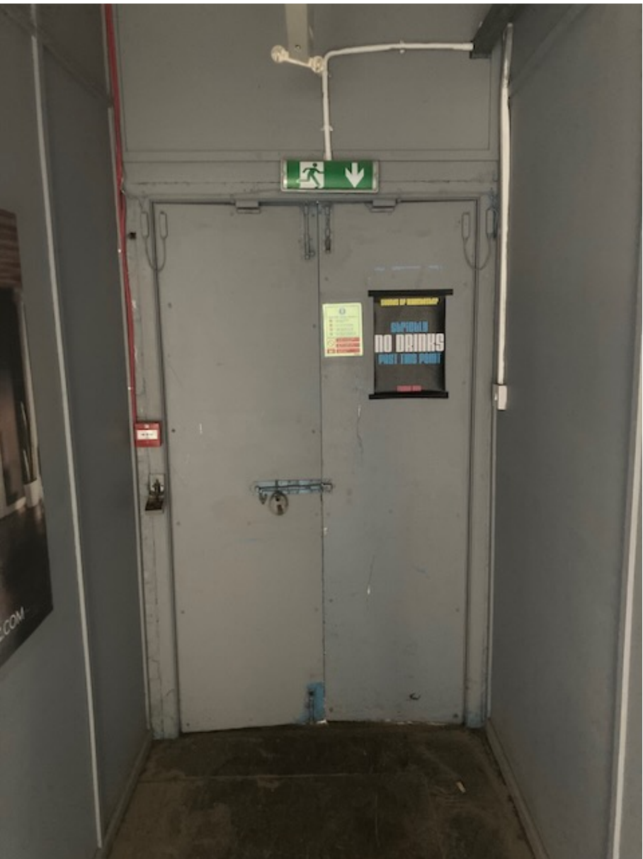
ITEM 22 Brickwork lobby and timber doors to north west stair (office side)
