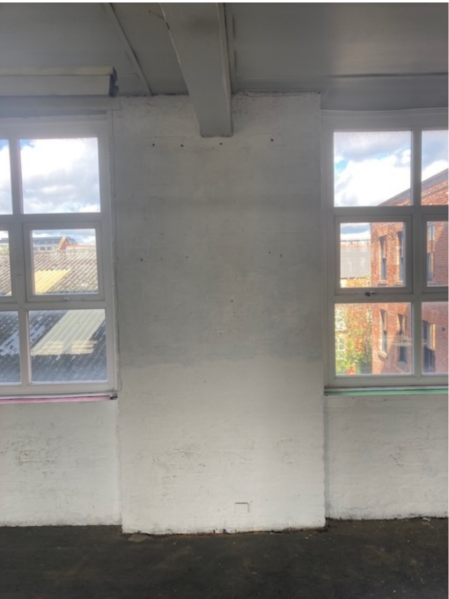
ITEM G6 Typical painted brickwork walls (2nd floor)
