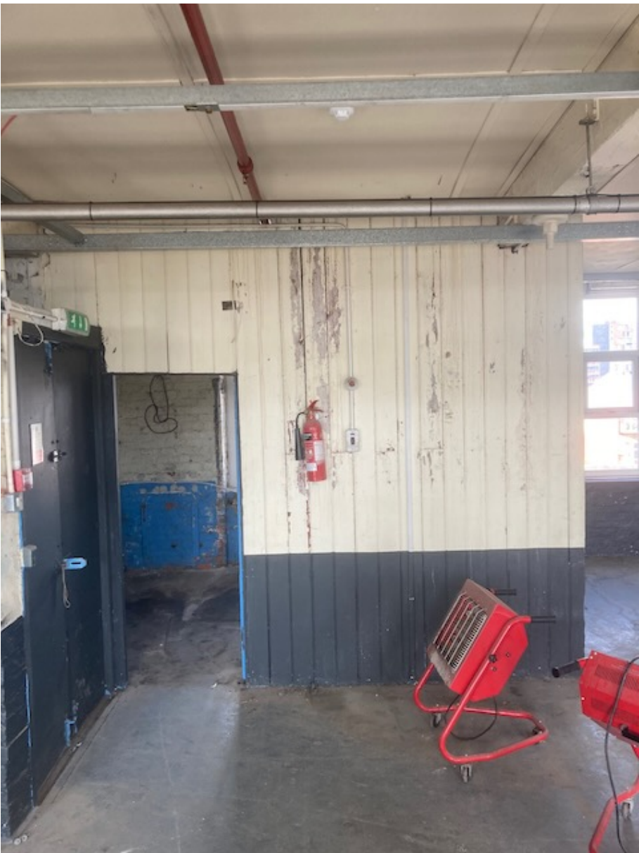
ITEM 33 Timber board partition forming WC area
