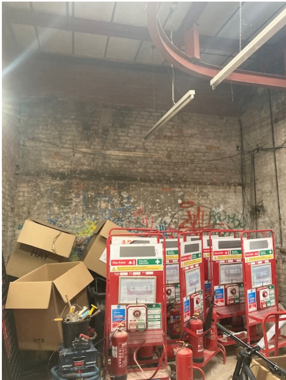
ITEM 01 Internal view of single storey offshoot showing new roof steelwork
