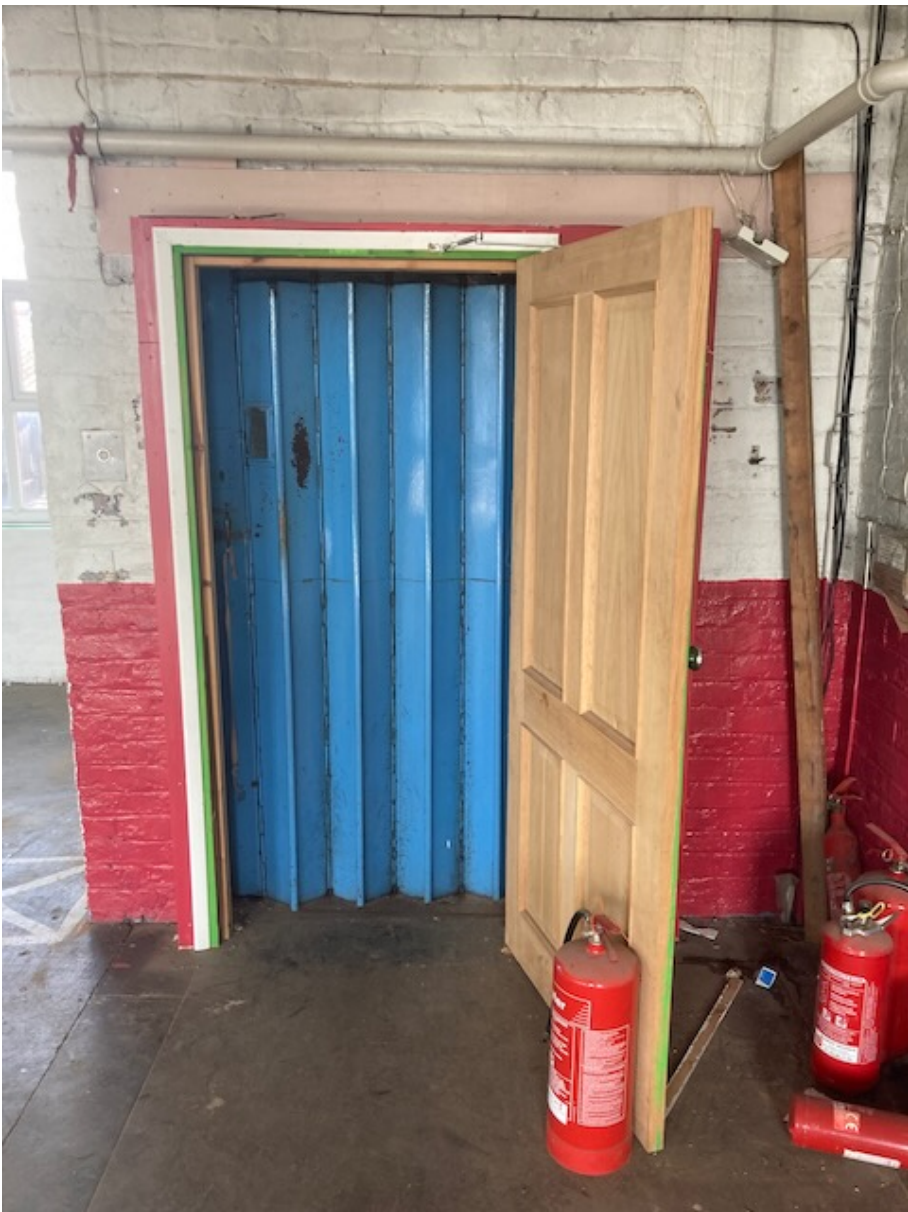
ITEM G7 Internal lift doors at 2nd floor
