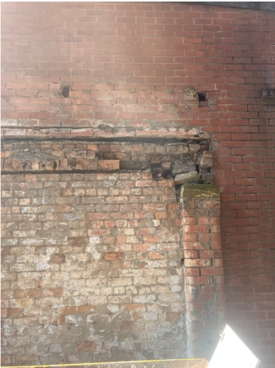
ITEM 01 Detail of brickwork to east elevation of offshoot
