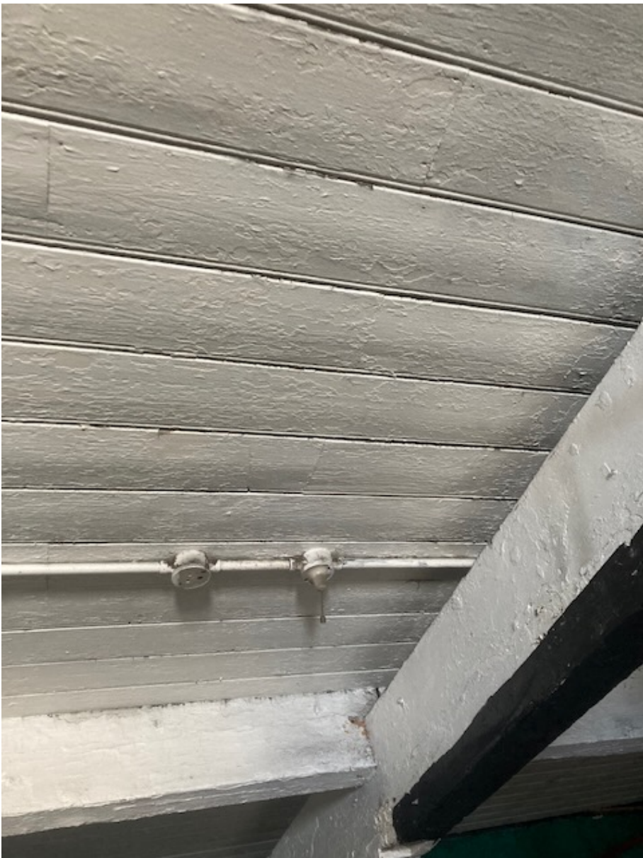
ITEM 44 Timber board lining to underside of rafters
