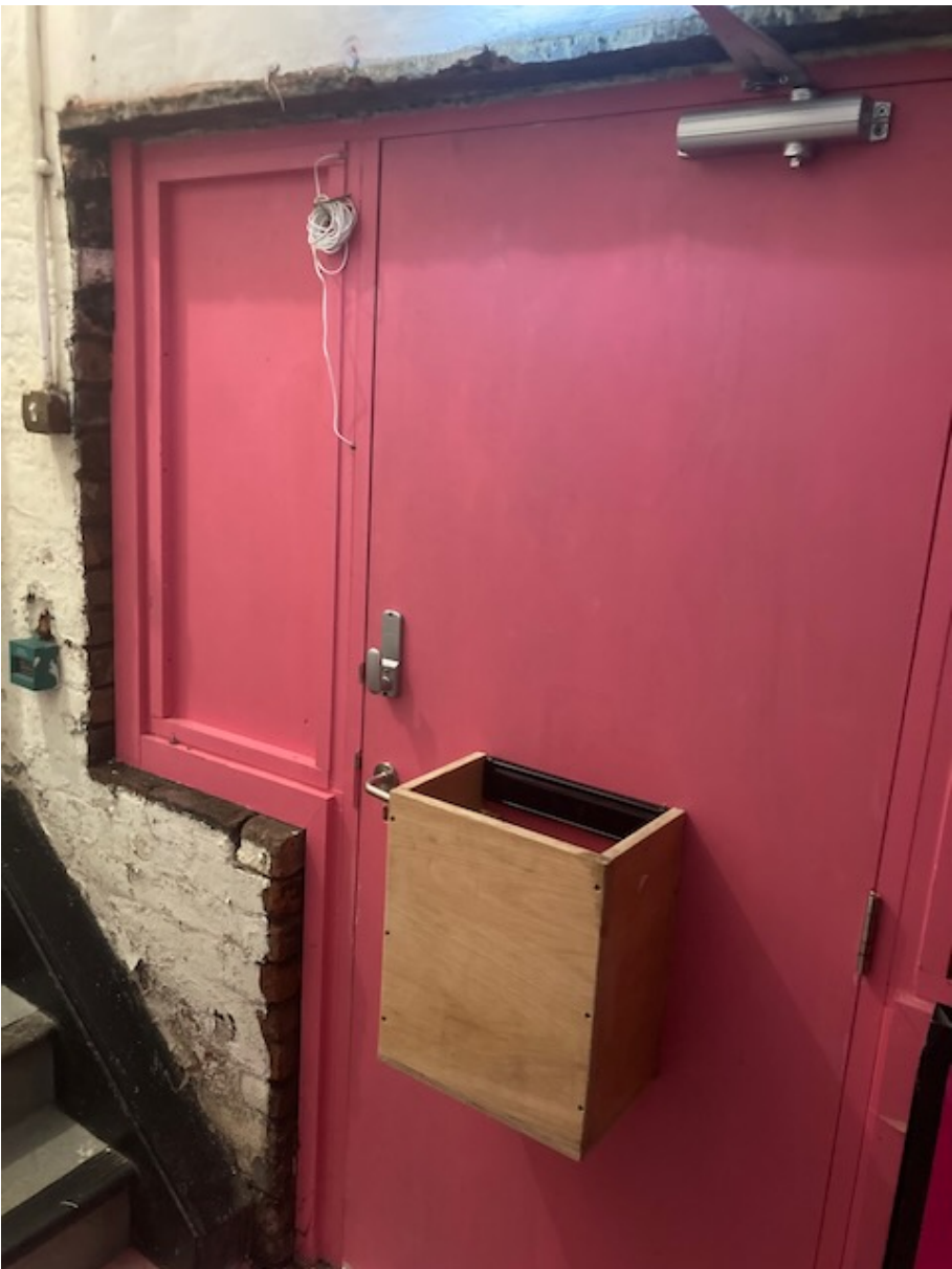
ITEM 03 Entrance opening viewed from inside
