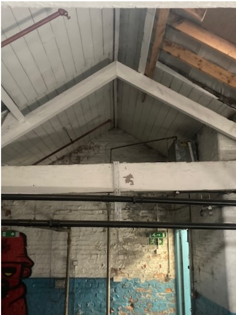
ITEM 41 Typical roof truss upper section with purlins and board ceiling
