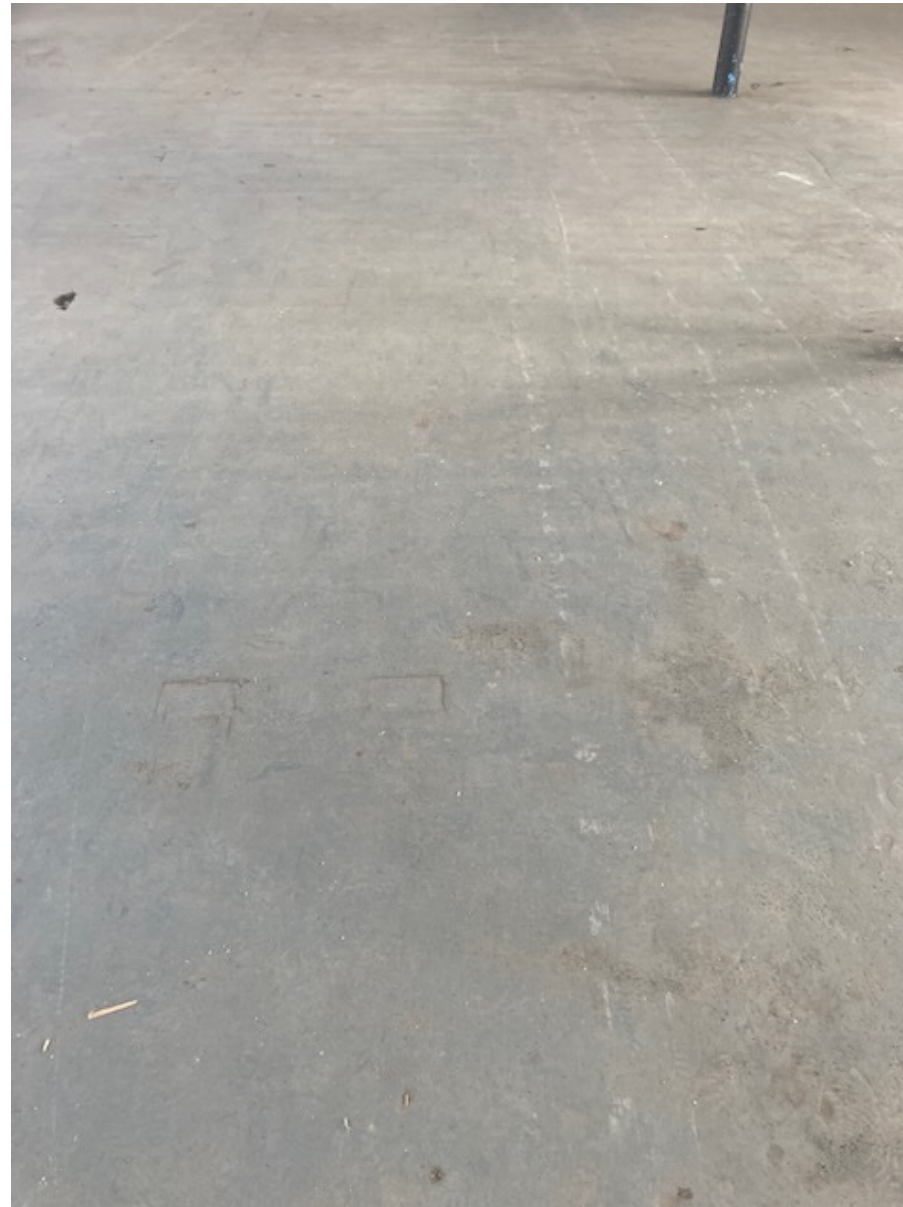
ITEM 13 Asphalt topping to timber boarded floor
