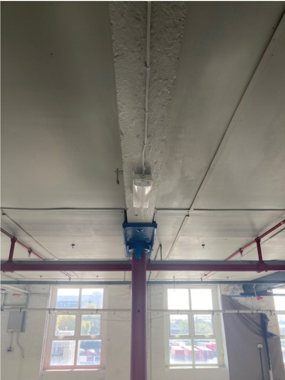
ITEM G2 Typical primary beam at 2nd floor
