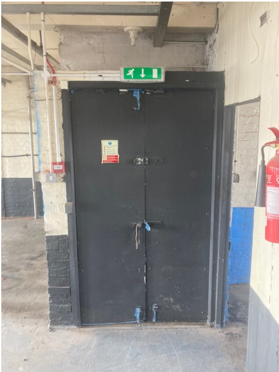
ITEM 32 Brickwork lobby and timber doors to north west stair (office side)
