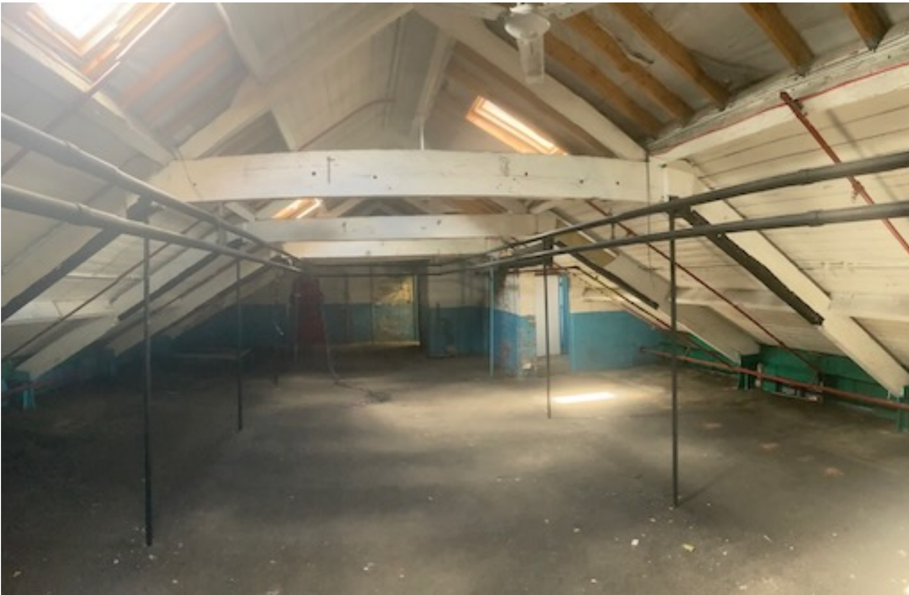
ITEM 41 / 42 Overall roof trusses and purlins with cast iron rods
