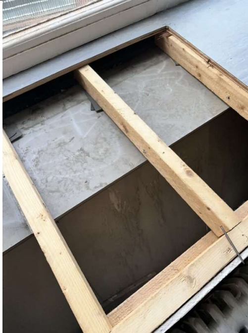
Figure 82- Underlying structure below cotton table (intrusive investigation pictures March 2024)
