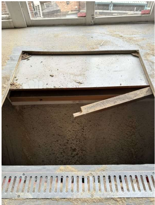
Figure 83- Below the cotton table (intrusive investigation pictures March 2024)
