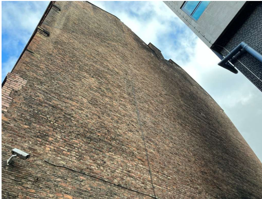
Figure 21- Exposed brick wall at the back of 117-119 Portland Street facing Linley House (Author's own image, 09 January 2024)
