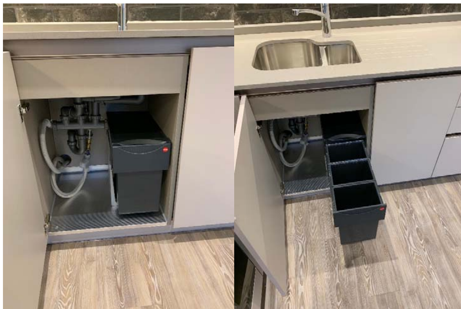
Fig B – photo of installed kitchen bin – with three separate compartments.
