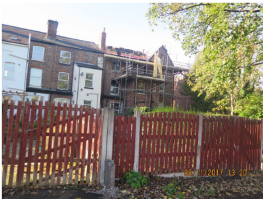
Rear view of property showing more clearly the dominance of the extension to number 97, which has come out further than that of number 95
