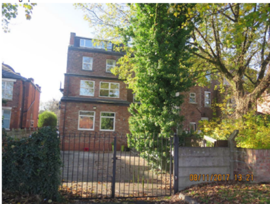
Large ground floor, first floor and dormer extension to number 107
