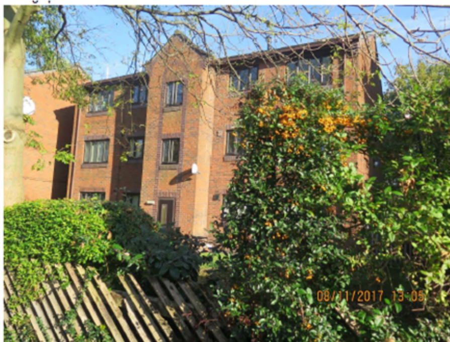
Modern development adjacent to 93 Withington Road
