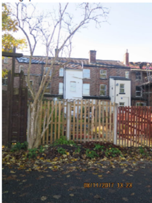
Rear of block showing the white extension of number 97, being an extension from the original building
