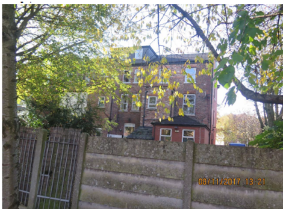
Large single storey extension to number 101 and dormer to 103
