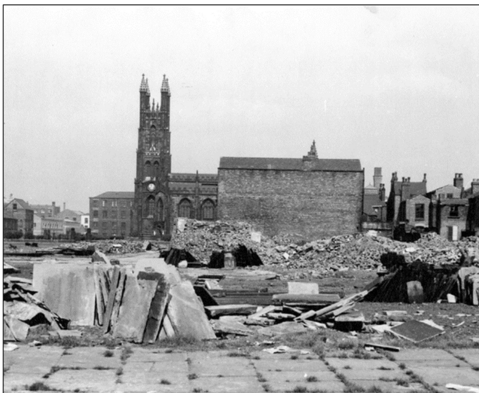
Plate 3: Slum clearance and St George's Church looking north from Silver Street. Site is to the right, 1957 (Source: Manchester Local Image Archive)
