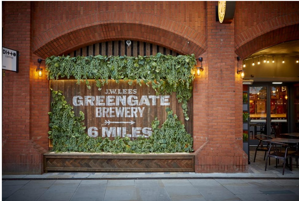
Photograph 1 – As-built external store enclosure wall constructed from reclaimed timber vertical boarding with herringbone upper and lower planters fixed within existing brick arch colonnade. As-built projecting sign visible on right hand column in same location as previously removed sign. As-built external lighting in same location as previous light fittings.
