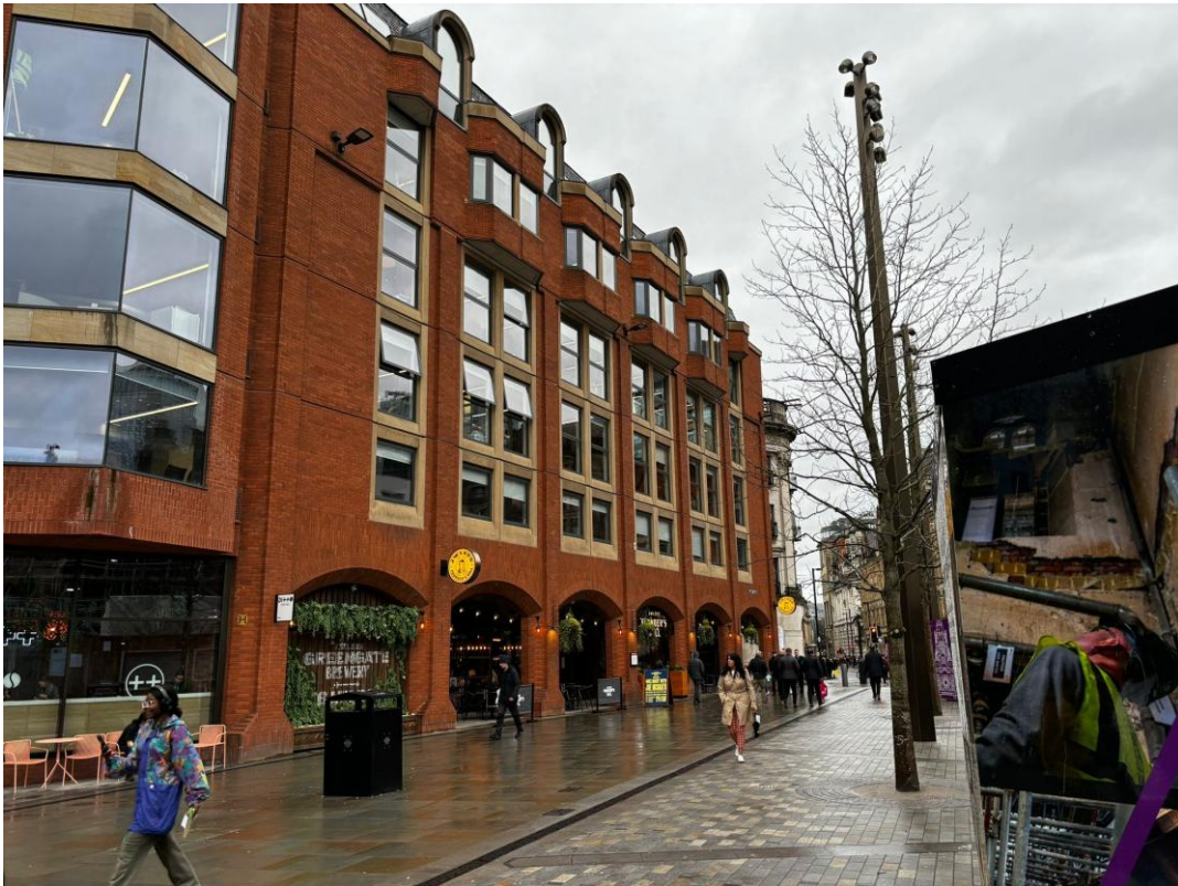
Photograph 3 – As-built external store enclosure wall and 2 nr replacement projecting signs within street scene.
