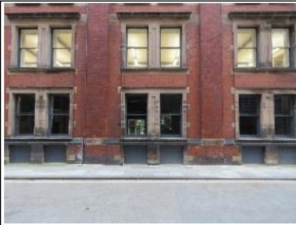
Figure 24: The simple window bays of E Block that maximised natural light gains down to the lower ground floor floor as well.
