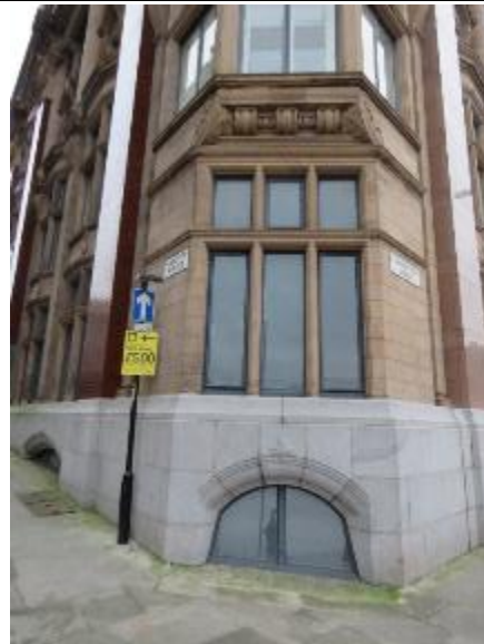
Figure 15: Corner detail of Hanover House with basement window and sandstone mullions and transoms of the steel casement windows.
