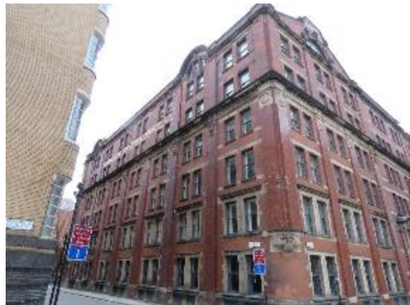
Figure 10: View of E-Block from the corner of Hanover Street and Federation Street showing the simple sandstone and red brick exterior with repetitive timber sash window fenestration.
