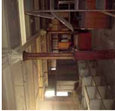
Fig. 6.1.6 and 6.1.7. 2011. Early coloured timber panelling encase the cast-iron columns on the 4th floor. This early display case was found on the sixth floor.
