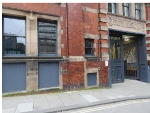
Figure 12: View of ancillary window adjacent to the loading bay that ran the full depth of the building to Balloon Street.
