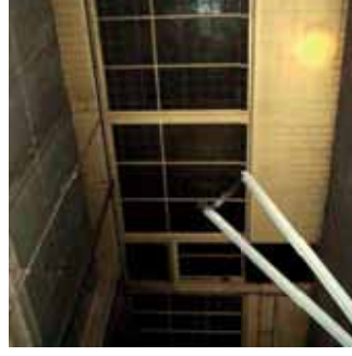
Photo 26 - EB.1F.01- Original glazed partitions
