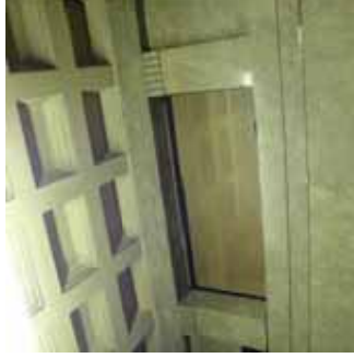
Photo 36. HB.GF.06- Original Ceiling
