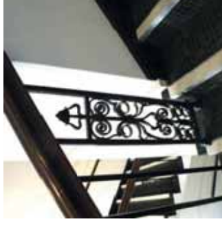
Photo 15. Typical stair detail
