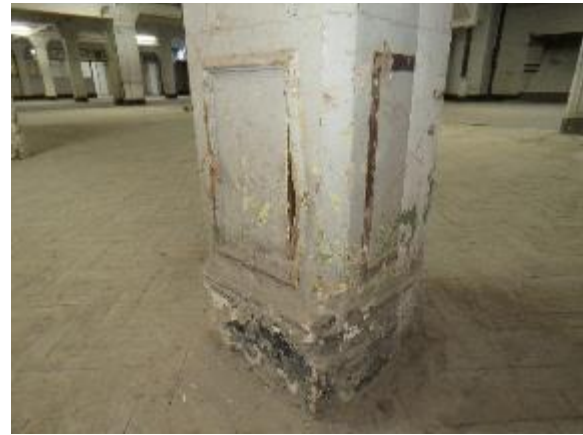
Figure 53: Column base detail with beading to provide panel effect.
