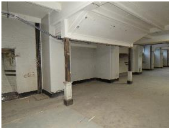
Figure 48: General view of basement windows on Corporation street (southern end of elevation) showing surviving glazed bricks (partially painted) and concrete floor structure.
