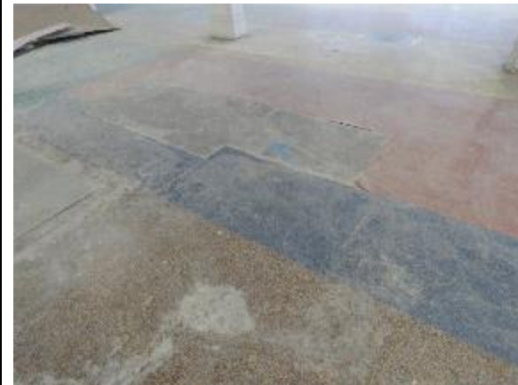
Figure 55: Non-significant floor coverings over earlier timber flooring.
