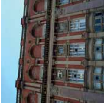
Photo 2. The large majority of windows are original, except for the top range which is a post WWII construction inset in the original arched top floor with roundel windows Balustrated parapet.
