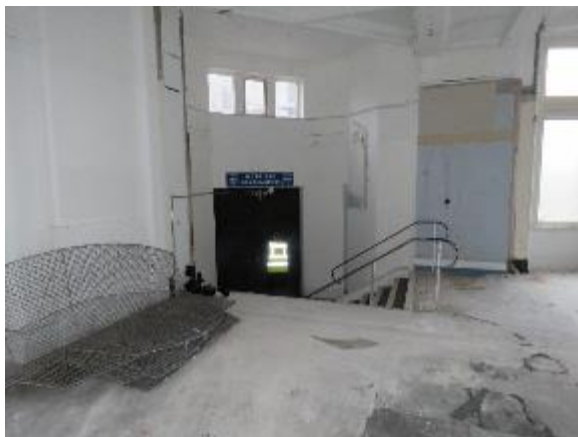
Figure 66: View towards existing corner entrance to Corporation Street and Balloon Street with modern handrail.
