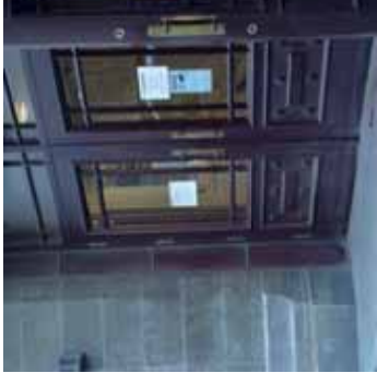
Photo 8. Early entrance doors
