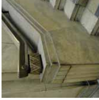
Photo 38. HB.GF.06 - Early stairs finishes
