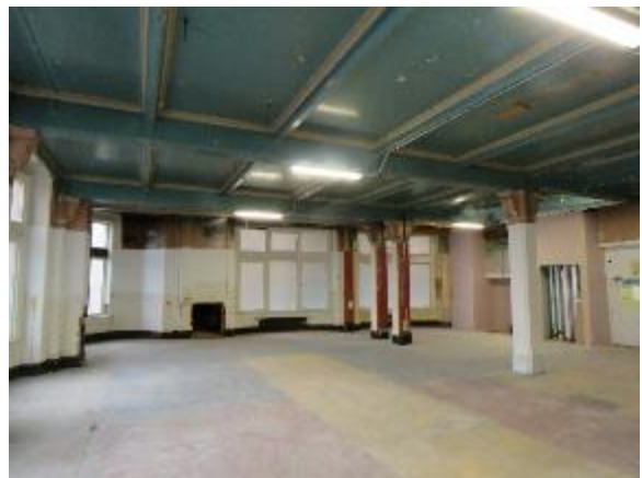
Figure 59: General view looking north through the ground floor space.
