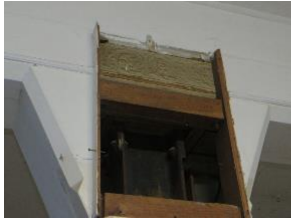
Figure 47: Exposed steel column with early decorative paper unpainted.
