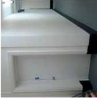
Photo 26. HB.GF.09- Early opening and architrave remains
