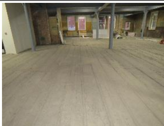
Figure 37: General view of exposed floor structure.
