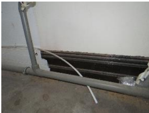
Figure 58: Surviving timber skirting boards, with some areas having been decorated white.
