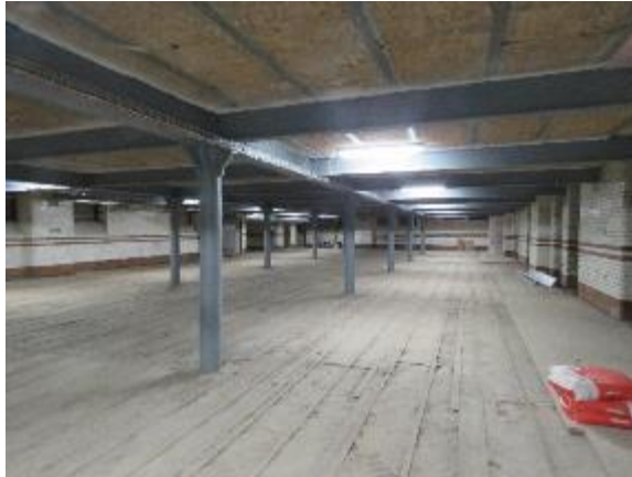
Figure 26: View through lower ground floor from the southern end looking north, with open plan form and floors and ceilings stripped back. Note the extent of glazed bricks to walls.
