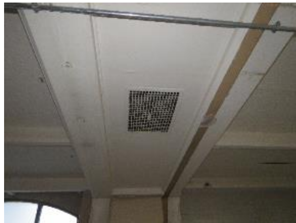
Figure 49: Surviving ventilation grill and ductwork at ceiling level of the original hot air ventilation system.
