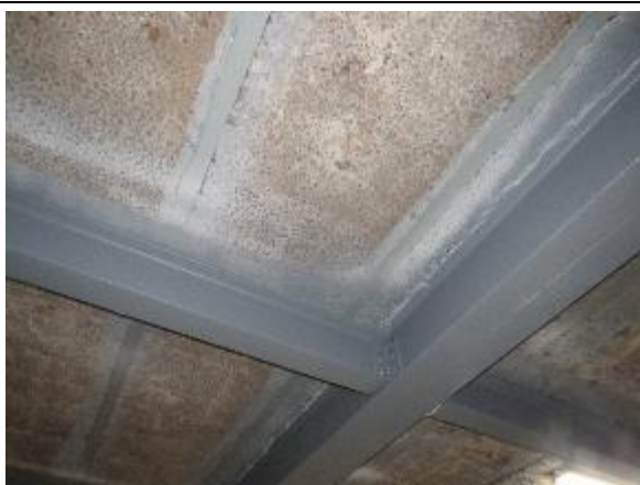
Figure 36: General view of the ceiling showing surviving structural steelwork and floor slab above.
