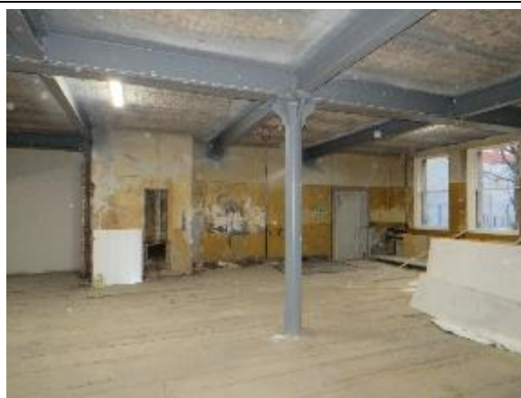
Figure 39: General view of the southern end of the ground floor, showing the column detail (note that there isn't any detail at the column base only at the column head) and ventilation stack with exposed grate.
