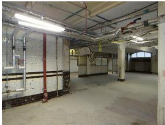
Figure 42: View towards the south west corner of the basement showing the glazed brick and surviving timber and glazed partitions.
