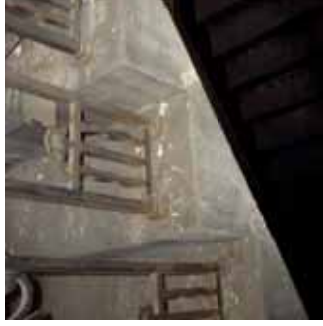
Photo 19 – Typical balustrade and stair detail
