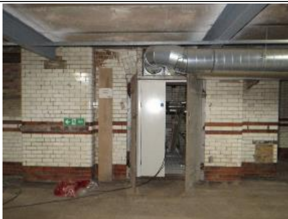
Figure 28: General view of the ceiling showing how the structural columns and beams have been previously painted for fire protection.
