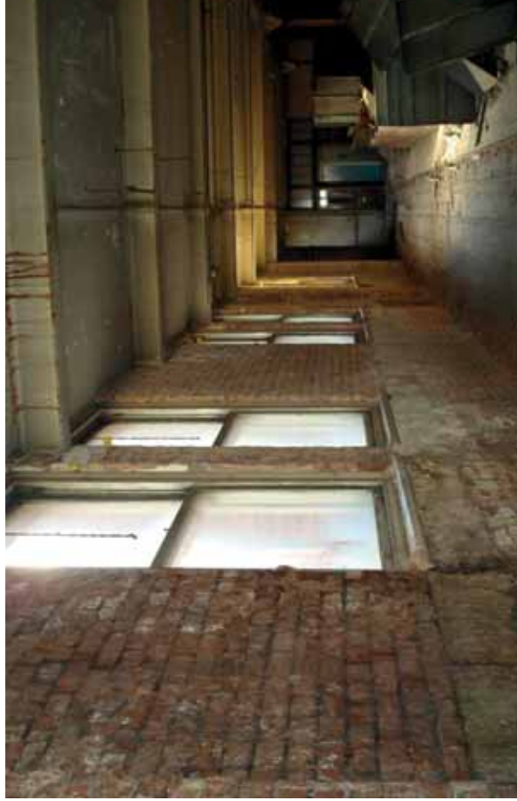
Fig. 6.1.5. 2011. General view of the 4 th floor showing the original ceiling with exposed steel beams. The wall and floor finishes have suffered the effects of water damage.
