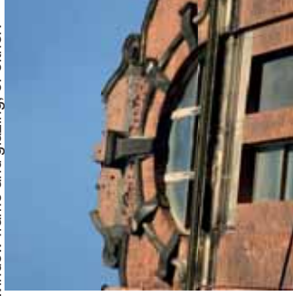
Photo 2 - Original openings (most of which are blocked off at basement and ground floor levels). Some have lost the window frame and glazing, or either.
