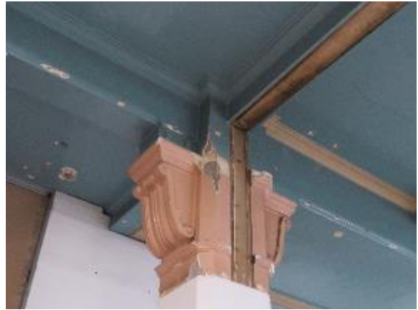
Figure 57: Column head detail with scrolled corbelling.
