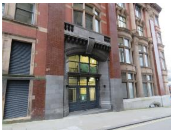
Figure 13: View of the junction between E Block and Hanover House on Hanover Street, with the granite plinth and Hanover Street entrance surround.
