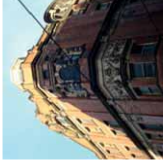
Photo 9 - Original decorative stonework.
