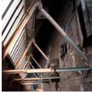
Photo 38 - EB.6F.01 - Original roof
