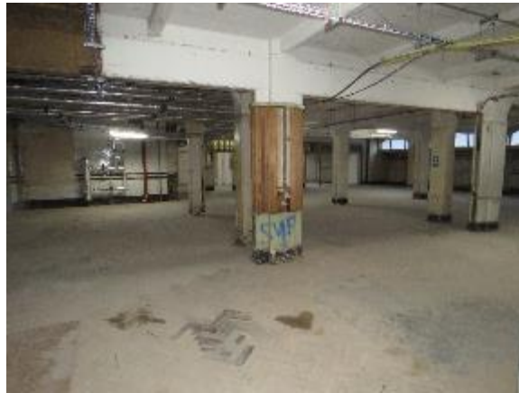
Figure 40: General view of the basement of Hanover House showing the difference in aesthetic as the area was originally used as a canteen.
