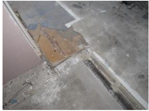
Figure 63: Timber floor coverings with boarding and vinyl over.
