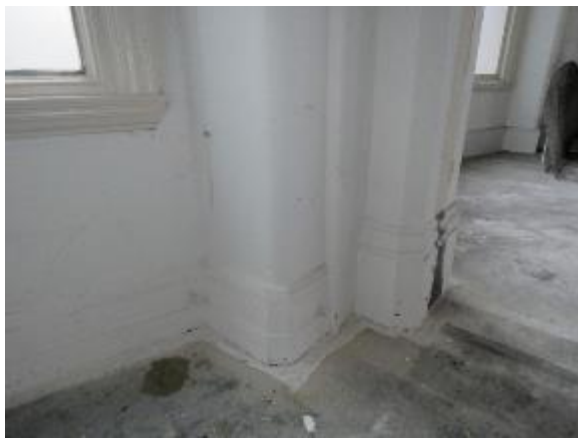
Figure 64: Surviving skirting boards to perimeter of space.
