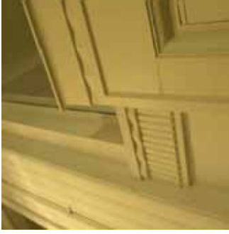
Photo 50. HB.1F.27- Early joinery detail
