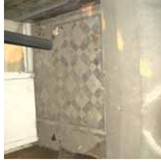
Photo 24 - EB.GF.02- Original tiled flooring
