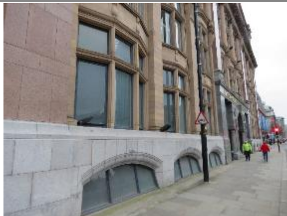
Figure 16: View looking south down Corporation Street along the ground and basement floor of Hanover House with repetitive window bays.
