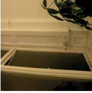
Photo 59. HB.2F.14- Original or early joinery around window, present on parts of the 2 nd floor and also on the 3 rd floor.
