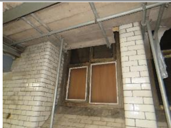
Figure 31: Another lower ground floor window to Balloon St.
