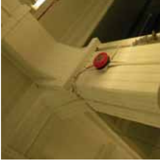
Photo 53. HB.1F.27- Early corridor column detailing
