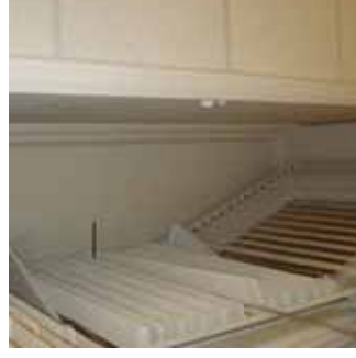
Photo 24. Typical ceiling detail for the ground floor
