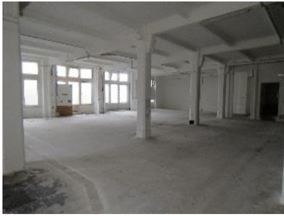
Figure 62: General view of southern area of ground floor.
