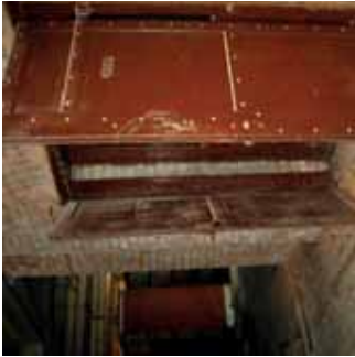
Photo 31 – Typical lift door occurring on all floors
