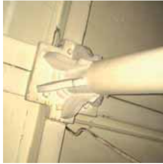
Photo 34 – Typical column head
