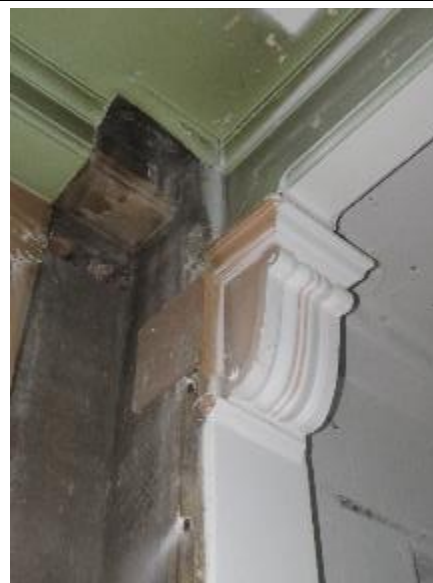
Figure 71: Close up column detail with scrolled corbel detailing and cornice.
