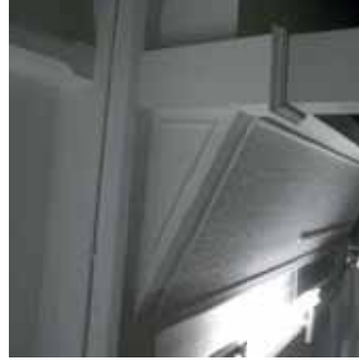
Photo 21. HB.BS.07- Original joinery
