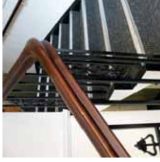
Photo 14. Typical stair handrail
