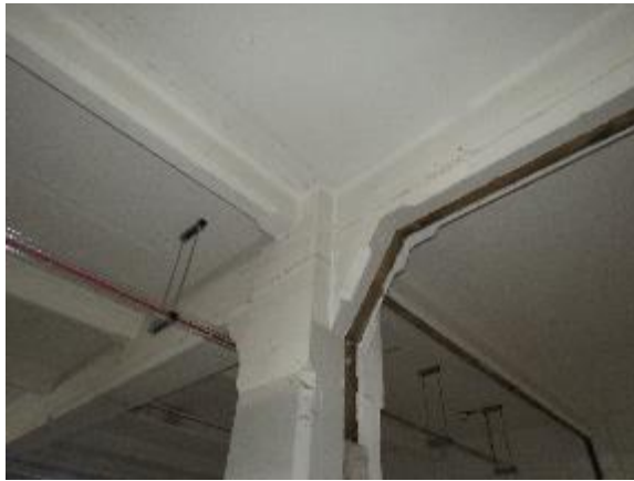
Figure 52: Column head detail with primary and secondary beams of the floor structure.
