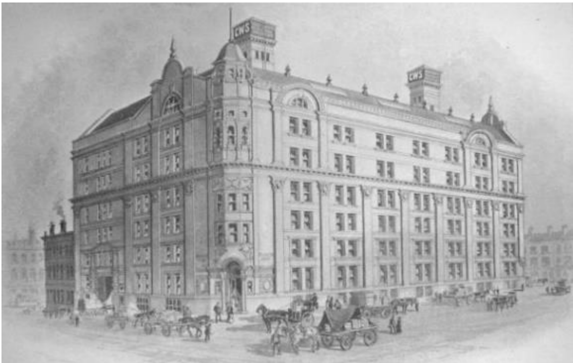
Figure 8: View of the corner of Balloon and Federation Street. The New Drapery Building (E-Block) towers over the streetscape and the much smaller building fronting onto Corporation Street. The overpowering scale of the new warehouse overlays the historic street grain, heralding the changes to be brought forth in the area. (Source: CWS Annual 1904).
