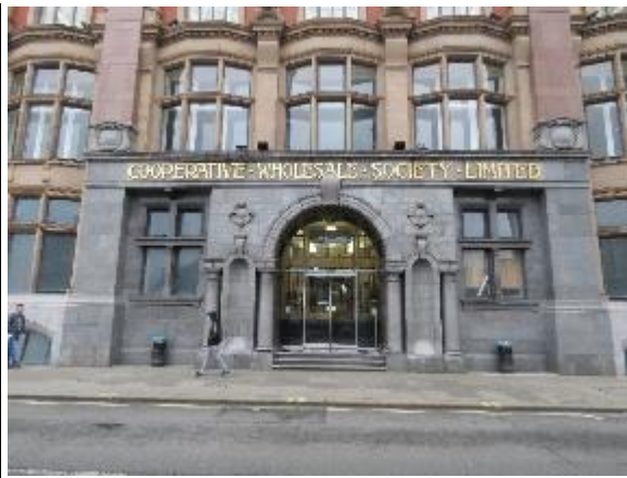
Figure 18: View of the primary Corporation Street entrance to the building.
