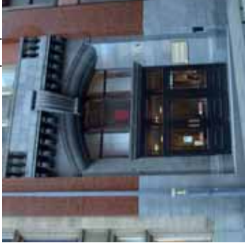
Photo 2. The large majority of windows are original, except for the top range which is a post WWII construction inset in the original arched top floor with roundel windows Balustrated parapet.
