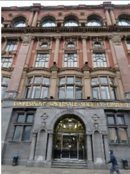
Figure 20: View of the primary central section of the Corporation Street Façade.
