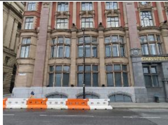
Figure 17: Northern section of the Corporation Street façade of Hanover House, illustrating repetition in the façade fenestration.
