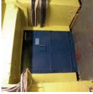
Photo 18. HB.BS.01- Original doors linking to old bank
