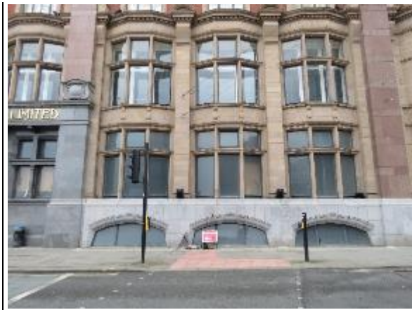
Figure 19: Southern section of the Corporation Street Façade, again illustrating repetition in facades design.
