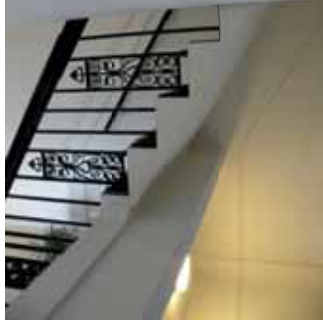
Photo 13. Typical stair balustrade
