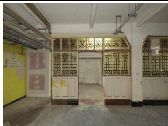
Figure 43: An area of the timber parquet floor which has been lifted
