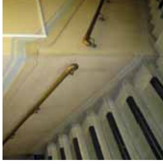
Photo 40. HB.GF.22- Early handrail and finishes on central stair core
