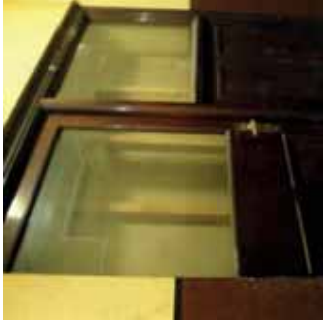
Photo 33. HB.GF.08 - Early door and joinery
