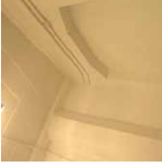
Photo 56. HB.2F.13- ca. 1930's moulded ceiling and arched wall.
