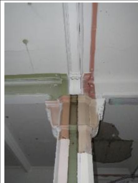
Figure 70: Close up column detail with scrolled corbel detailing.
