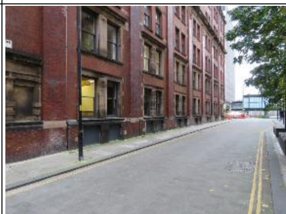
Figure 23: View looking north down Federation Street showing the repetition in E Block's design.
