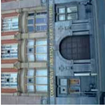
Photo 5. Impressive round-headed central doorway, flanking niches and side windows set in black polished granite surround with frieze & lettering
