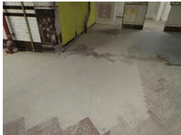
Figure 43: An area of the timber parquet floor which has been lifted
