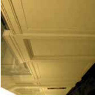
Photo 49. HB.1F.27- Early door opening blocked and early partitions
