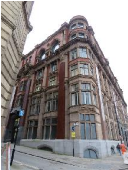
Figure 14: The chamfered corner of Hanover House between Hanover Street and Corporation Street, not the substantial increased use of sandstone between E Block and Hanover House.
