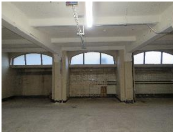
Figure 48: General view of basement windows on Corporation street (southern end of elevation) showing surviving glazed bricks (partially painted) and concrete floor structure.
