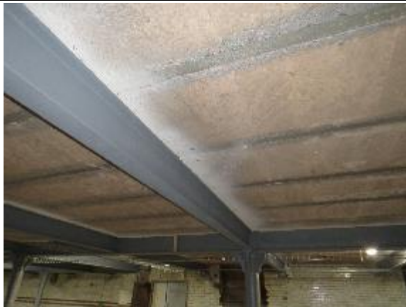
Figure 28: General view of the ceiling showing how the structural columns and beams have been previously painted for fire protection.
