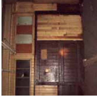
Photo 21 - EB.GF.07- Thought to be original or early partitions
