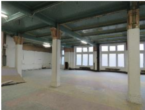
Figure 54: General view of northern area of the ground floor showing current condition of space.
