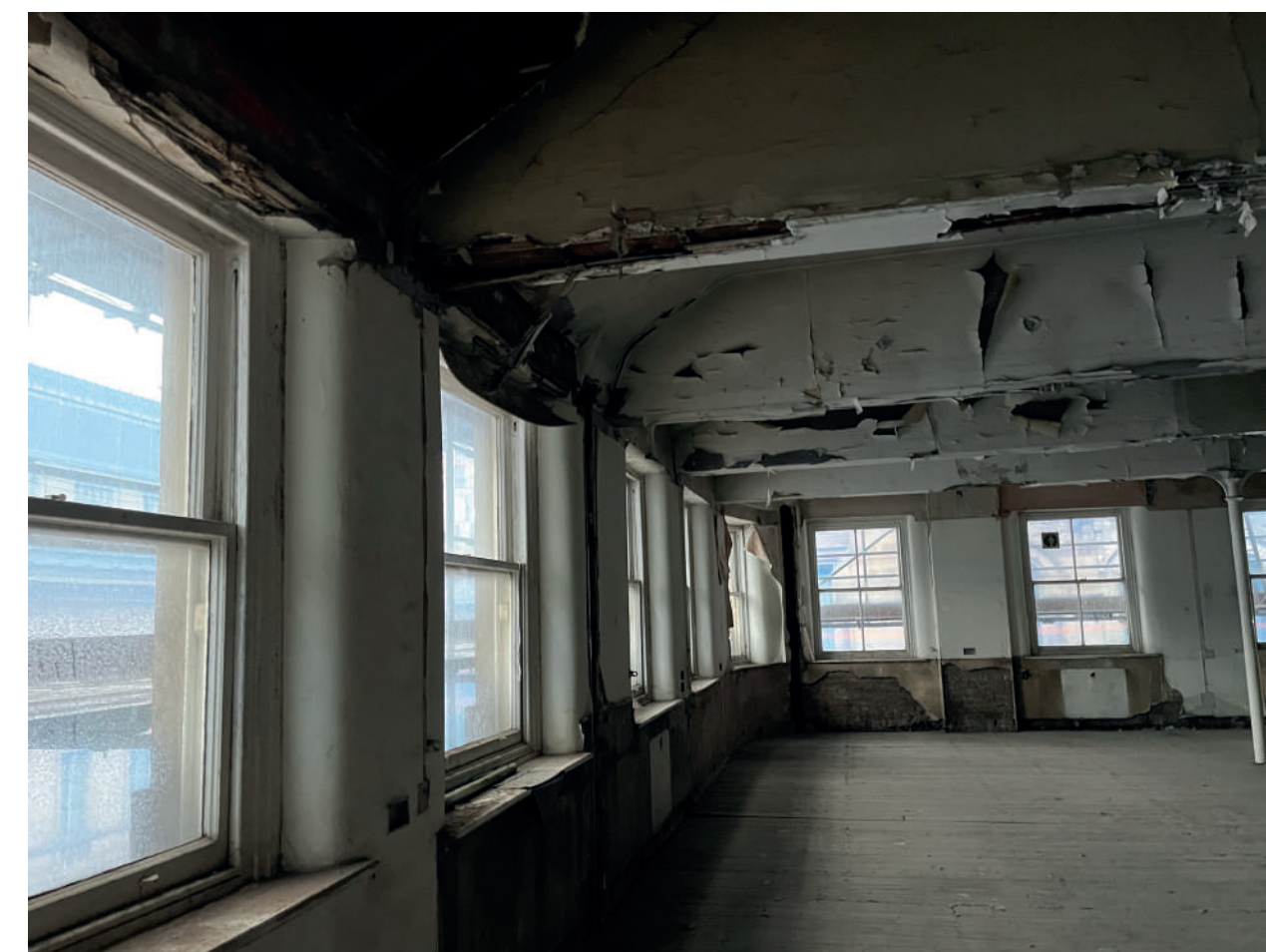
Typical ceiling profile- sloped eaves, and flat ceiling between beams generally.
