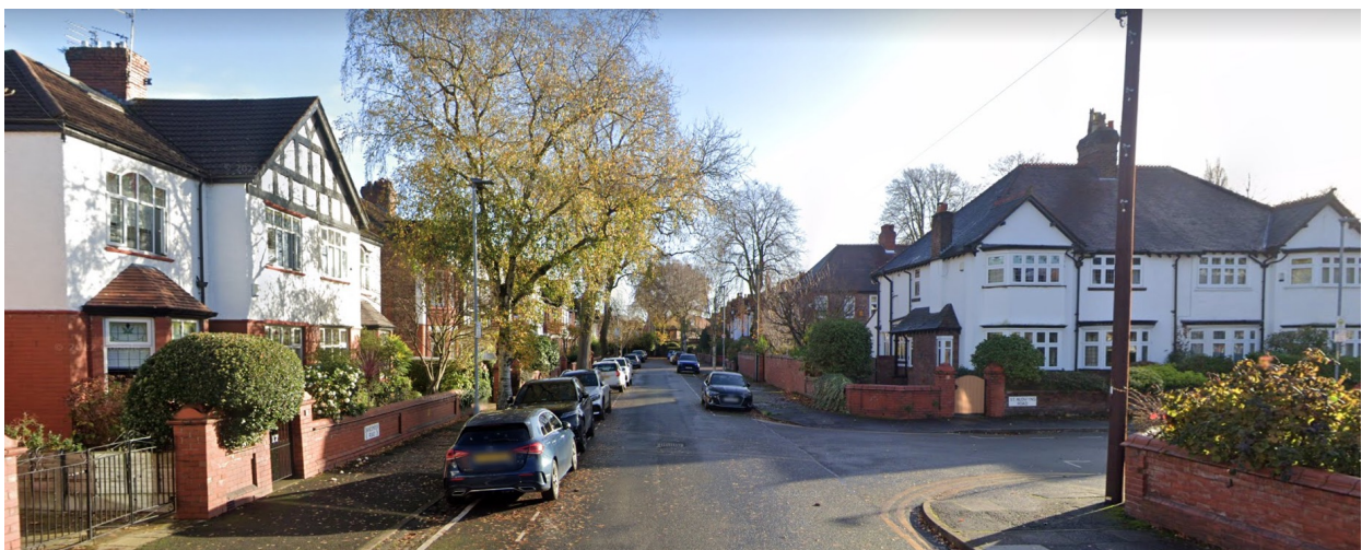
• View looking east along Danesmoor Road
