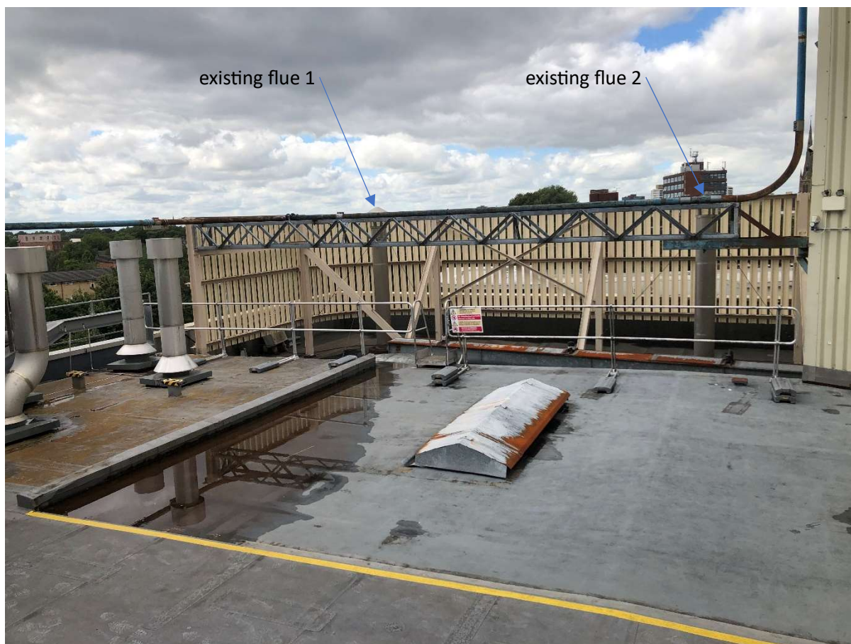
Photograph of the existing flues from the adjacent roof showing the existing screening which will be retained.
