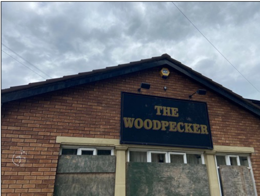
Photograph 4; A view of the front facing gable of the building. The newer brickwork again indicates this section has been more recently added. This section is in very good condition.
