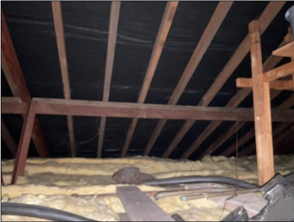
Photograph 7; Another view of the internal loft space. Wooden purlins and rafters support the roof, with some steel support beams also noted. The external roof features a felt membrane beneath; this membrane is in very good condition.
