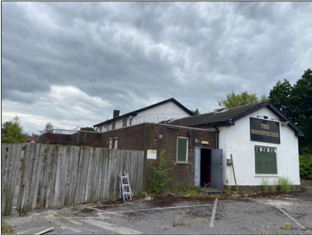
Photograph 1; A view of the subject building on site. Note the single-storey pitched roof section adjacent to a concrete flat topped roof section. Whitewash walls and wooden fascia linings feature across the building.
