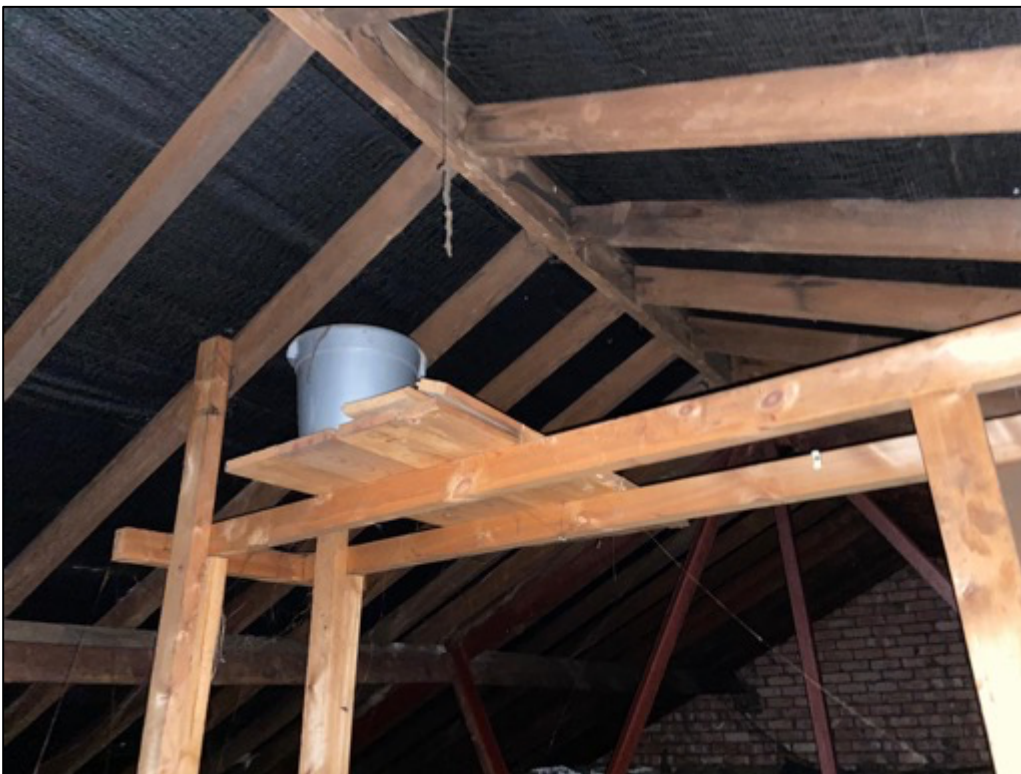
Photograph 8; Internal walls are in good condition also, with no displacement exposing cavities and sealed to intersecting purlins and rafters.
