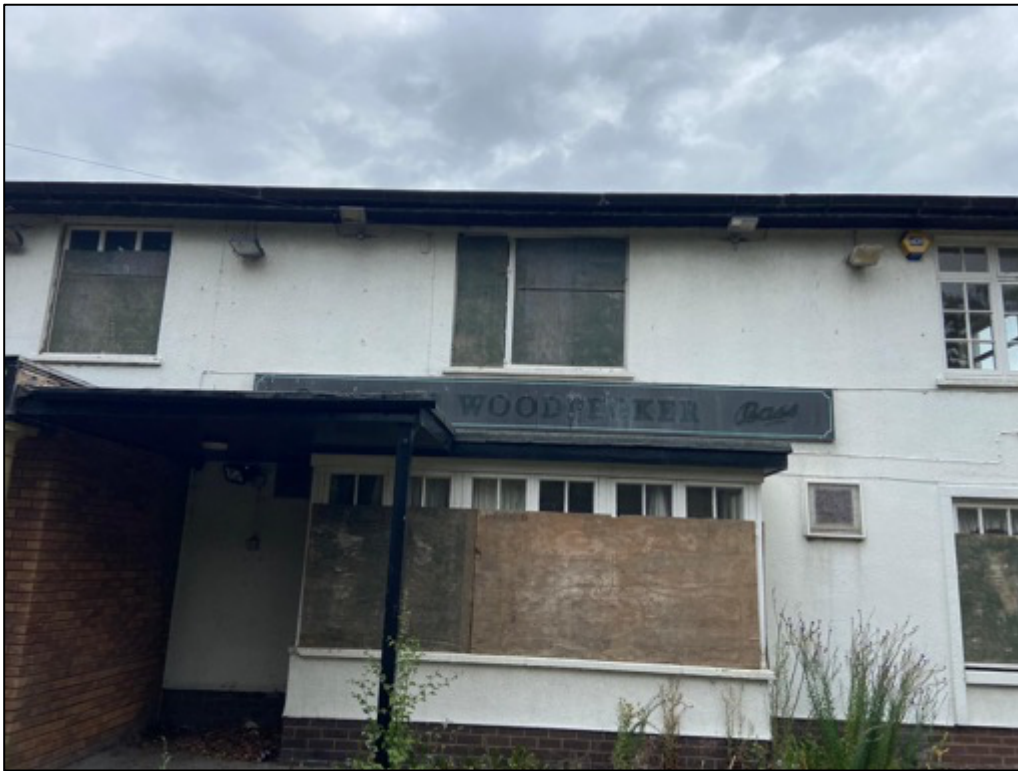
Photograph 5; The wooden soffit and fascia linings are in good condition across all faces of the building.
