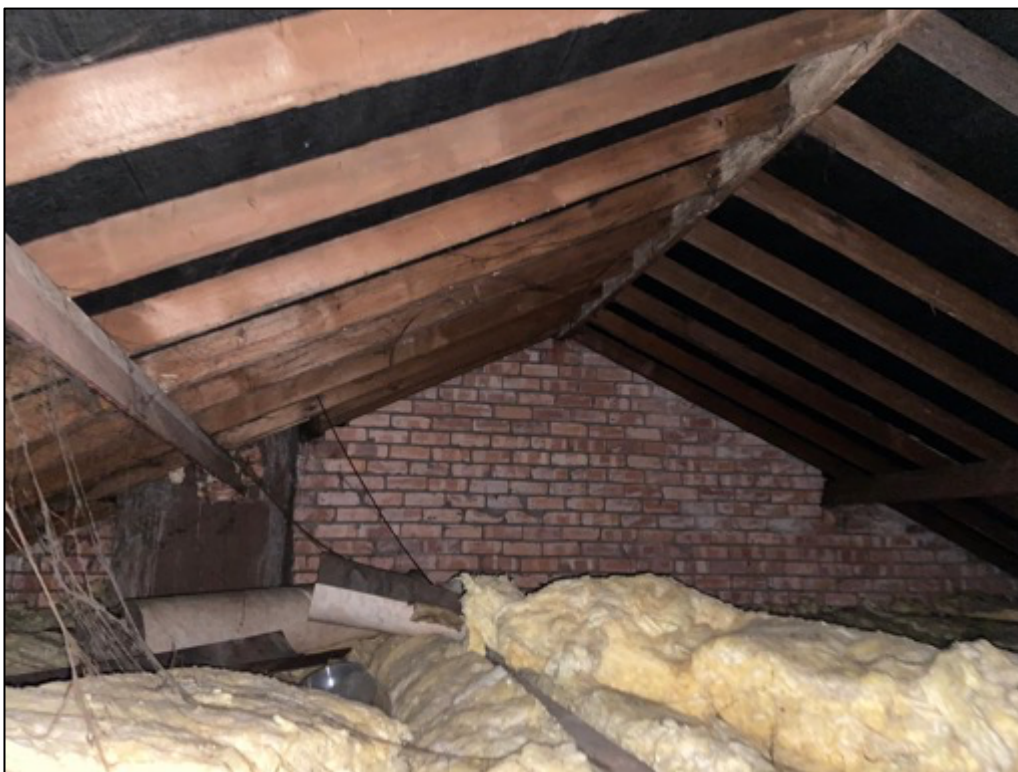
Photograph 6; An internal view of the building loft space. Standard insulation material is scattered across the loft floor, with no signs of previous bat usage or bird nesting noted during the survey.
