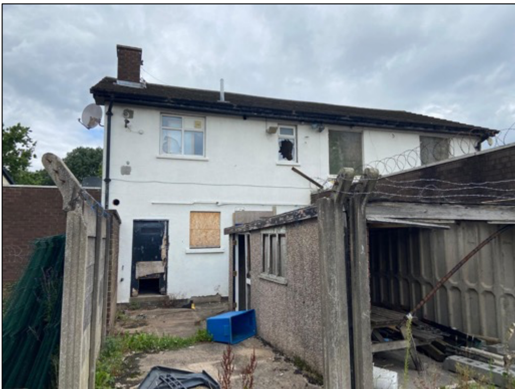
Photograph 2; A view of the rear of the subject building. Boarding and reinforcement has been added to most windows and external walls. Some upper windows are smashed. The roof can be seen in good condition, with no instances of tile displacement or damage.
